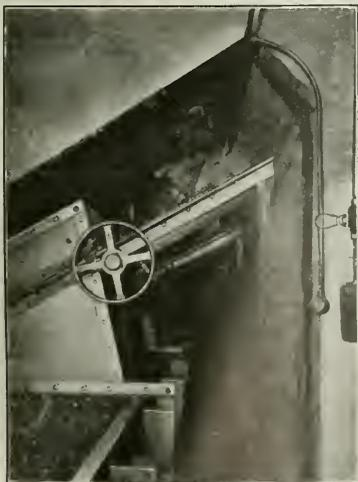
RECLAIMING CONVEYOR IN TUNNEL BENEATH STORAGE
