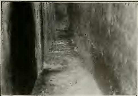
FIG. 1. VIEW OF WATER RING WITH WATER FALLING FROM TERRA-COTTA PIPES ABOVE
