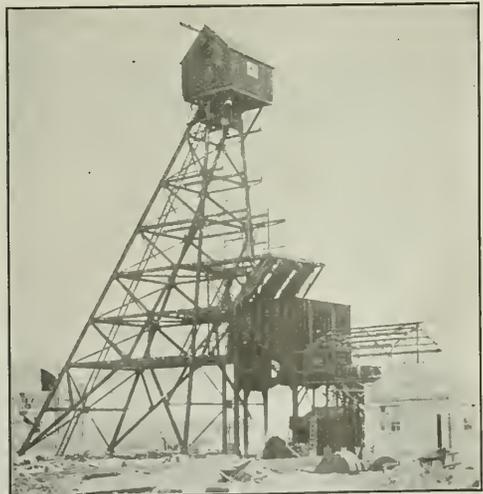
CLOSE-UP VIEW OF MAIN-SHAFT HEADFRAME, TIPPLE AND CRUSHER HOUSE
