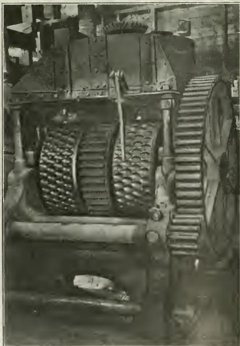
FIG. 1. PRESS FOR MAKING 4-OZ. EGGET BRIQUETS
