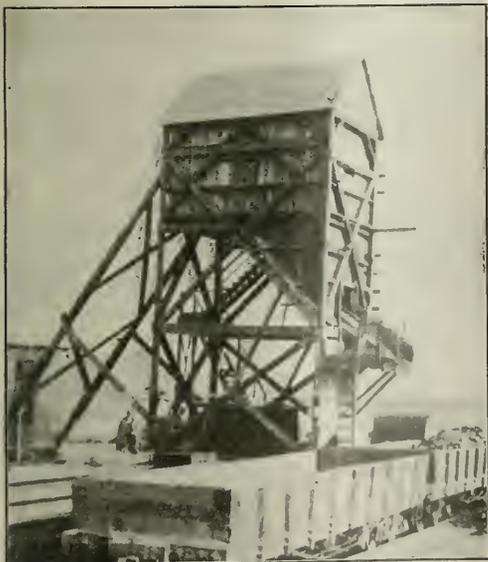
TIPPLE USED IN SINKING SHAFT
