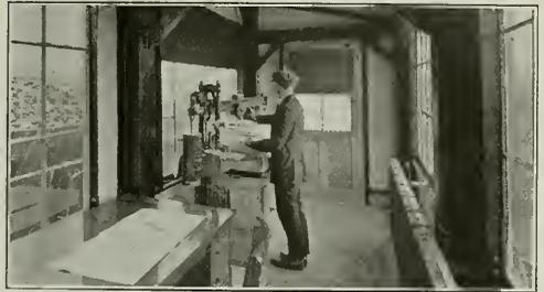
WEIGHMASTER PUNCHING TICKET ON SELF-REGISTERING SCALE BEAM
