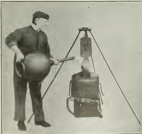
FIG. 1. CHARGING THE AEROPHOR WITH LIQUID AIR. The liquid air is being poured out of a Dewar flask, a sort of magnified "vacuum bottle," into the breathing apparatus which is hanging from a spring balance. By the dial on this scale the weight of liquid air received can be determined.
