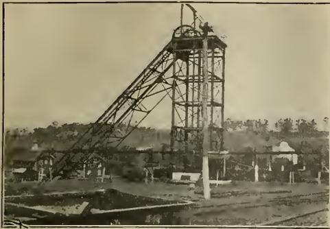
PEACH ORCHARD HEADFRAME OF GLEN ALDEN COAL CO. Separate empty storage tracks feed separate compartments of the shaft and each compartment receives its loaded cars at the foot of the shaft from a separate storage track. Thus the car stops can be placed near the cages.
