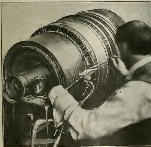
FIG. 3. SOLDERING A COMMUTATOR WITH RISERS
