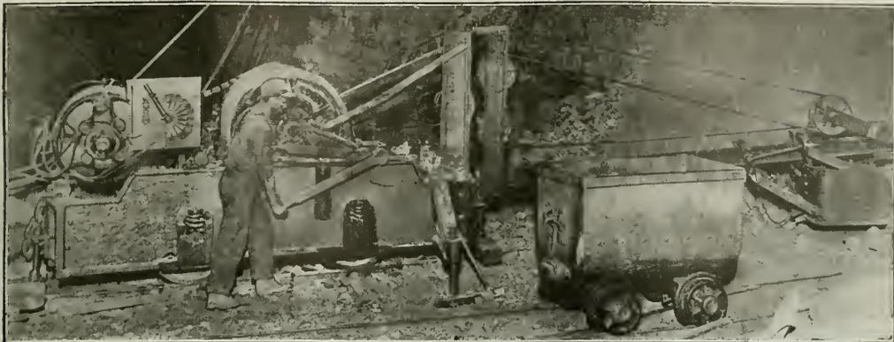
CONWEIGH SHOVEL LOADER, IN WHICH THE DIPPER SLIDES BACK AND FORTH ALONG A BOOM
