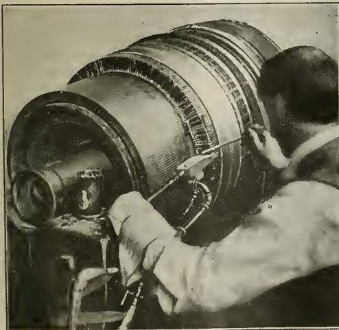
FIG. 3. SOLDERING A COMMUTATOR WITH RISERS
