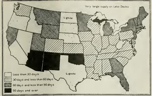
**FIG. 3. DAYS' SUPPLY OF SOFT COAL ON HAND AT INDUSTRIAL PLANTS ON MARCH 1, 1922**
