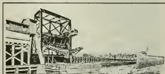
DUMPING THE COAL FROM CARS INTO BOATS, 8.5c. PER TON
