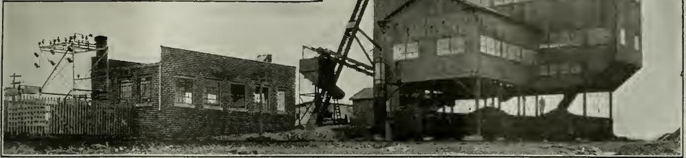
Coal Fed to Picking Table Car by Car, Lumps Being Delivered Above Slack—By Single-Roll Crusher Coal Can Be Delivered as All Egg and Slack or as Slack Only
