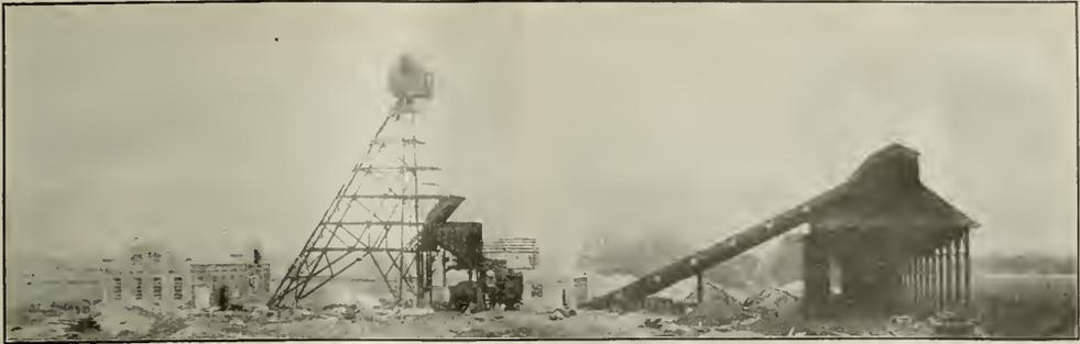
HOIST HOUSE, HEADFRAME OF MAIN HOISTING SHAFT, TIPPLE, CRUSHER HOUSE, CONVEYOR SHED AND LOADING BINS\*
