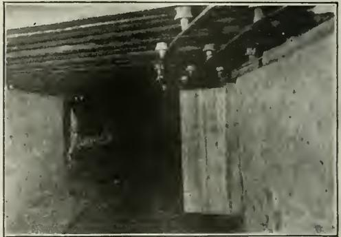
A CONCRETE OVERCAST WITH AN EXPLOSION DOOR
