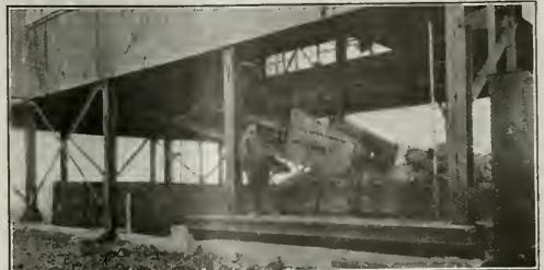
FIG. 1. LOADING BOOM ADJUSTED BY ELECTRIC HOIST
