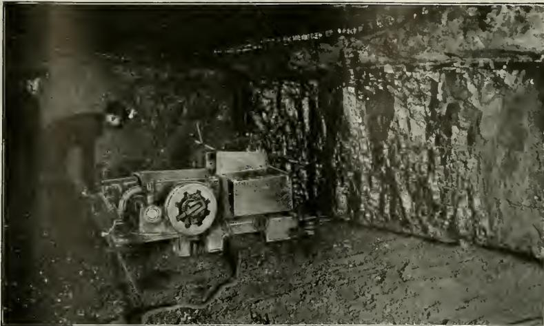
the right-hand rope is wound up in sumping, it is ready for use as a tail-rope on the running cut. On the completion of the cut across the face an ample length of this rope is unwound for the reloading operation. When the machine has been loaded the right-hand rope is completely wound upon its drum; the left-hand rope is almost completely wound up at the completion of the face cut.
