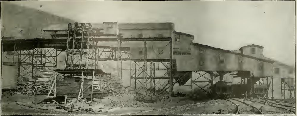
TIPPLE AT PARKERS RUN MINE; ELEVATORS ON SIDE USED FOR RAISING PIT PROPS TO TIPPLE HEIGHT
