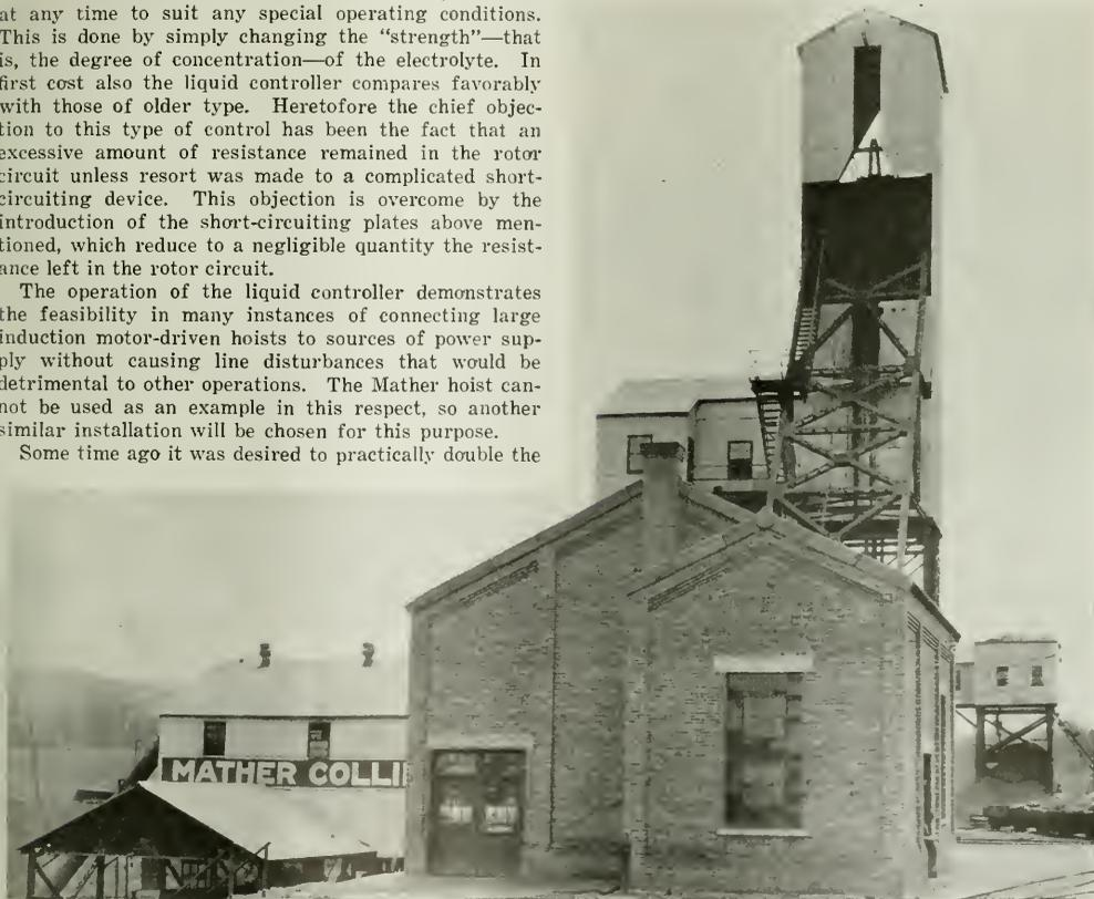
REAR VIEW OF MATHER COLLIERIES HOIST HOUSE WITH TIPPLE IN BACKGROUND. This plant has a capacity of 3,000 tons per eight-hour day. The mine is laid out for a production of 6,000 tons, which tonnage would require, however, a duplication of the present tippel and hoisting equipment. The wing of the hoist house, containing the liquid controller, the primary oil switches and two magnetically operated reversing switches, may be seen in the foreground.
