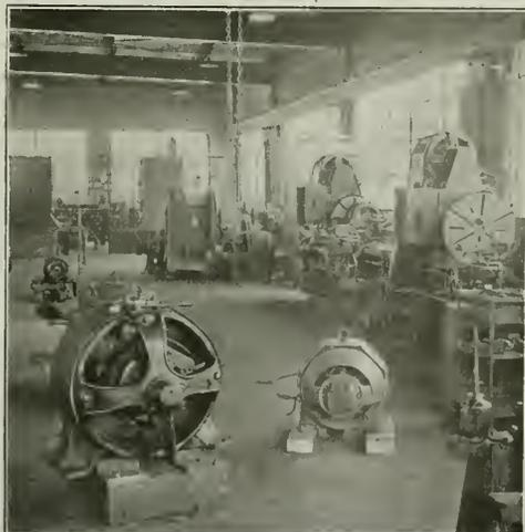
FIG. 6. WHERE MOTORS ARE TORN DOWN AND ASSEMBLED
