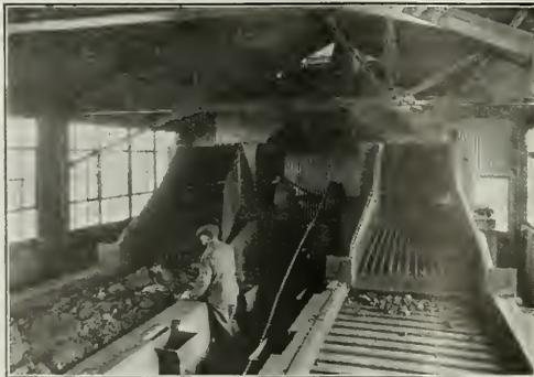
FIG. 3. PICKING TABLES; LUMP COAL ON TOP
