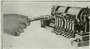
TESTING CONTACTOR PRESSURE
