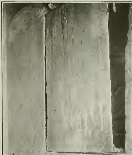
CONCRETE SHAFT-LINING SLABS AND ANGLE PIECES
