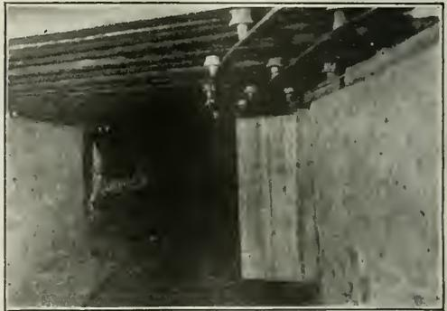
A CONCRETE OVERCAST WITH AN EXPLOSION DOOR
