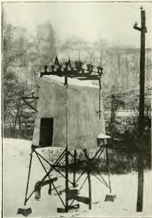
STEEL TOWER CONTAINING TRANSFORMERS PROTECTED BY HORN-GAP SWITCH AND LIGHTNING ARRESTER
