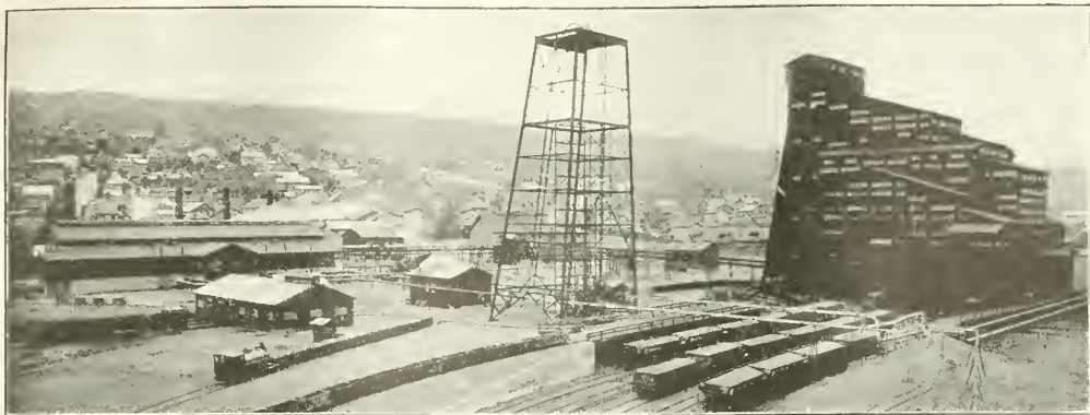
FIG. 7. NEW NOTTINGHAM BREAKER TO WHICH IS SENT THE COAL FORMERLY SENT TO THE REYNOLDS BREAKER. A considerable contrast between this and the breaker in Fig. 6. This structure belongs to the Lehigh & Wilkes-Barre Coal Co. It will be noted that some progress has been made in this breaker toward adequate lighting, though not so much light is provided as in some of the more recent breakers.
