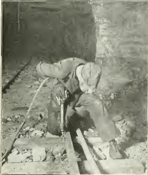
PICK HAMMER DRIVING SPIKE IN TIE
