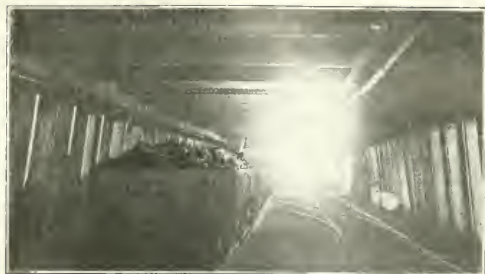
FIG. 5. STEEL TIMBERING AT LANDING
