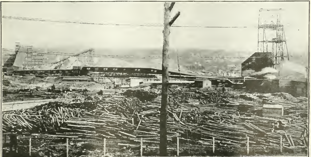
PILES OF WOOD TO BE USED IN THE MARVINE MINE OF THE HUDSON COAL CO. FOR POSTING ROOF
