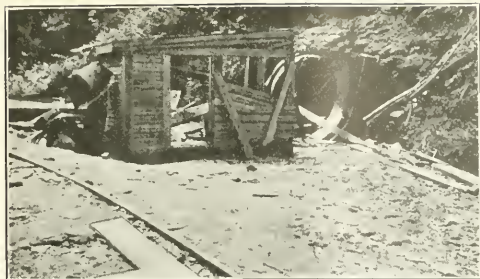
FAN HOUSE AFTER THE EXPLOSION
