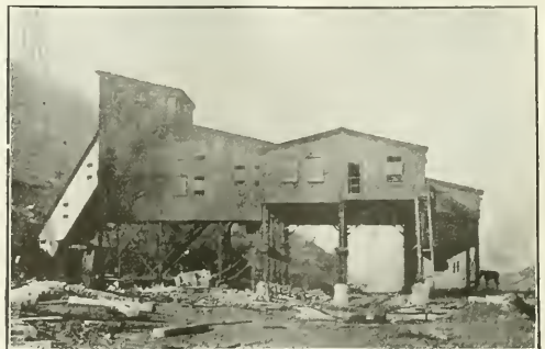
HIMLER COAL CO. TIPPLE WITH ITS 45-DEG. SLOPE
