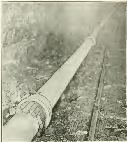
FLUSH PIPE OF CAST IRON WITH WOOD-WEDGE JOINTS
