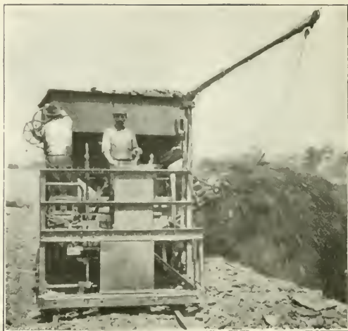
FIG. 3. CONVEYOR WIDENING A FILL—ON THE RUN
