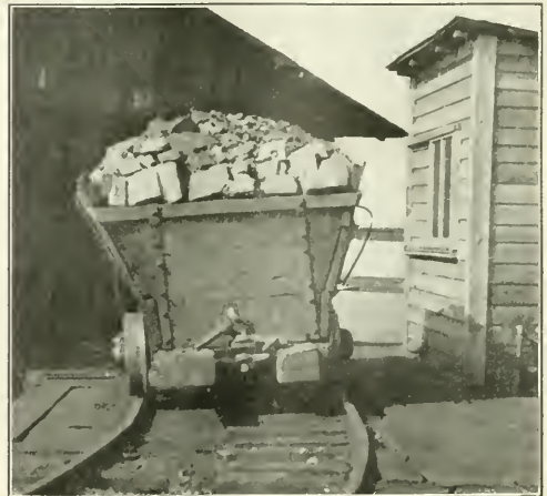
TRACK CURVES IN CROSSING MINE SCALES
