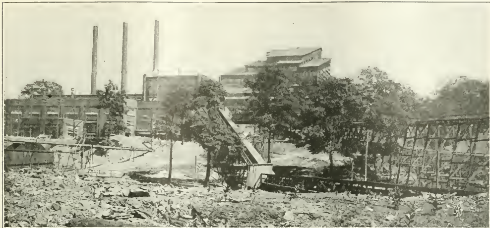
FIG. 2. LYTLE PLANT OF THE SUSQUEHANNA COLLIERIES CO. NEAR MINERSVILLE, PA. Ball mills of the type described are used in the power plant of this colliery for the crushing of anthracite. The powdered coal thus manufactured is consumed under the boilers of the power plant.
