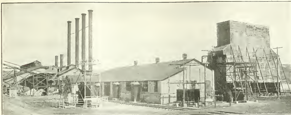
BOILER HOUSE, TURBINE ROOM, COOLING TOWER AND STEP-UP TRANSFORMERS AT ROCK SPRINGS, WYO.
