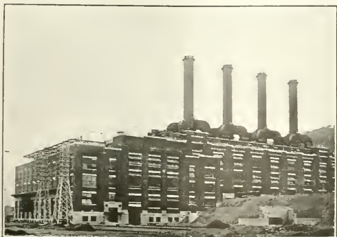
HAUTO POWER PLANT, LEHIGH COAL & NAVIGATION CO. This plant has three alternating-current General Electric Co. turbo-generators totaling 37,500 kw. The 3-phase 60-cycle current is distributed at 11,000 volts. The Babcock & Wilcox boilers generate 8,392 hp.
