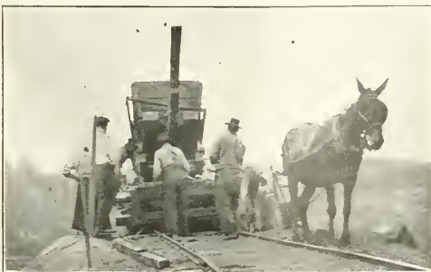
DUMPING MINE ROCK BY TURNTABLE TRUCK
