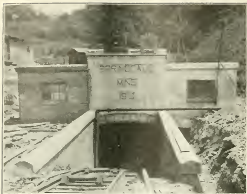
FIG. 5. SLOPE FOR HOISTING AND LOWERING MATERIAL.
