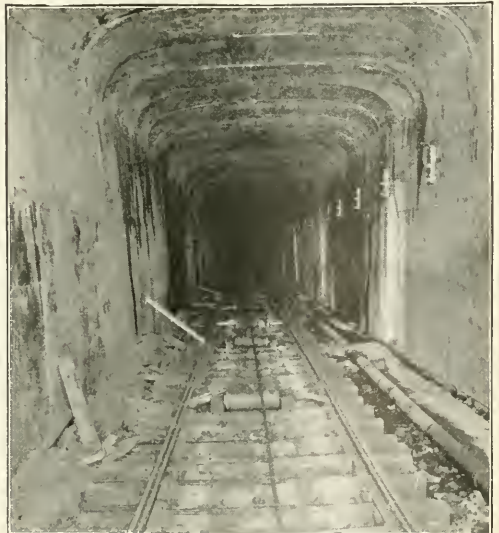
FIG. 8. LOOKING DOWN THE HAULAGE SLOPE Almost 12 ft. wide and 9 ft. 6 in. high to the springing line, this slope furnishes ample room and headway for hoisting purposes.
