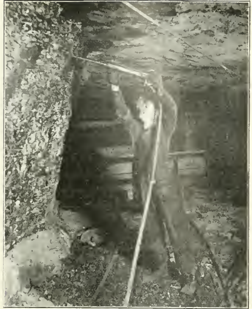
CUTTING A HITCH IN THE COAL
