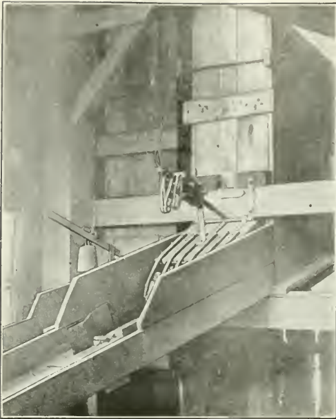
LOWER END OF TWO BOX CHUTES SHOWING FINGERED DOOR
