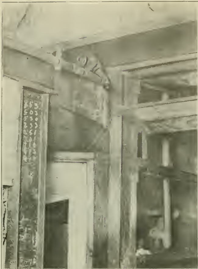
DISTRIBUTING LINES CONNECTING WITH THE MAIN In this illustration one of these lines controlled by a valve may be seen leading away from the shaft
