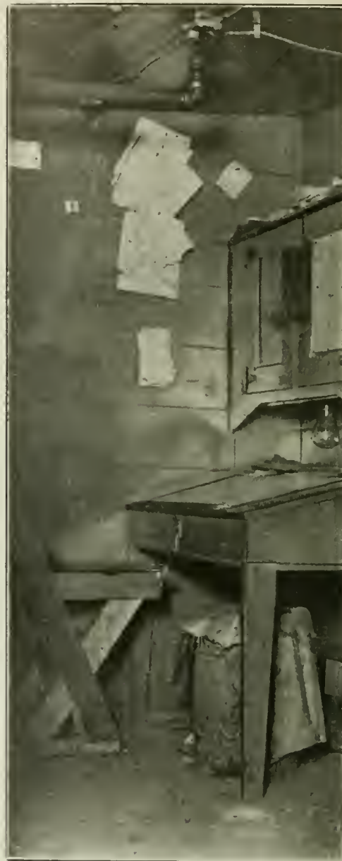
MINE MANAGER'S OFFICE PROTECTED One fused fire-plug, seen in the upper center of the illustration, protects this small room.
