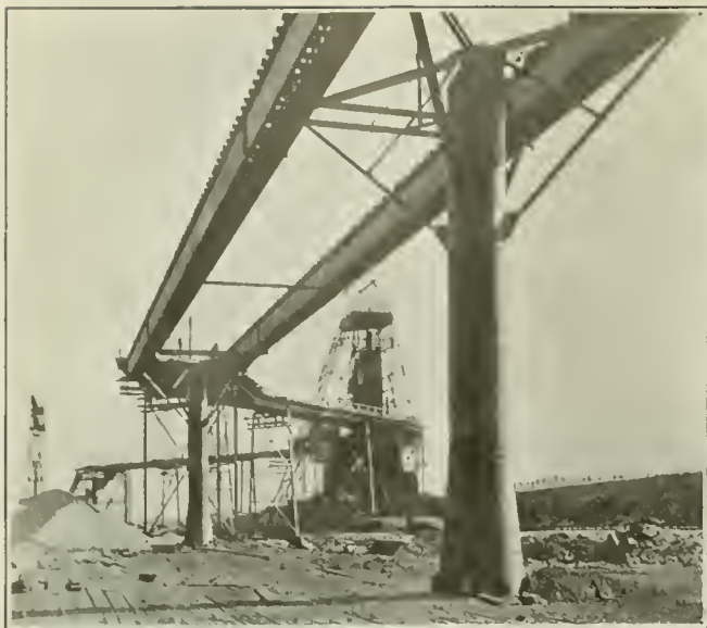
PERMANENT TREESTLE AT NEGAUNEE NO. 3 SHAFT Piers have 114 ft. centres. The height to the top of the rail is 42 ft.
