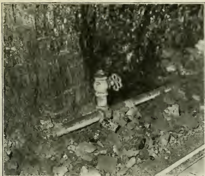
FIG. 5. TEE CONNECTION FOR SPRINKLER
