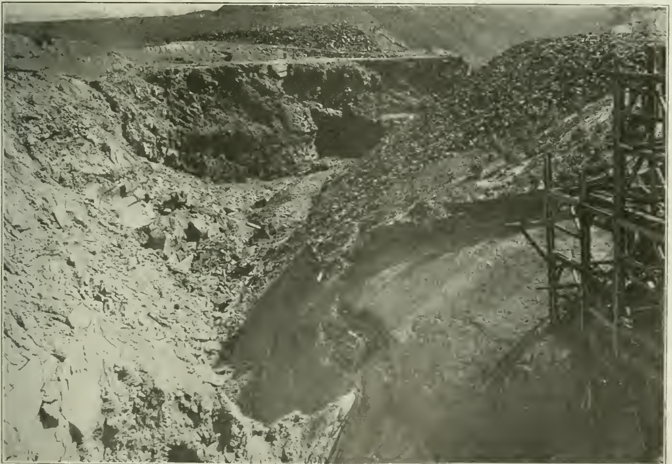
WHERE THE OCCURRENCE OF AN ANTICLINE MAKES STRIPPING POSSIBLE Anthracite stripping often differs from bituminous in the unevenness in level of the material to be stripped and in the fact that the strip material is all hauled out to a spoil bank, whereas in bituminous stripping as practiced the operation is one of casting. As the shovel in the latter pits has a long handle—about 90 ft. long—the casts of the shovel are large, but the operation is casting nevertheless.
