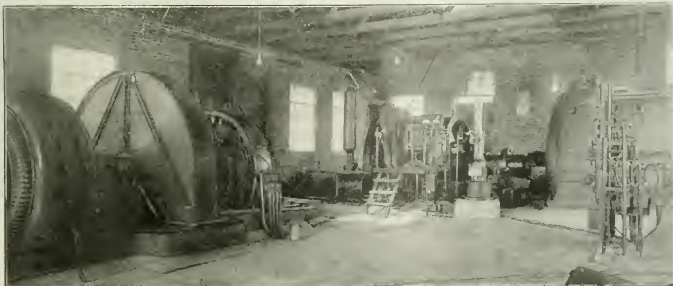
MAIN-SHAFT HOIST AND FLYWHEEL MOTOR-GENERATOR SET AT THE VALIER MINE
