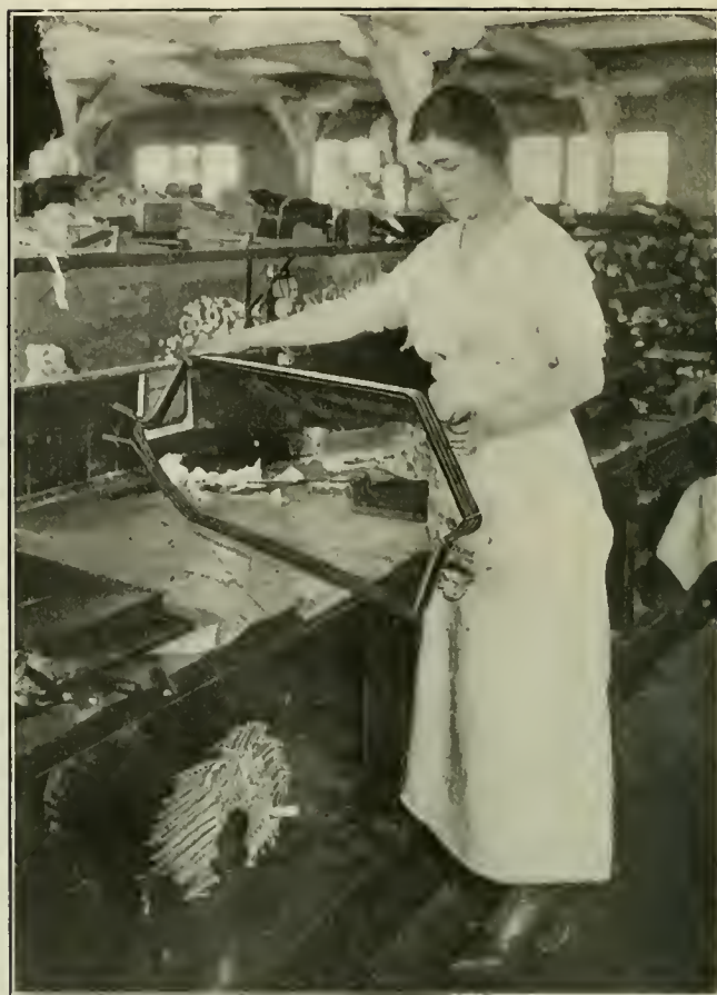
INSULATING AN ARMATURE COIL
