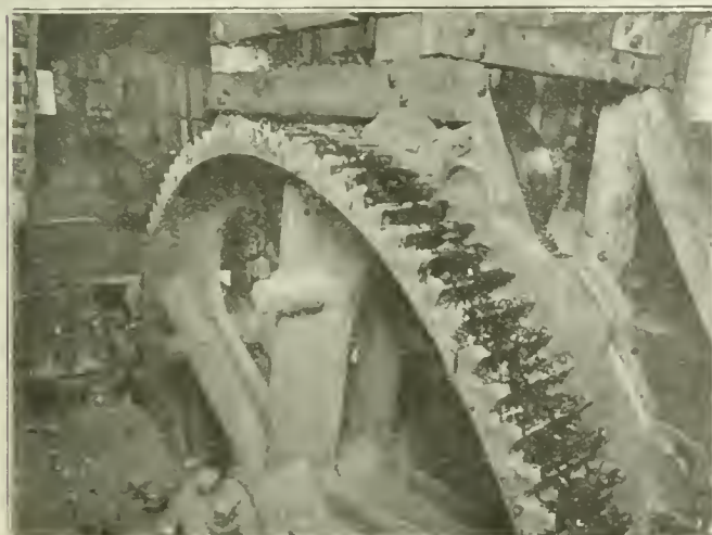
TWO VIEWS OF THE HEAD SHEAVE AND ENCLOSED BRAKE BLOCK
