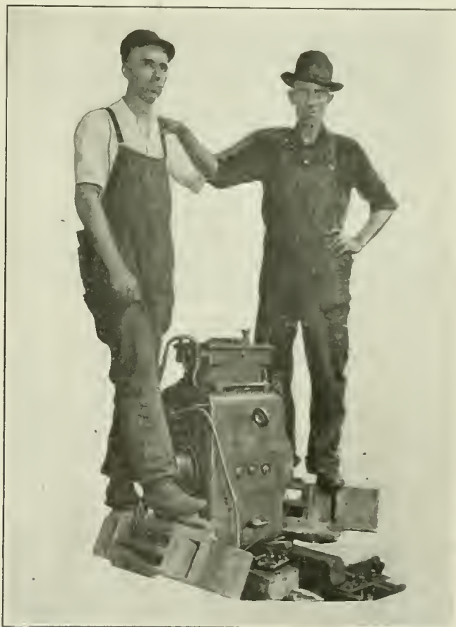
TESTING THE EFFECT OF PUTTING A JUMPER ACROSS TERMINALS OF A SHUNT COIL
