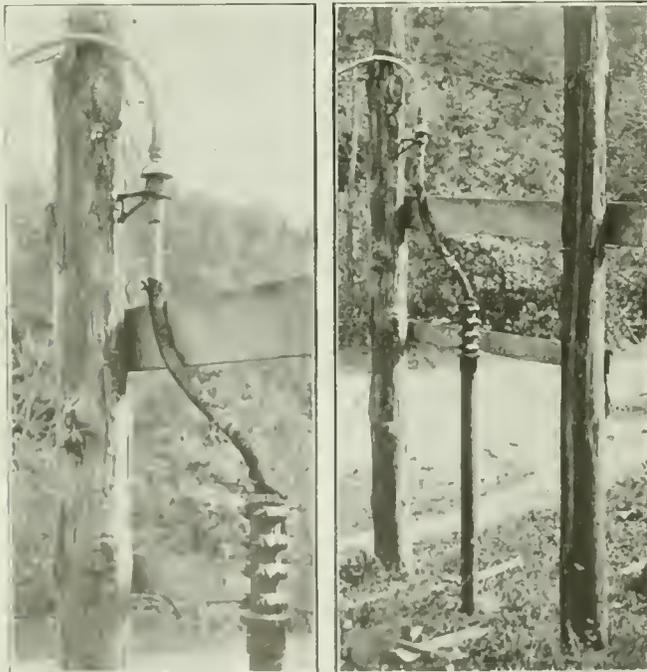
FIGS. 10 AND 11. A POWER CABLE INSTALLED IN A BOREHOLE
