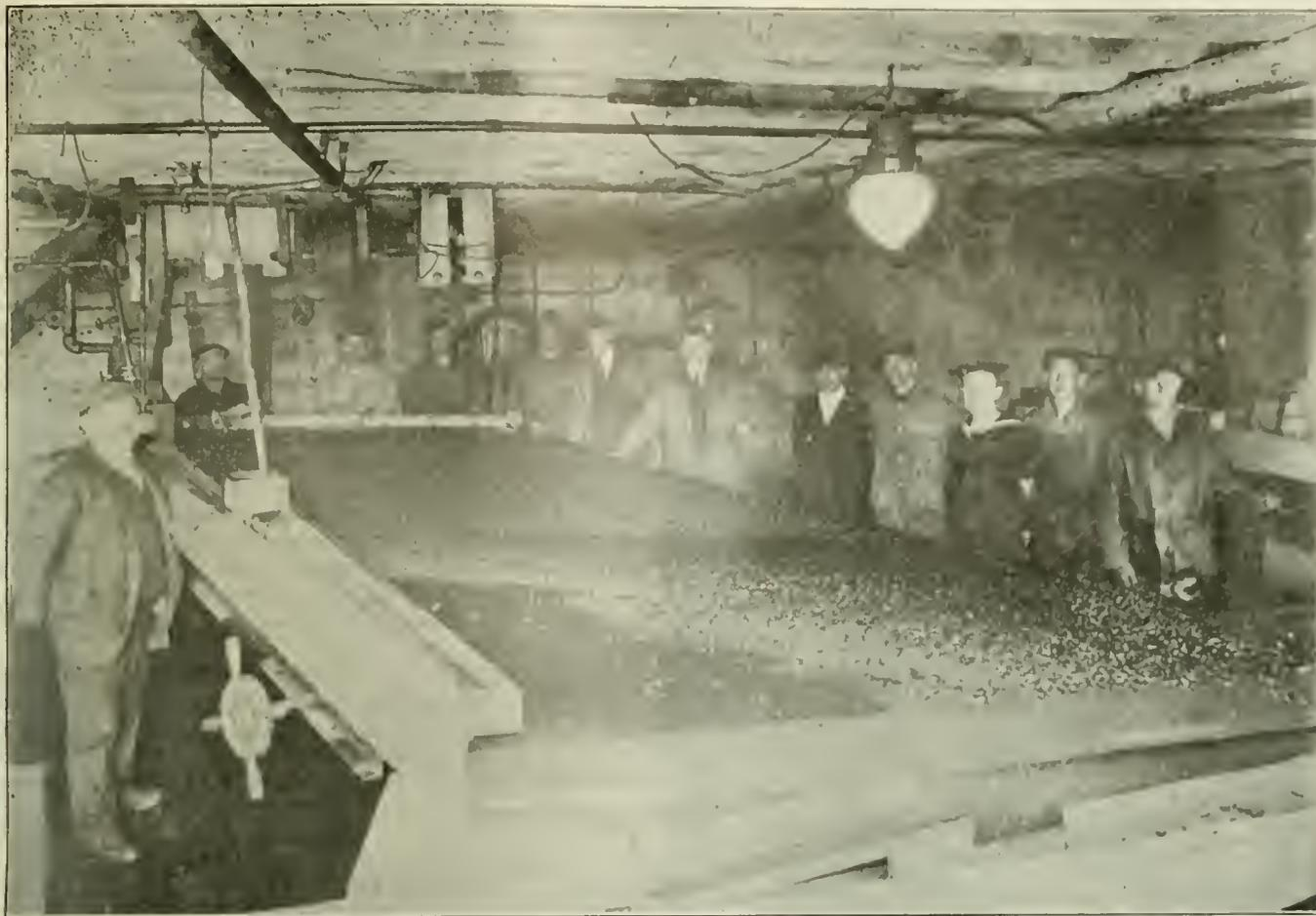
VIEW OF No. 7 DEISTER OVERSTROM WASHING TABLE IN OPERATION ON COARSE COAL FEED
