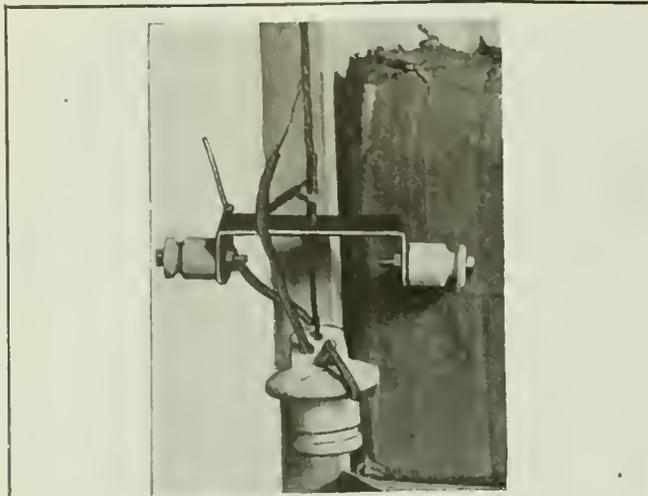
FIG. 9. BRACKET FOR SUPPORTING SMALL WIRES
