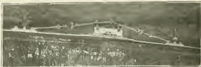
FIG. 8. A SECTION INSULATOR ANCHORED IN PLACE
