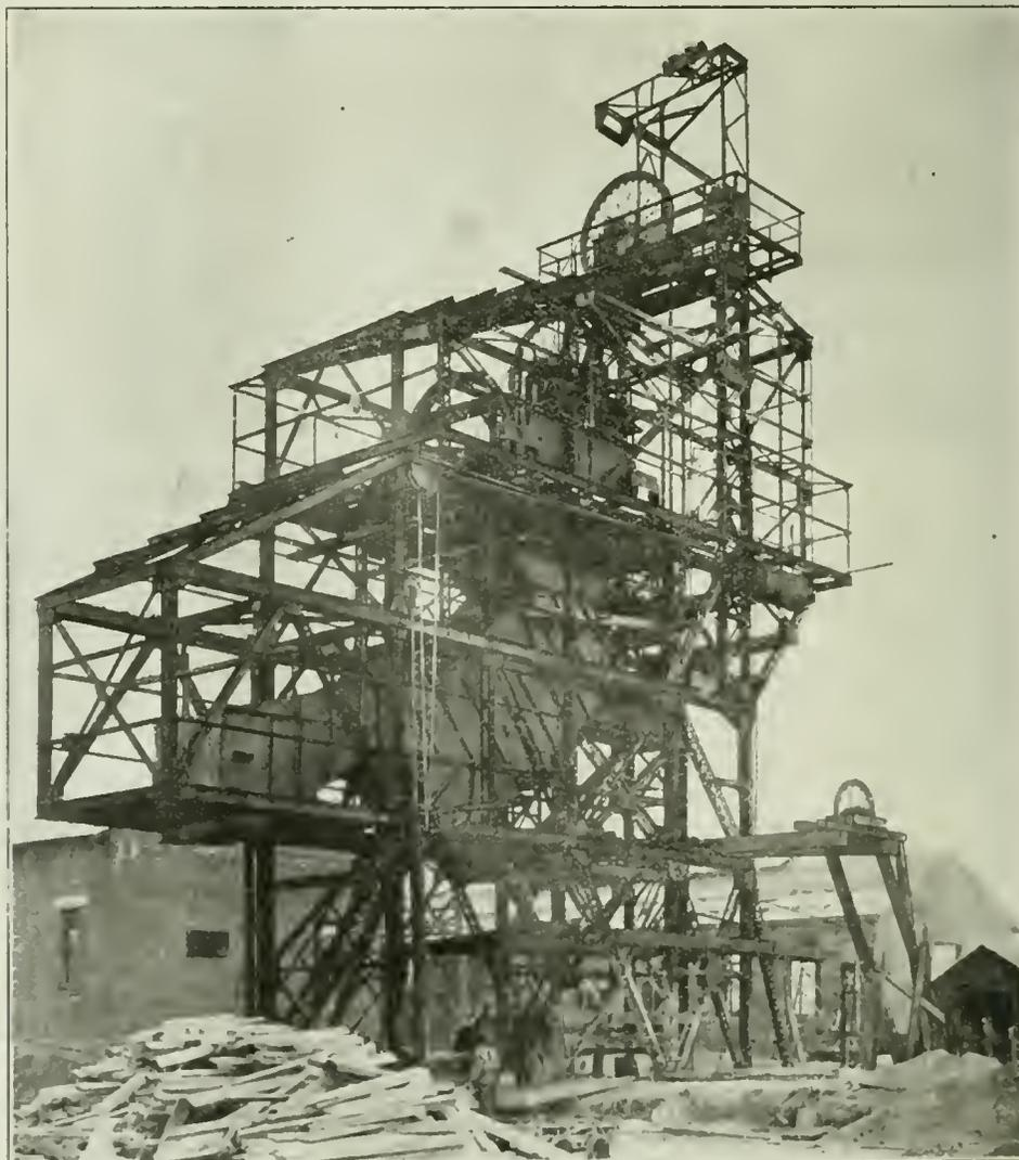
tons. At the bottom of the shaft is located a two-car rotary dump, the coal being spilled directly from this into the skips, its flow being directed by a butterfly valve. The sump extends some 50 ft. below the level of the coal and is equipped with a conveyor for the removal of waste, as well as with a small pumping station.
