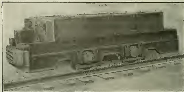
FIG. 6. A TWO-MOTOR STORAGE-BATTERY LOCOMOTIVE
