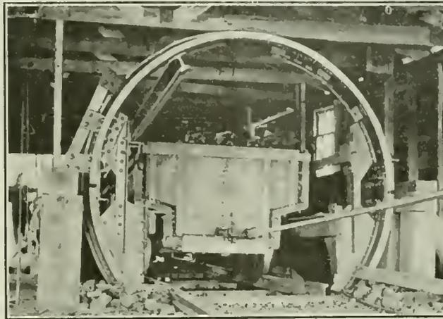
SHOWING SLOPE MINE HOISTING IN BALANCE
