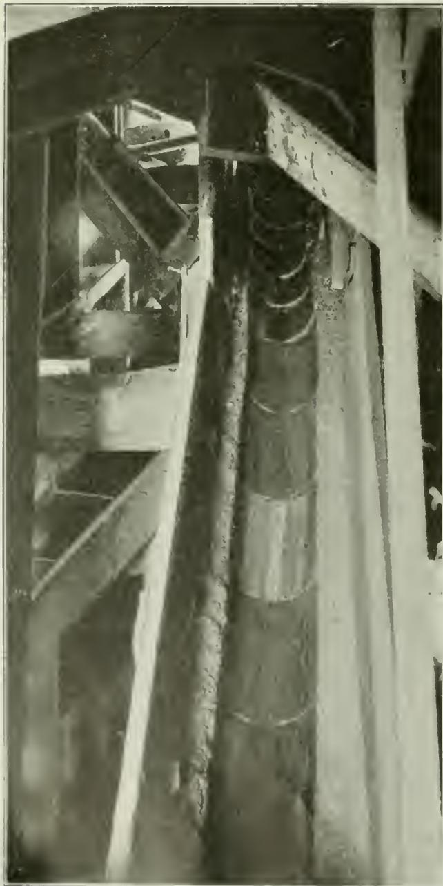
FIG. 1. VITRIFIED CLAY-LINED CHUTE
