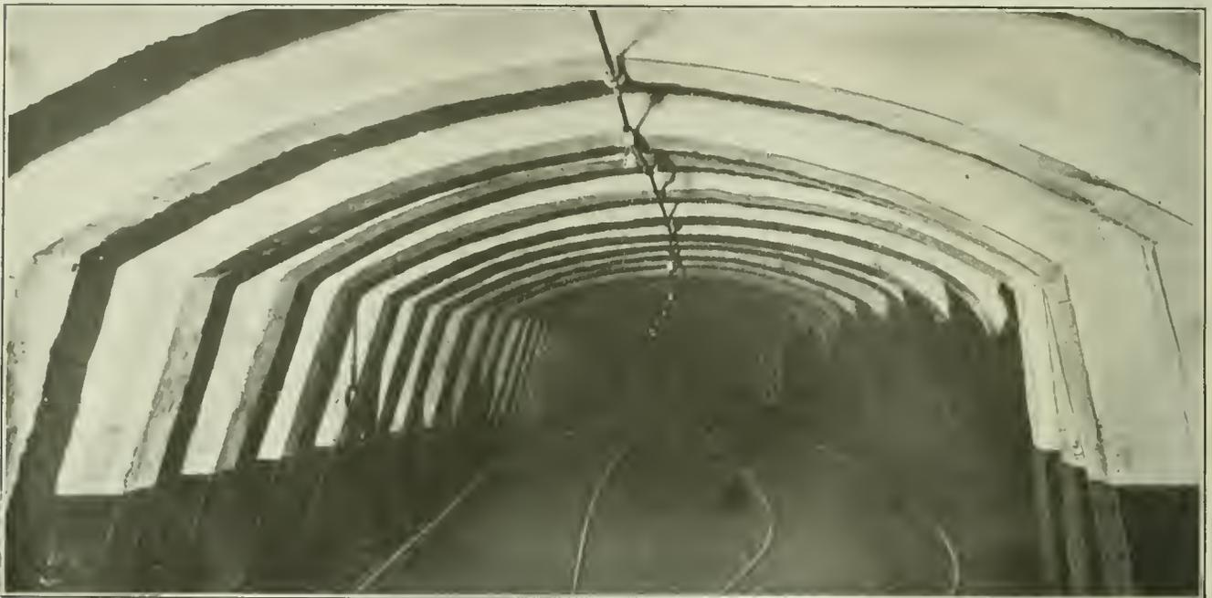
FIG. 4. CONCRETE CONSTRUCTION ON HEADING ON BOTTOM LIFT
