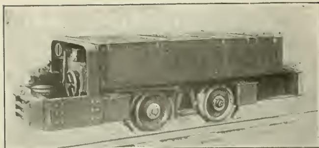
FIG. 4. NARROW LOCOMOTIVE FOR USE IN RESTRICTED PASSAGES
