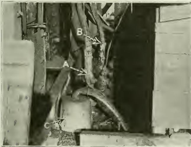
FIG. 1. THREE CABLES CARRIED DOWN THE SAME SHAFT. Two of the cables, A and B are held by clamps, the third cable is threaded through a cast-iron block, the strands spread, and spelter, or solder, poured around them. This method is applicable only for bare cables at earth potential.
