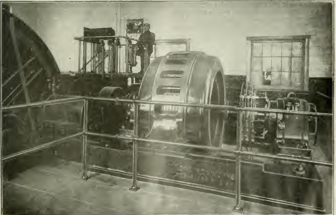
FIG. 4 FRONT VIEW OF THE DRIVING MOTOR AND OPERATOR'S PLATFORM
