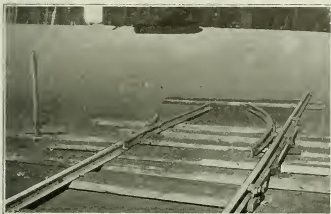
FIG. 14. SAFETY SWITCH USED ON ROOM PARTINGS
