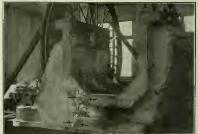
FIG. 6. WELD MADE BUT STILL IN THE ROUGH
