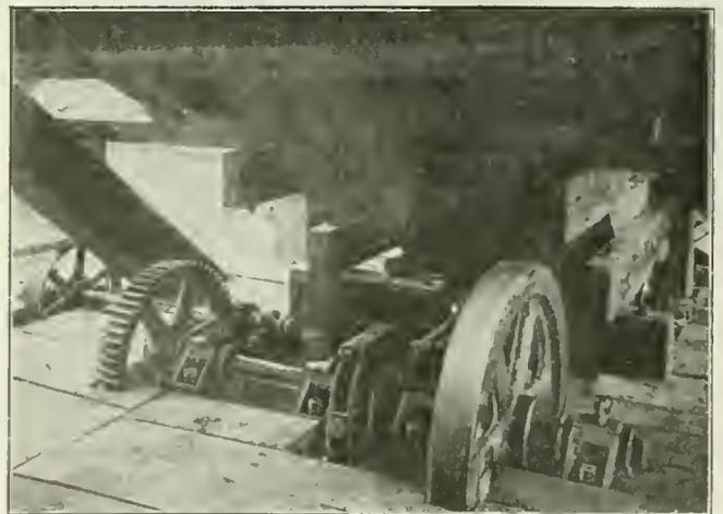
FIG. 1. MECHANISM OPERATING RECIPROCATING FEEDER
