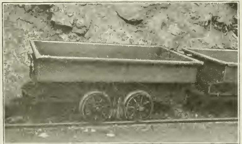
angle extends over the top of the car box, while the other lies along the side. These four angle irons thus hold the cars in place while the trip is being revolved and the cars emptied.
