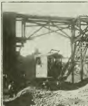
SPECIAL MACHINES ARE SOMETIMES BUILT FOR STORING AND RECLAIMING COAL
