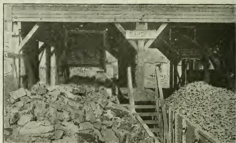
tributed upon the retarding conveyor by a reciprocating feeder, which insures a uniform supply. This is an advantageous method.
