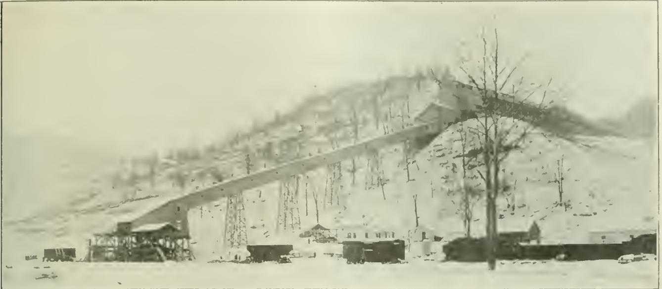
FIG. 1. A MIDWINTER SCENE AT THE BUD MINE SHOWING TIPPLE, RETARDING CONVEYOR AND HEAD-HOUSE
