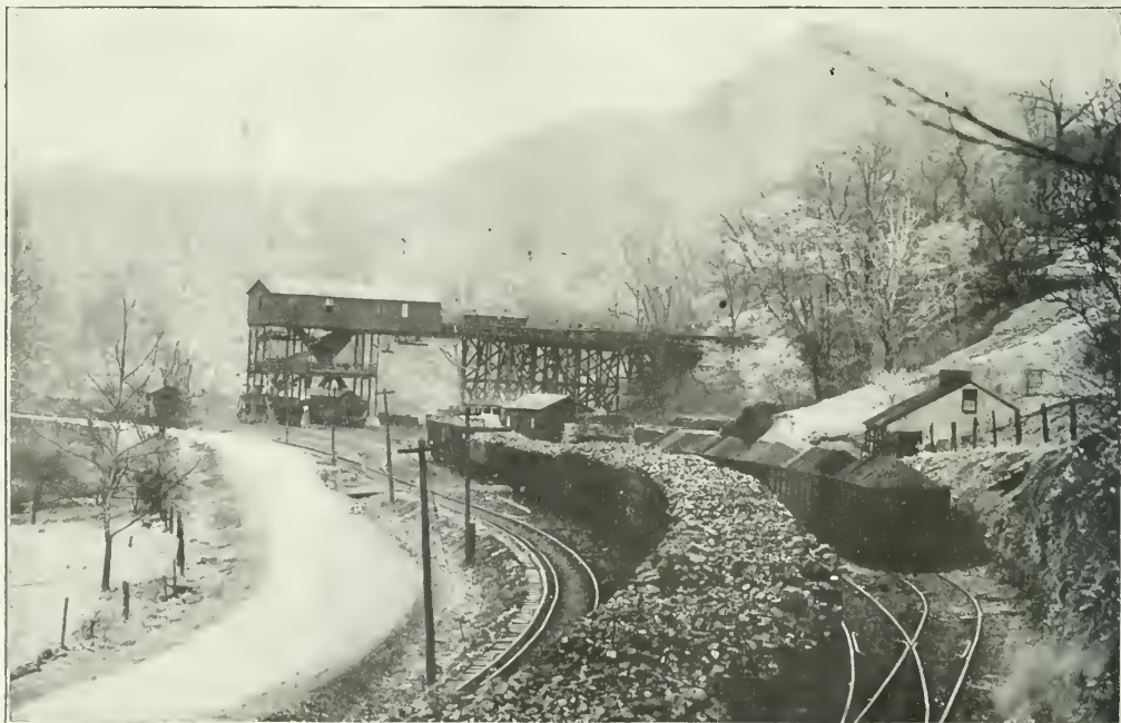
VIEW OF THE TIPPLE OF THE PATTERSON MINE, OWNED BY J. H. HILLMAN & SONS CO., OF PITTSBURGH, PENN. The mine is located near McKeesport, Penn., on the Monongahela River. In the cars is shown the day's loading of 3-in. and slack coal. The operation is in the Pittsburgh seam.
