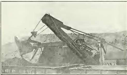
TWO VIEWS OF THE STEAM SHOVEL AT WORK LOADING THE STORED COAL
