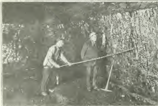
ILLUSTRATING TWO GENERALLY FOLLOWED METHODS OF BORING A SHOTHOLE
