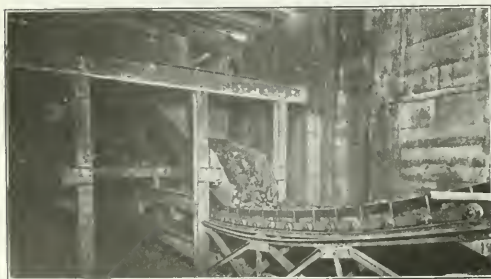
FIG. 5. RECIPROCATING FEEDER WITH OSCILLATING BOTTOM
