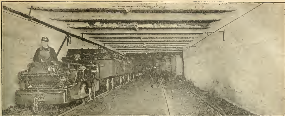
STEEL AND CONCRETE CONSTRUCTION NEAR THE SHAFT BOTTOM
