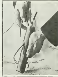
DIFFERENT STEPS IN PRIMING WITH AN ELECTRIC DETONATOR
