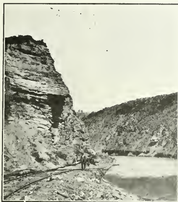
VIEW UP THE CUT, OVERBURDEN SHOWN ON LEFT AND SUMP ON RIGHT
