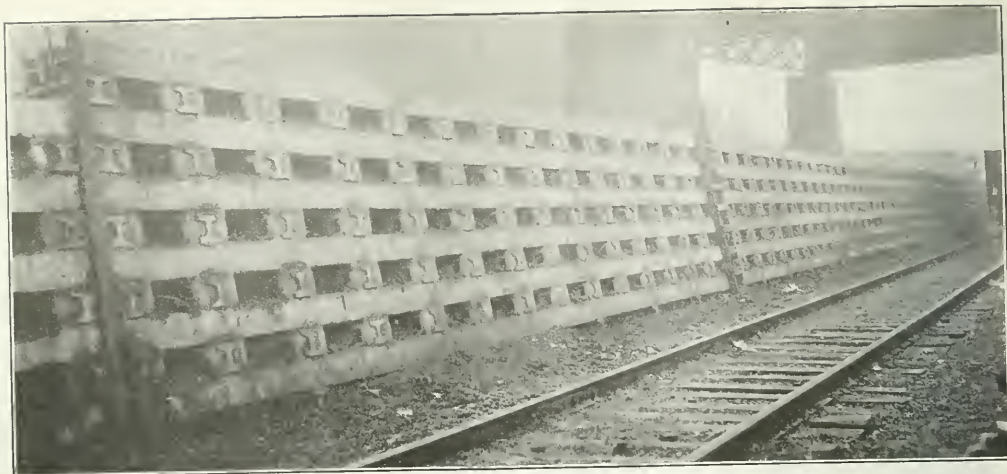
FIG. 2. SECTIONAL CONCRETE RETAINING WALL IN PERMANENT FORM
