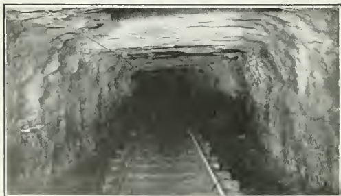
FIG. 3. ENTRY TREATED WITH CEMENT COATING
