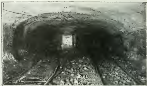
FIG. 4. JUNCTION POINT OF TWO HAULAGE ENTRIES TREATED WITH CEMENT COATING
