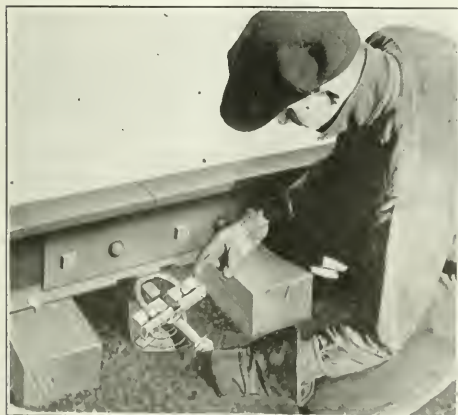
SLIDING A BOND INTO POSITION UNDER THE RAIL AND WELDING IT IN PLACE
