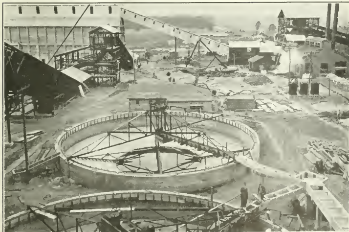
FIG. 22. DORR THICKENER, 70 FT. IN DIAMETER, WITH CONCRETE TANK
