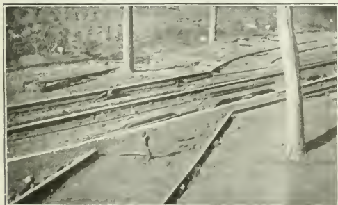
FROGLESS CROSSOVER TRACK, SHOWING FORKED ROD AND LOCKING LEVER (ON LEFT) AND RAILS REMOVED FROM UNDER TRACK (ON RIGHT)
