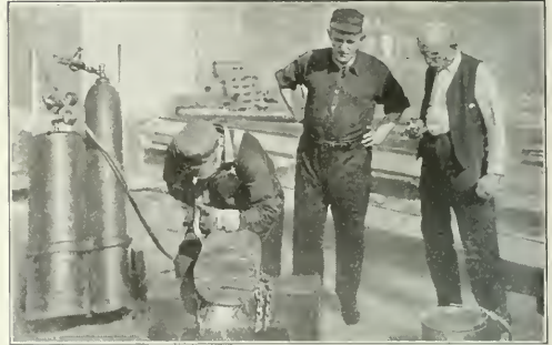
FIG. 4. CUTTING A 10-IN. SHAFT
