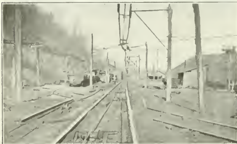
FROGLESS CROSSOVER TRACK, SHOWING FORKED ROD AND LOCKING LEVER (ON LEFT) AND RAILS REMOVED FROM UNDER TRACK (ON RIGHT)
