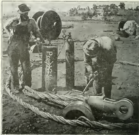
FIG. 9. REPAIRING WIRE CABLE
