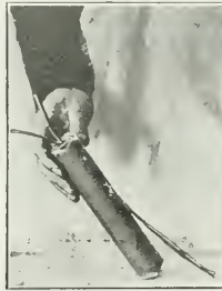
DIFFERENT STEPS IN PRIMING WITH AN ELECTRIC DETONATOR
