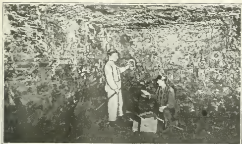
LOADING A HOLE WITH PERMISSIBLE EXPLOSIVE
