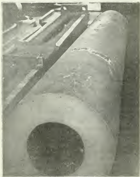
FIG. 14. A WELDED PUMP PLUNGER
