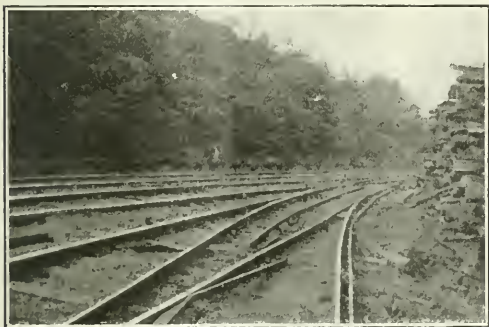
HINGED MINE RAIL IN RAILROAD YARD
