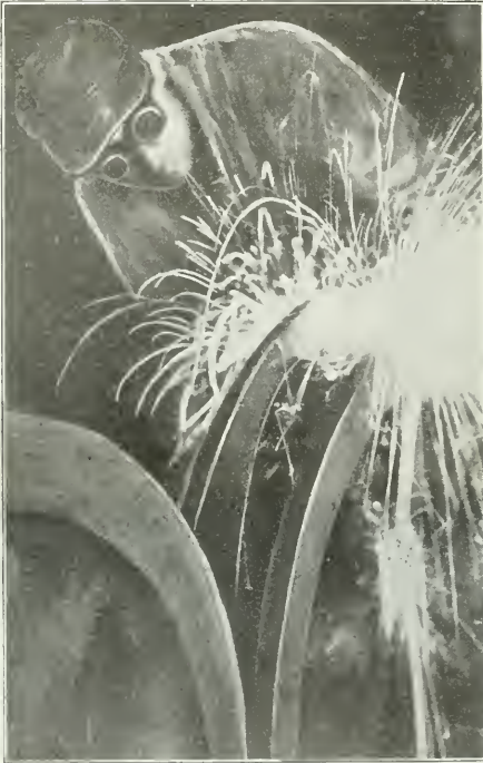
FIG. 3. CUTTING TIRE OF LOCOMOTIVE WHEEL
