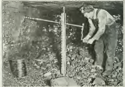
ILLUSTRATING TWO GENERALLY FOLLOWED METHODS OF BORING A SHOTHOLE
