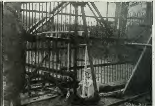
SAME SAFETY DEVICE WITH LATCH OPEN. THE CAGE HAS RISEN, AND ACTING AS A FULCRUM HAS PERMITTED CAGER TO OPEN GATE
