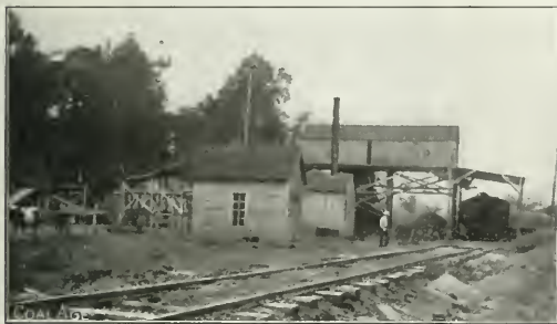
TIPPLE AT MINE OF FORSYTHE COAL CO., PROVIDENCE, KY. OUTPUT 150 TONS PER DAY, COAL SHOT FROM SOLID
