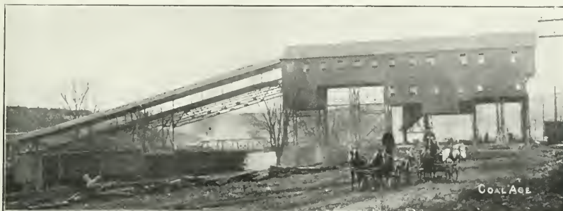
TIPPIE AND INCLINE UP WHICH CARS TRAVEL
