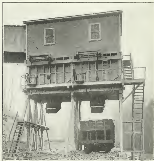
FIG. 3. RUN-OF-MINE LOADING BIN FITTED WITH TWO LARGE CHUTES
