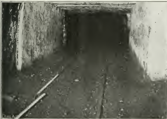
FIREPROOF OVERCAST OF CONCRETE WITH STEEL AND TILE ROOF
