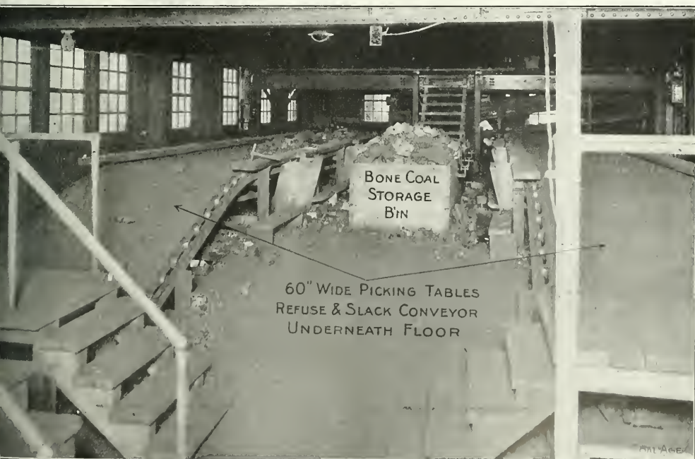
FIG. 5. TWO OVERLAPPING, CORRUGATED APRON TYPE PICKING BELTS, 35 FT. LONG
