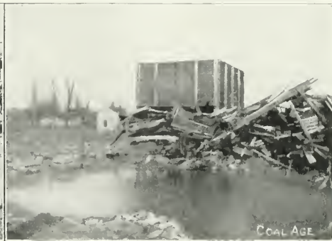
AFTER THE TIPPY HAD SUNK OUT OF SIGHT BY UNDERMINING
