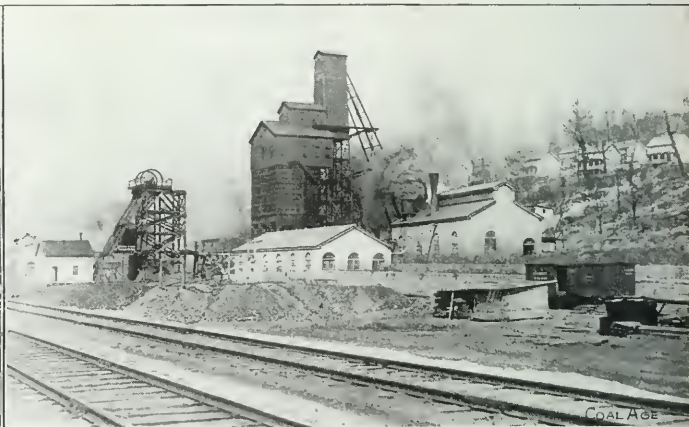
SURFACE WORKS AND COKE PLANT OF THE ISABELLA CONNELLSVILLE COKE CO. HEIGHT OF HEADFRAME, 180 FT.
