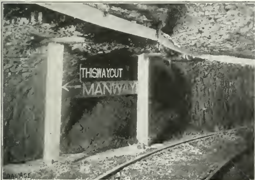
TROLLEY-WIRE PROTECTION AND SIGN POINTING THE WAY OUT
