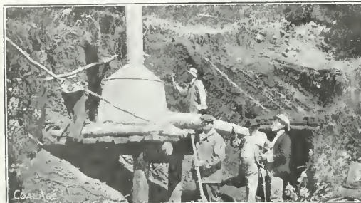
VENTILATING A PROSPECT TUNNEL IN BRITISH COLUMBIA
