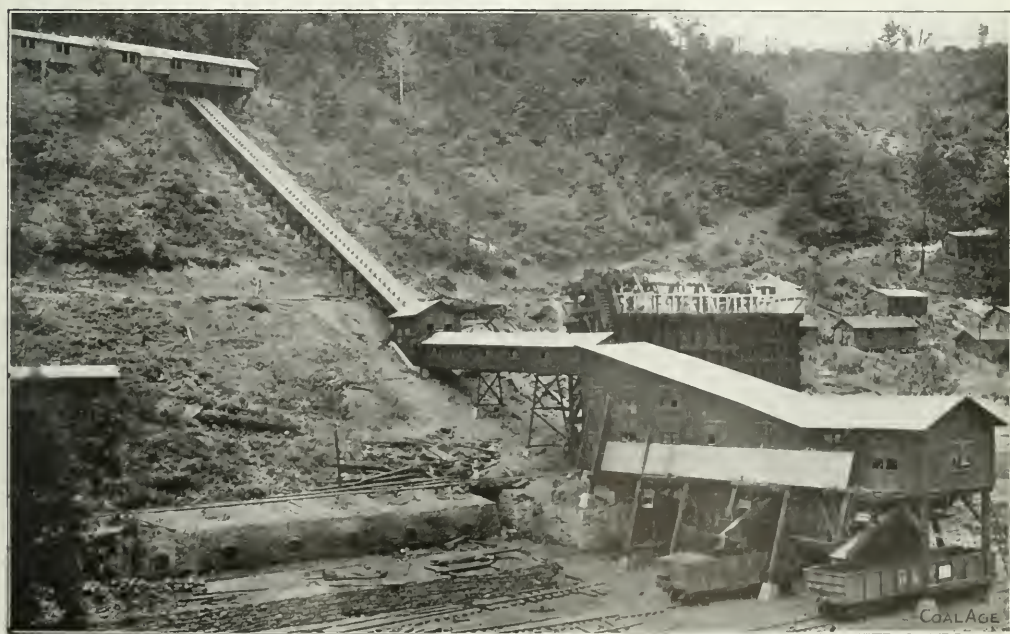
JEFFERY STEEL TIPPLE AND RETARDING CONVEYOR, ROANOKE COAL & COKE CO., BEAR HOLLOW, W. VA.
