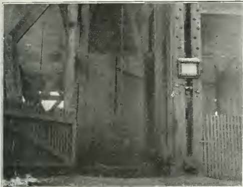
STEEL DOORS TO DROP OVER SHAFT MOUTH IN CASE OF FIRE
