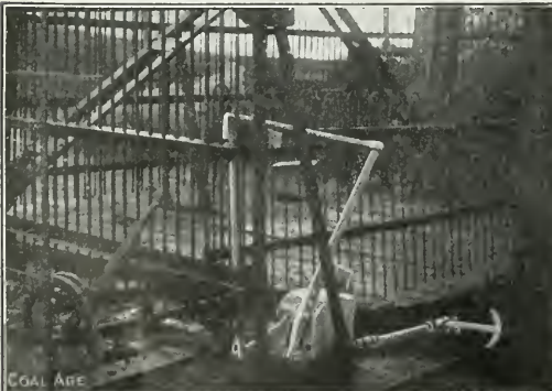
A SAFETY SHAFT-GATE LATCH, WHEN CAGE IS NOT AT LANDING, LATCH WILL NOT OPEN. GATE REMOVED TO SHOW MECHANISM
