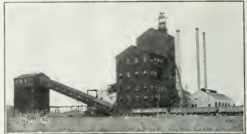
VIEW OF ZIEGLER COLLIERY, SHOWING RESCREENER WITH CONNECTING CONVEYOR
