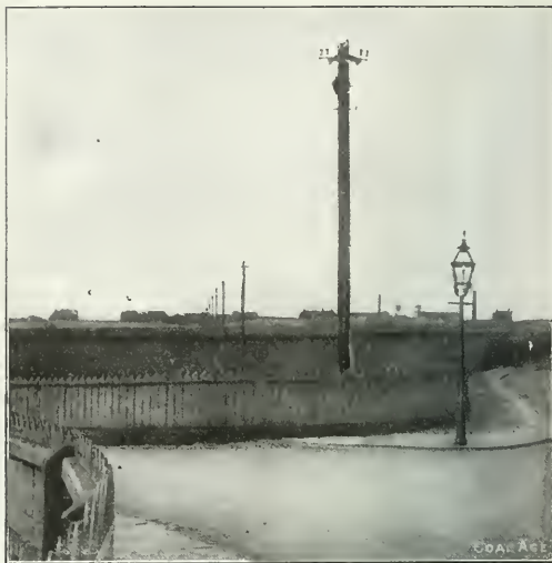
FIG. 3. EXTRA HEIGHT, THREE-PHASE TRANSMISSION LINE
