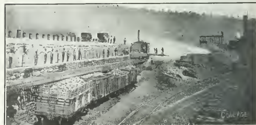
THOMAS TYPE OF COKE OVENS AT COALBURG, ALA. PROBABLY FIRST MECHANICALLY DRAWN OVENS IN UNITED STATES
