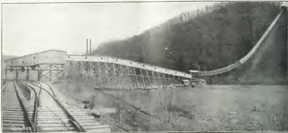
RETARDING CONVEYOR OF THE HARLAN COAL MINING CO. TAKEN BEFORE COMPLETED
