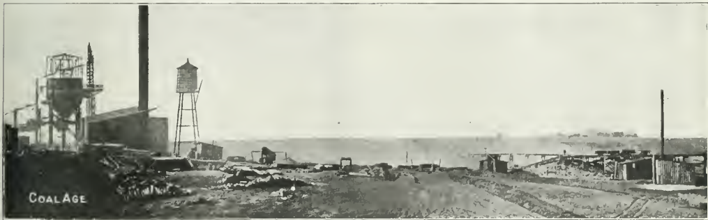
NO. 1 PLANT CONSOLIDATED INDIANA COAL CO., DALLAS, IND. AN ESCAPEWAY IS BEING CONSTRUCTED ON THE RIGHT ON A 17-DEG. SLOPE, BY WHICH MEN WILL ENTER MINE. NO MEN WILL BE HOISTED
