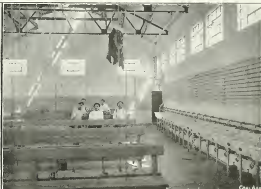
EXTERIOR AND INTERIOR VIEWS OF BATH HOUSE AT UNIVERSAL MINES, CONSTRUCTED OF REINFORCED CONCRETE WITH STEEL WINDOW FRAMES AND CEMENT TILE ROOF
