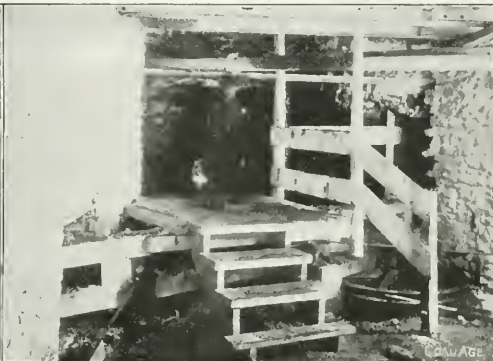
STILE OVER ROPE SHEAVES TO PROTECT TRAVELING MEN
