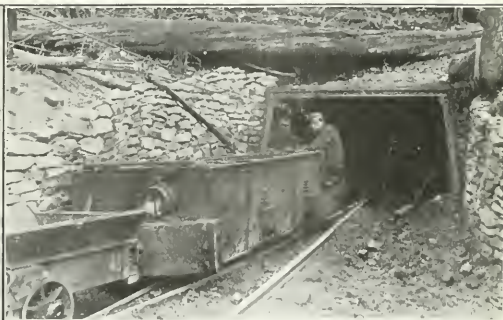
FIG. 3. AN ENTRANCE TO NO. 7 MINE, SHOWING IRON-RAIL TIMBERS AND A BALDWIN-WESTINGHOUSE MOTOR
