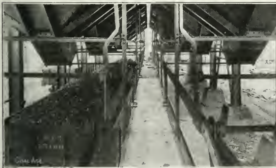
VIEW OF TRACKS AND UNDERSIDE OF BINS BENEATH RESCREEENER
