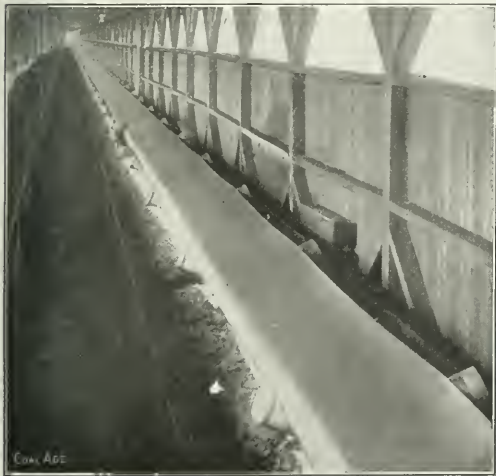
FIG. 7. A 22-IN. BELT CONVEYOR 1050 FT. LONG
