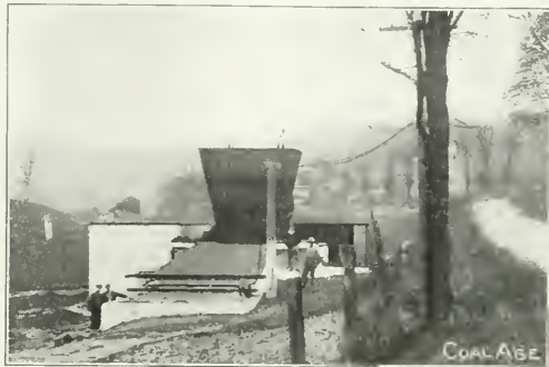
ELECTRICALLY DRIVEN MINE FAN. THE EXPLOSION DOORS IN THE FOREGROUND WERE BLOWN OPEN BUT THE FAN WAS UNINJURED
