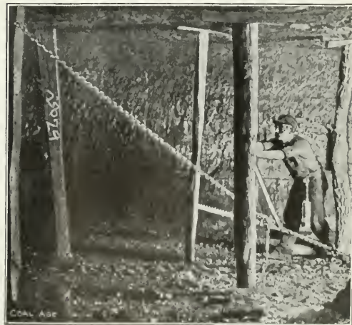
FIG. 1. DRAWING A POST IN THE THIRD ROW FROM THE FACE OF AN ADVANCING ROOM
