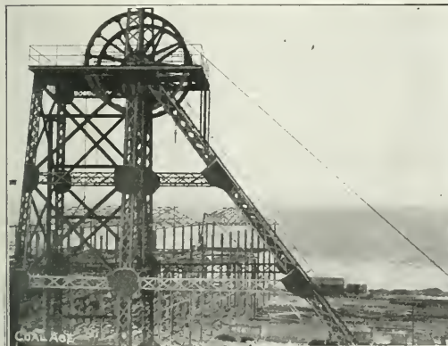
HEADFRAME AND SCREENING PLANT UNDER CONSTRUCTION AT WELLESLEY PIT, WEYMSS COAL CO., DENBEATH, SCOTLAND
