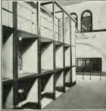
BACK VIEW OF SWITCH GEAR
