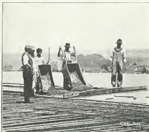
FIG. 11. CONCRETING A HY-RIE ROOF
