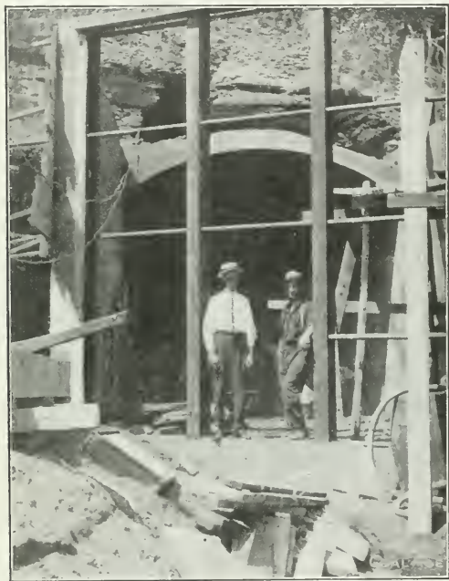
EXPLOSION-DOOR FRAME AND PIT MOUTH DURING ERECTION
