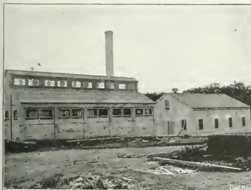
EXTERIOR AND INTERIOR VIEWS OF BATH HOUSE AT UNIVERSAL MINES, CONSTRUCTED OF REINFORCED CONCRETE WITH STEEL WINDOW FRAMES AND CEMENT TILE ROOF
