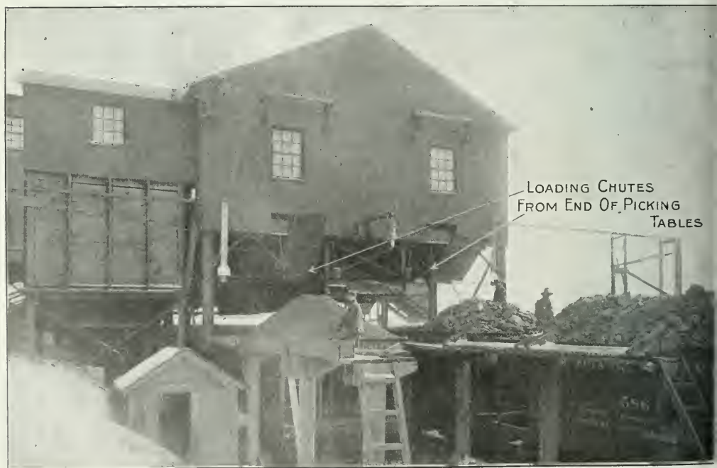
FIG. 3. NEAR VIEW OF THE TIPPLE, SHOWING THE METHOD OF LOADING CARS
