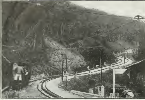
INCLINED ELECTRIC RACK-RAIL HAULAGE SYSTEM
