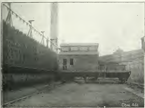
COKE PUSHER WORKING AT BATTERY No. 8
