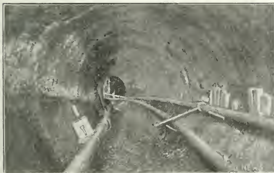
FIG. 3. A 6-FT. DIAMETER HEADING, ON A 10-DEG. CURVE DRIVEN WITH THE KARN'S MACHINE
