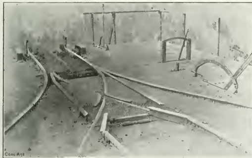
FIG. 2. THE SWITCHES OVER THE UPPER BIN, PERMITTING RAPID DUMPING OF COAL
