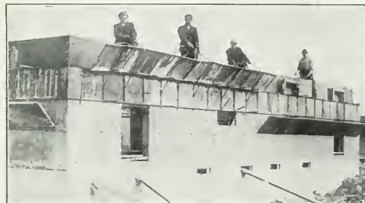
FIG. 7. RAISING A BELT. NOTE WINDOW AND DOOR FRAMES
