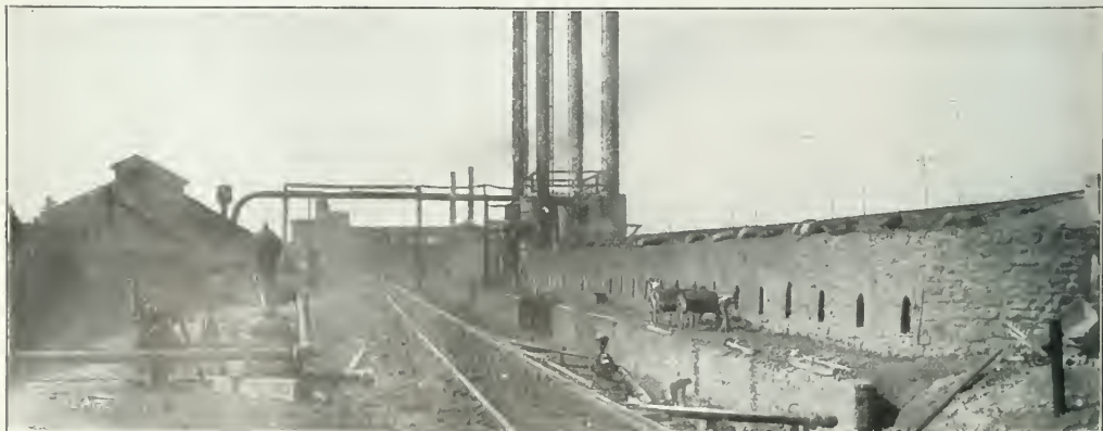
UTILIZATION OF WASTE HEAT FROM BEEHIVE OVENS
