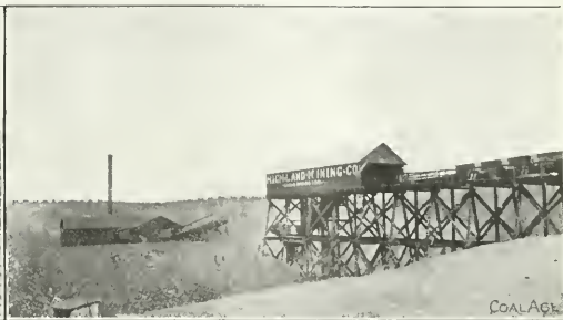
SURFACE PLANT OF HIGHLAND MINING CO., PROVIDENCE, KY. A 700-TON MINE, VENTILATED BY A 16-FT. CRAWFORD AND McCRIMMON FAN
