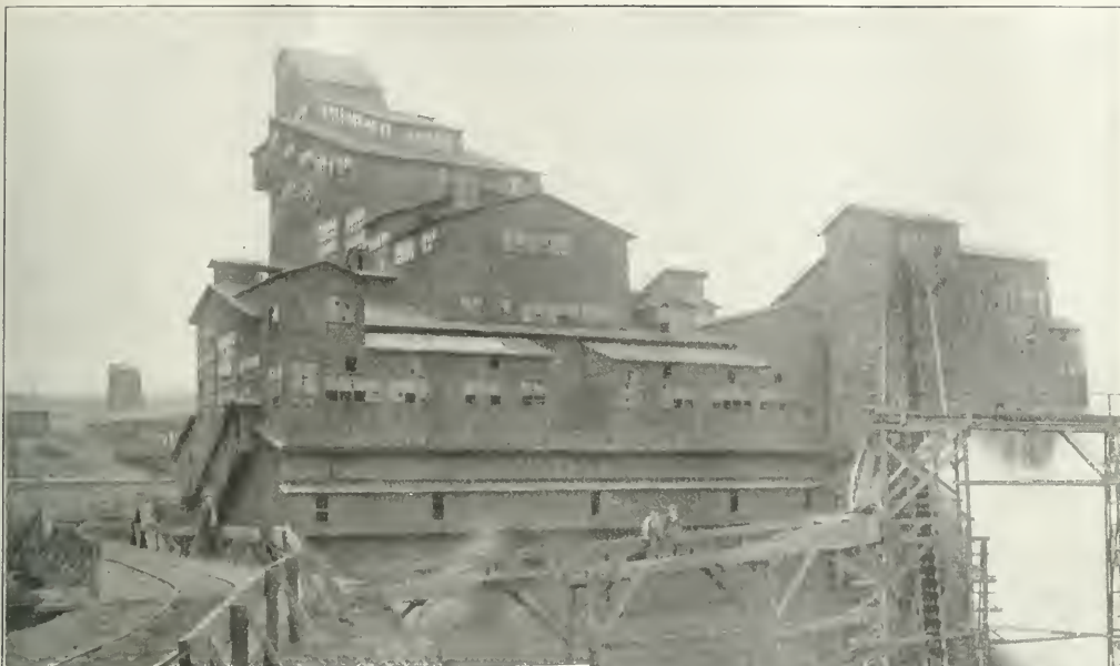
BUTTONWOOD WASHERY AND BREAKER, SHOWING MAIN CONVEYOR AND INCLINE TO WASHERY
