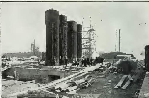
FOUR VERTICAL WATER-TUBE BOILERS SET UPON CONCRETE FOUNDATIONS PREPARATORY TO BRICK-ING IN. A PART OF THE PLANT SHOWN AT THE LEFT OF THIS PHOTO.
