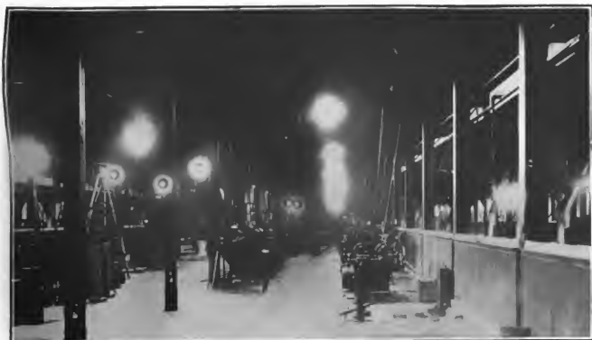
A 480-foot lane of gas-arc-lighted automatic machines, in the "south bay" of the National Brake & Electric Co.'s shops.
