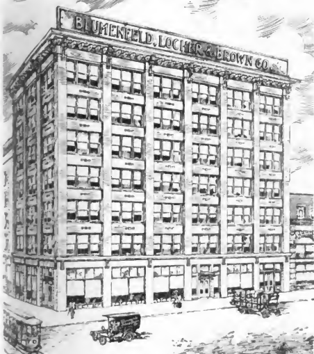
Building now being erected at Broadway and Mason Sts. for Blumenfeld, Locher & Brown Co., The Progressive Millinery House of Milwaukee
