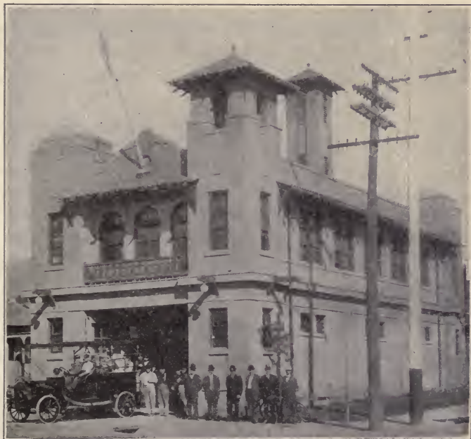
FIRE ENGINE HOUSE.
