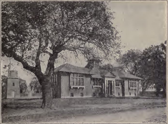
TYPICAL RURAL SCHOOL BUILDING, SONOMA COUNTY, CAL.
