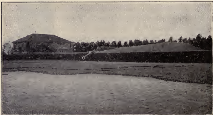
FILTER BED OF THE INDIANAPOLIS WATER WORKS.
