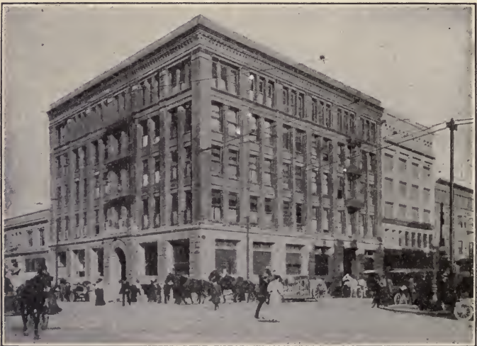
CENTRAL BANK BUILDING, OAKLAND, CALIFORNIA.
