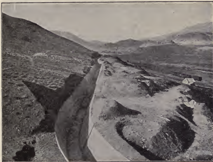
TRUCKEE IRRIGATION CANAL, NEVADA.
