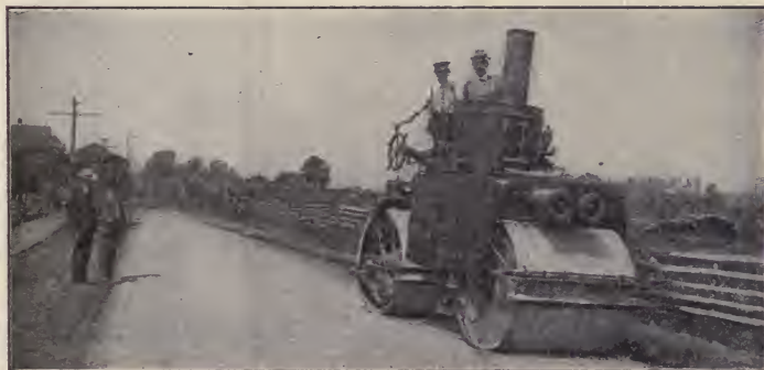
3. Finishing the road.
