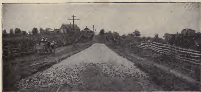
2. Laying the foundation course.
