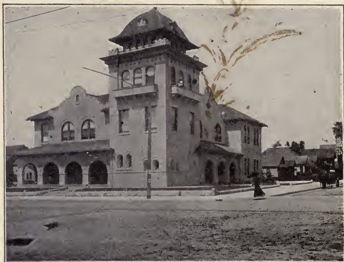
CITY HALL, SANTA MONICA, CAL.
