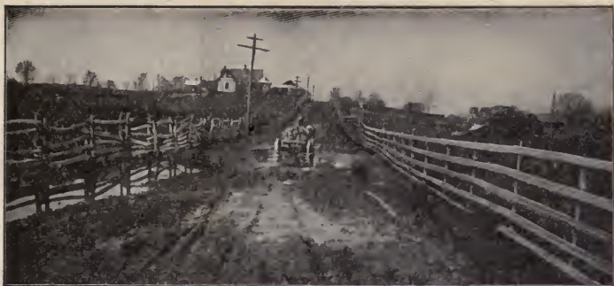
1. The road in its original condition.
