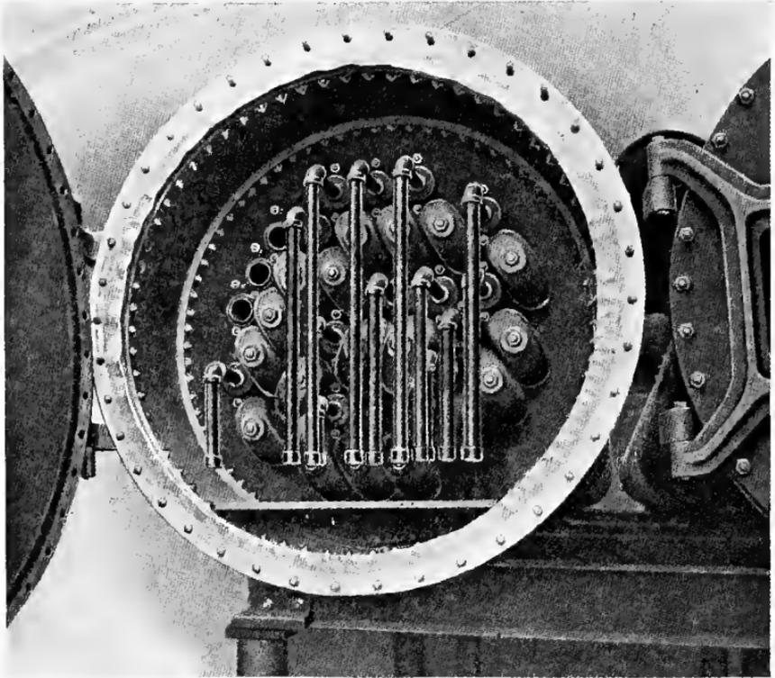
FIG. 18. YARYAN EVAPORATOR FEED END OF ONE EFFECT
