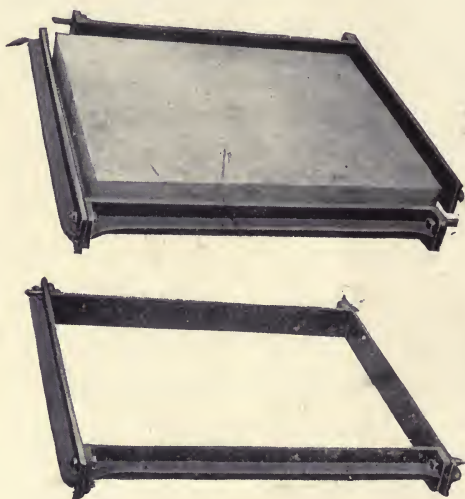
FIG. 87.—Mould for Slabs.
