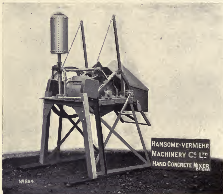
FIG. 38.—Hand Mixer for Concrete.
