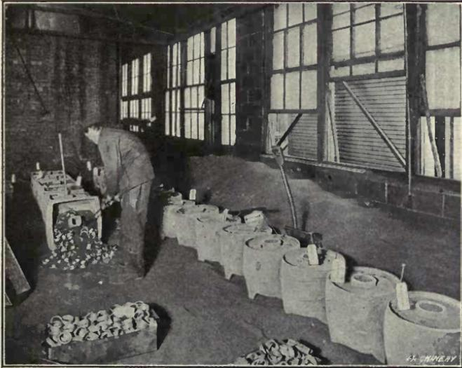
Fig. 3. Dumping and sorting Work that has been carbonized
