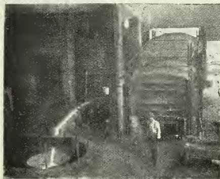
Catching the molten metal from the air furnace into the ladle
