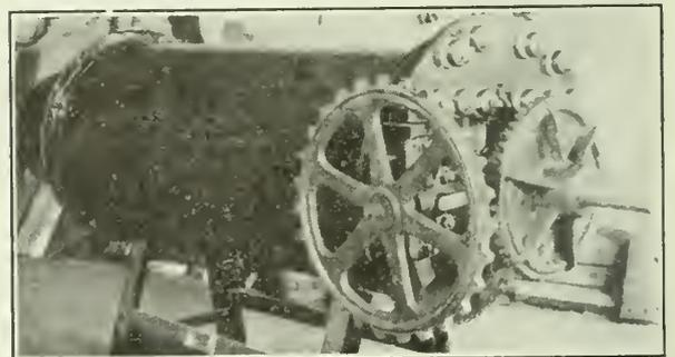
Automatic electric furnace for heat-treating small parts. These are fed in at one end, carried through by worm, and released at other end.
