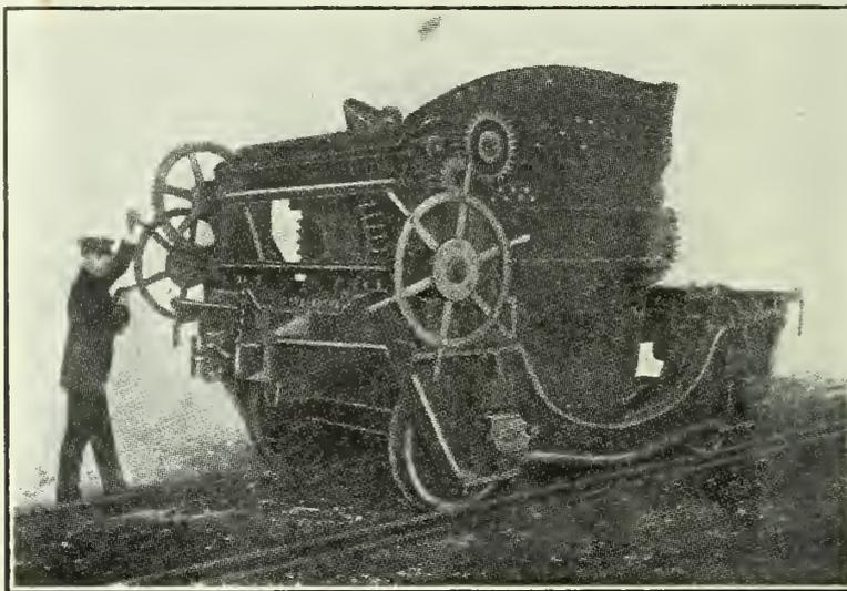
Hundred-ton ladle which can be handled in perfect safety by one man. This ladle can be filled at the furnace and taken to the machine, wherever located. Machine and ladle are always ready. No pig beds to get in readiness.
