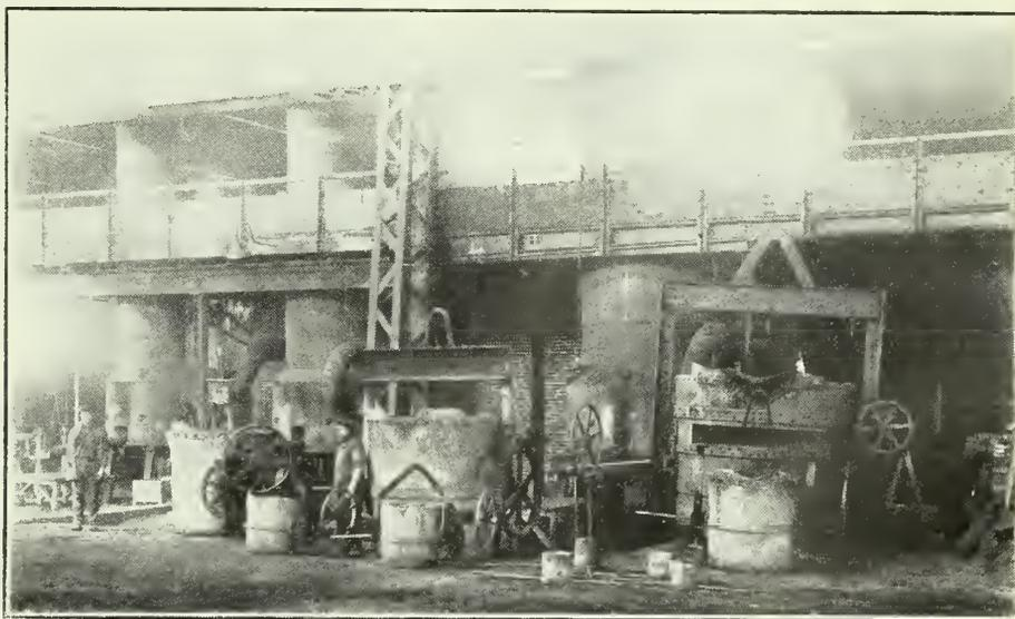
Fig. 1.—Cupolas and Ladle Equipment of Foundry consisting of, One 37", One 54" and One 84" cupolas, giving a melting capacity of 35 tons per hour. Ladles range in capacity from 1 ton to 50 tons each.
