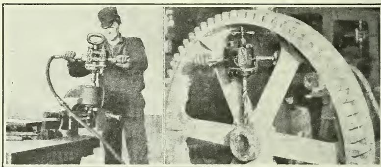
Left—Grinding throttle joints with reversible drill. Right—Piston air drill drilling 1-in. oil hole 3½ in. deep in cast steel gear wheel.
