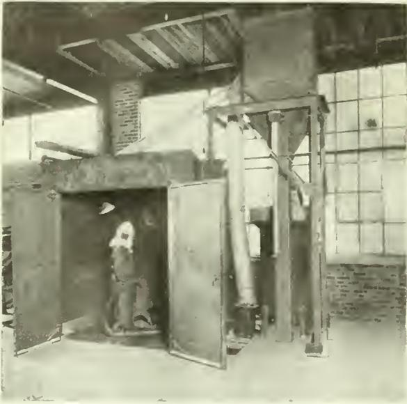
Helmet required only for protecting operator's face from abrasive
