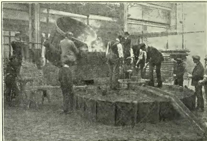
Fig. 4.—Pouring a propeller with manganese bronze.
