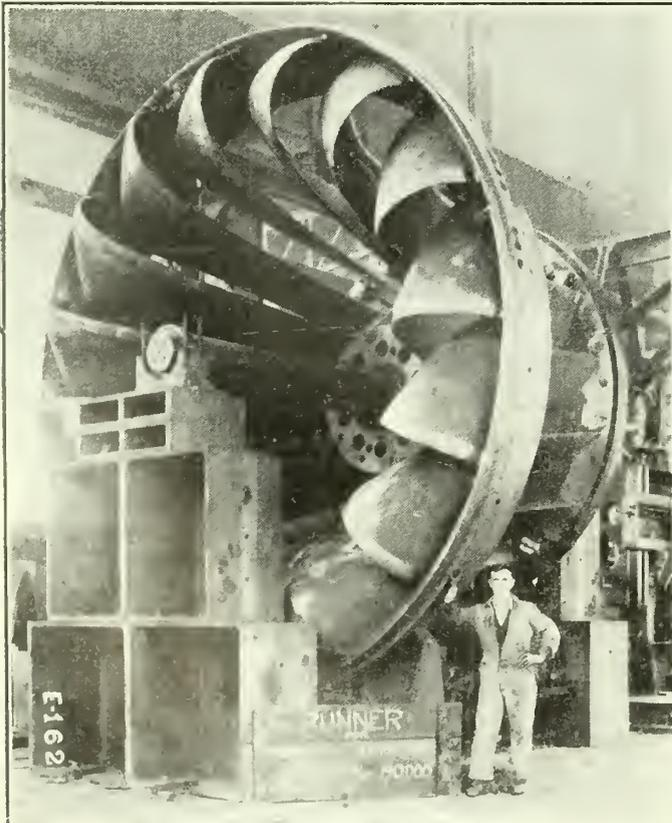
Fig. 5.—Cast Iron Francis Runner, (High Speed Type) of 11,300 H.P., V.S.S.R., turbine for Montreal Light Heat & Power Consolidated. This is the largest runner of this type ever built. Owing to shipping limitations it was necessary to build it in four sections. Total shipping weight, 190,000 pounds.
