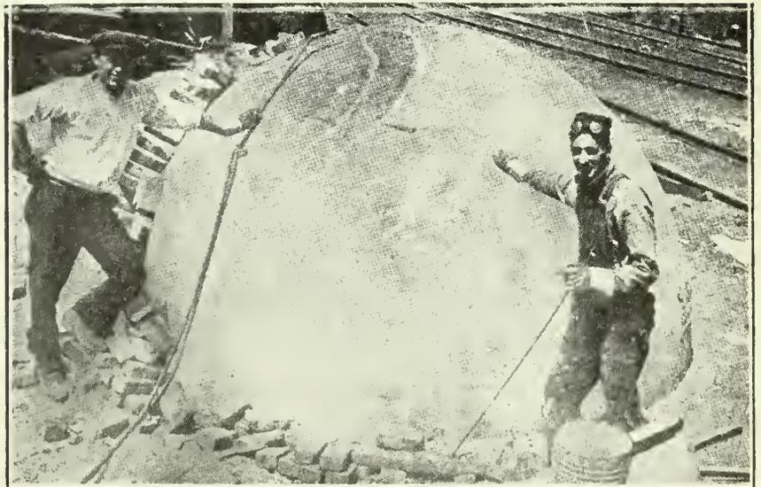
Eight-ton kettle which cracked from continuous expansion and contraction. Ordinarily it would have been scrapped. Oxy acetylene saved it.
