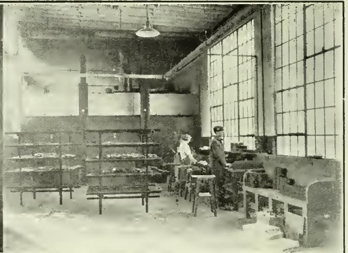
Fig. 5. Core room with rack type ovens in the rear
