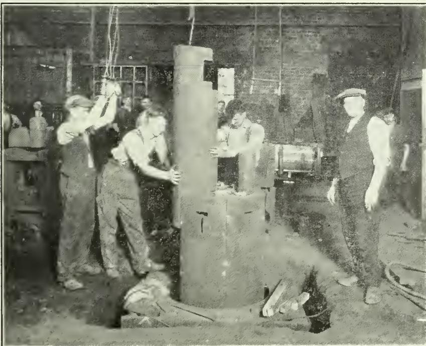
Setting cores in three-ton drum, Darling Bros. Foundry, Montreal.
