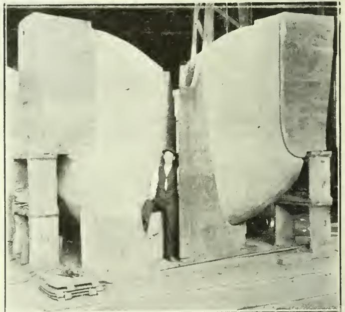
Fig. 6.—Some of the cores for Runner of 11,300 H.P. unit for M.L.H. & P. Cons. Some idea of the amount of core work required may be realized from the fact that each of these cores weighs well over 7 tons and 16 of them are required for one runner.
