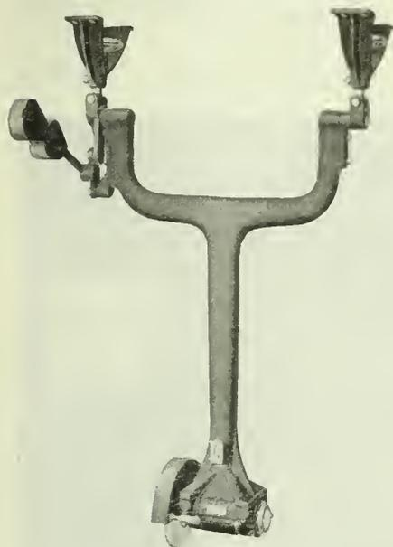
Swinging cut-off saw with motor on the arbor.
