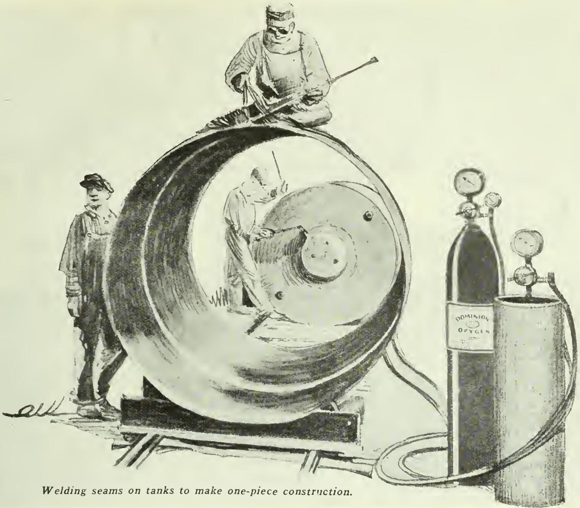
*Welding seams on tanks to make one-piece construction.*
