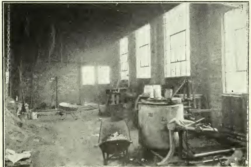
Fig. 2.—General view of interior of foundry, showing melting furnaces.
