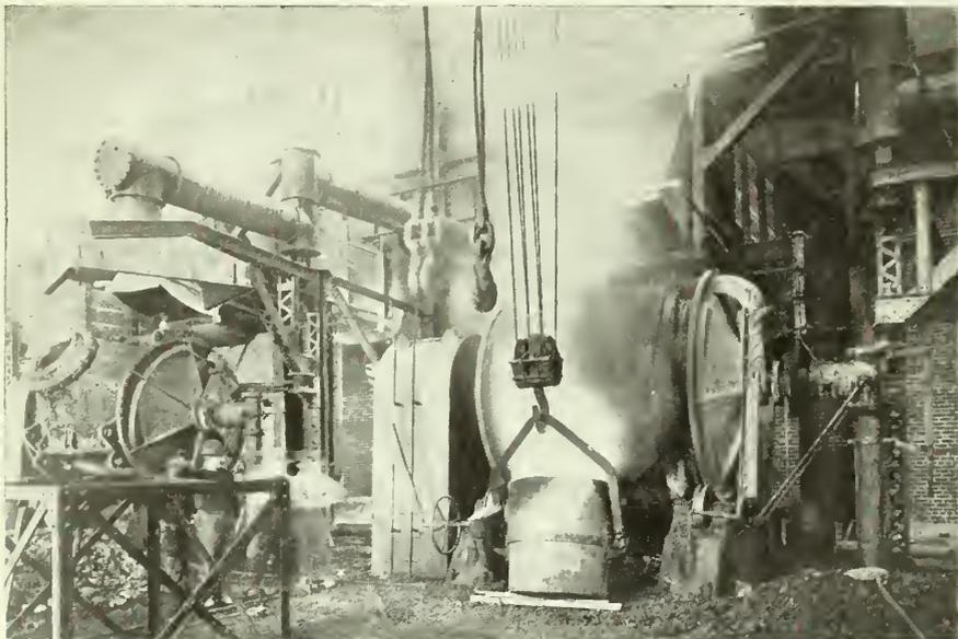
Copper converters at Port Colborne refinery, similar in appearance to those used in steel foundries, but built especially for refining copper.
