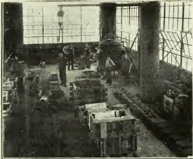
Brass foundry department, Dominion Steel Products Company, Brantford, Ont. Note electric furnace and molds for heavy bronze castings.
