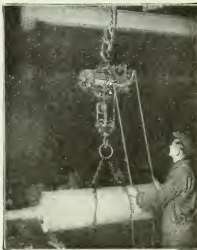
Lifting heavy roll with air hoist.
