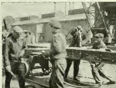
Driving 3/4 in. and 1/2 in. rivets on steel underframes.
