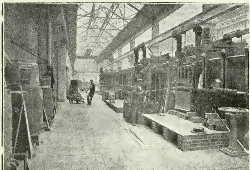
Fig. 3.—Battery of three large reverberatory furnaces.
