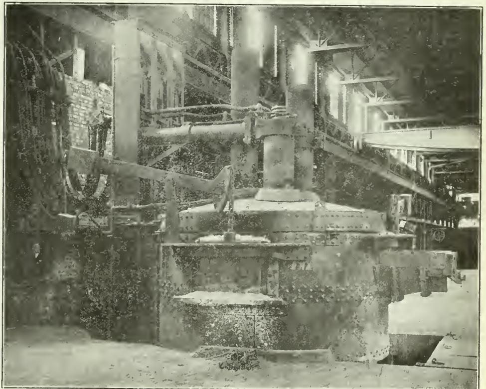
Six-Ton Heroult Type Electric Furnace
