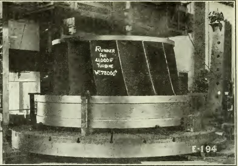
Fig. 4.—Cast Iron Francis Runner, (High Speed Type) of 41,000 H.P., V.S.S.R., turbine for Shawinigan Water & Power Co., Loam casting, total weight, 78,000 lbs.
