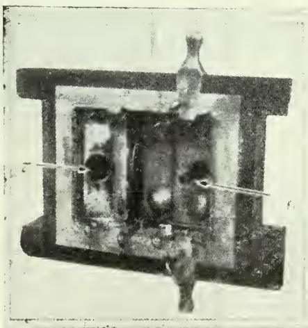
Fig. 7—Core box assembled.
