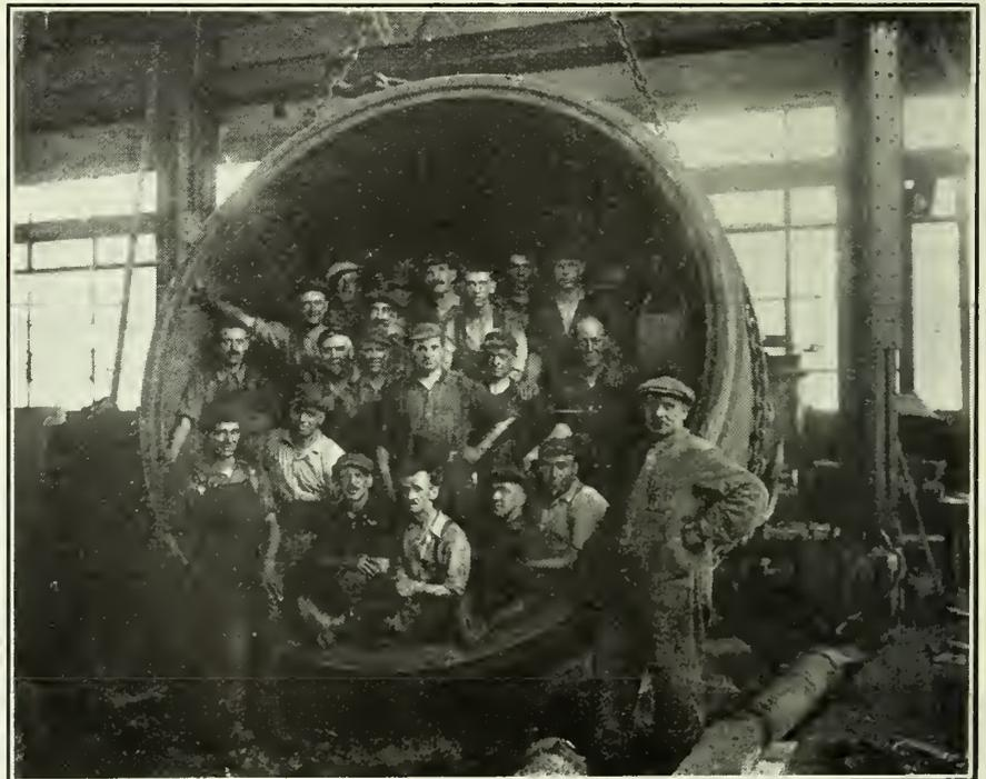
Thirteen-ton caustic kettle cast at the Foundry of the Dominion Steel Products Co., Brantford, Ont.
