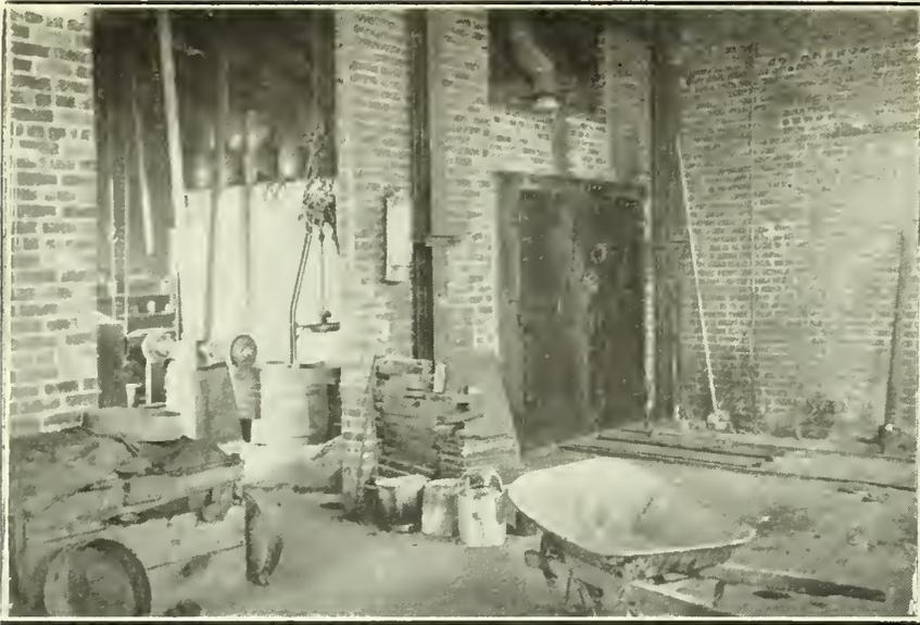
Fig. 3.—Core oven at back of foundry.
