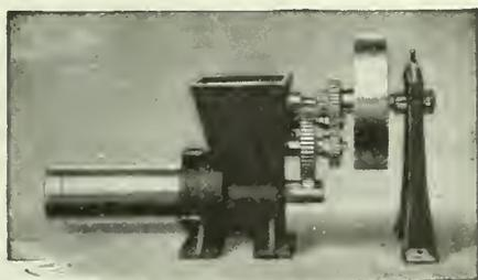
The Wadsworth No. 3 Core Making Machine,  $\frac{3}{8}$  to 7in.
