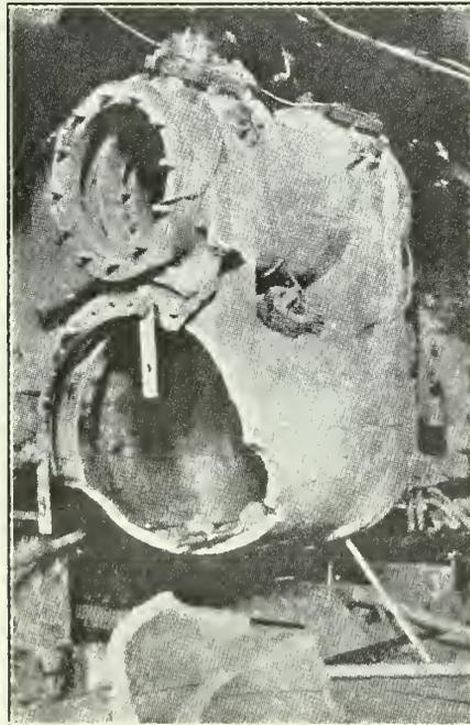
Four stages in the repair of a broken locomotive cylinder, ranging from two inches to four and one-half inches in thickness.
