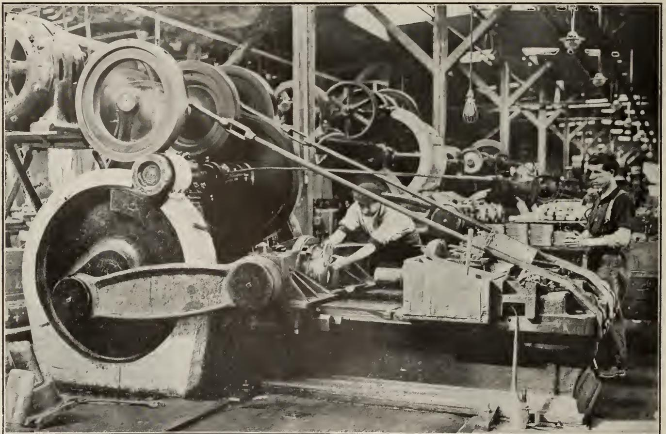
FIG. 22. CUPPING BRASS DISCS IN THE MANUFACTURE OF 4.5 HOWITZER CARTRIDGE CASES ON A "WILLIAMS & WHITE" BULLDOZER.
