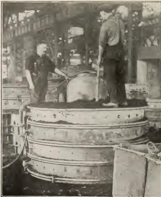
FIG. 11. PREPARING MOLD FOR LARGE STEEL HYDRAULIC CYLINDER.
