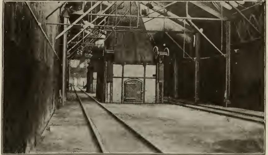
CHARGING FLOOR, SHOWING TOP OF A FURNACE.
