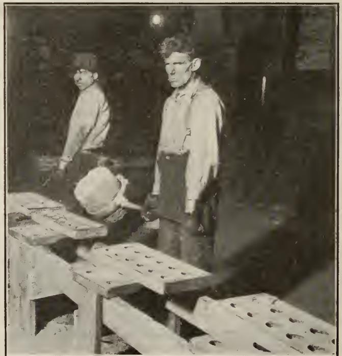
CONTINUOUS POURING OF SLUGS FOR SOCKETS AND CAPS.
