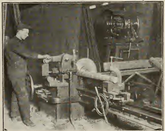
FIG. B—NEWTON SAW SHOWING MOTOR AND STEEL BAR FEED MECHANISM.
