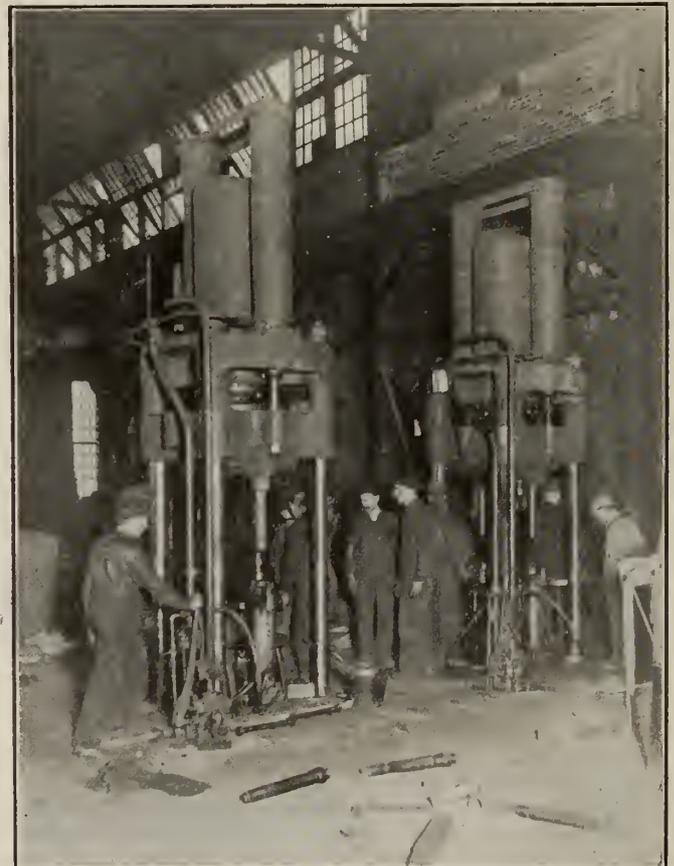
FIG. D—250-TON R. D. WOOD HYDRAULIC PRESSES PERFORMING SECOND AND FINAL OPERATION ON 18-POUNDER SHELL FORGINGS.
