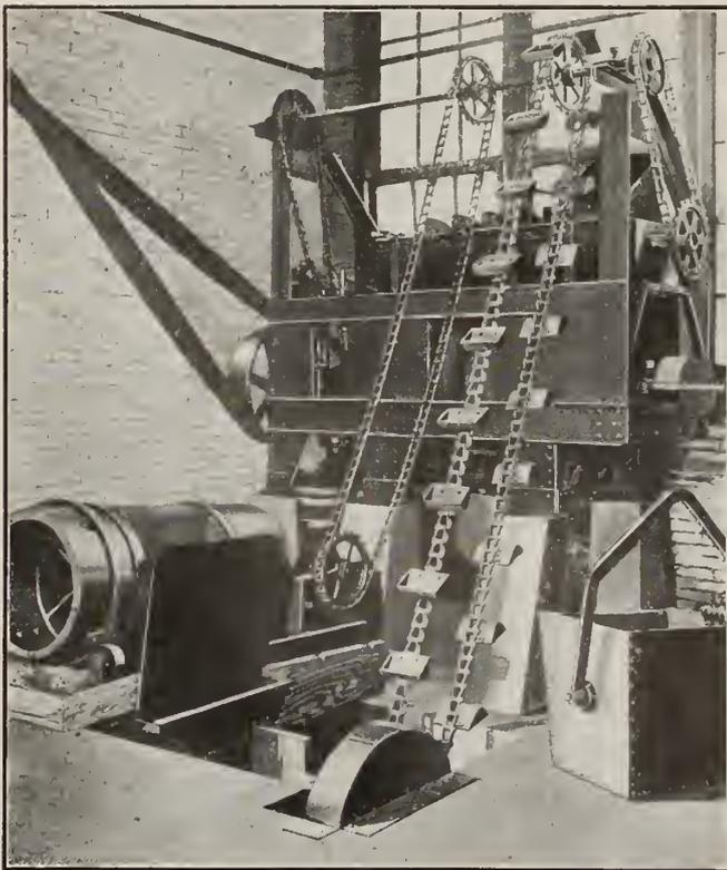
FIG. 1. MIXING, ROLLING AND BONDING MACHINE.
