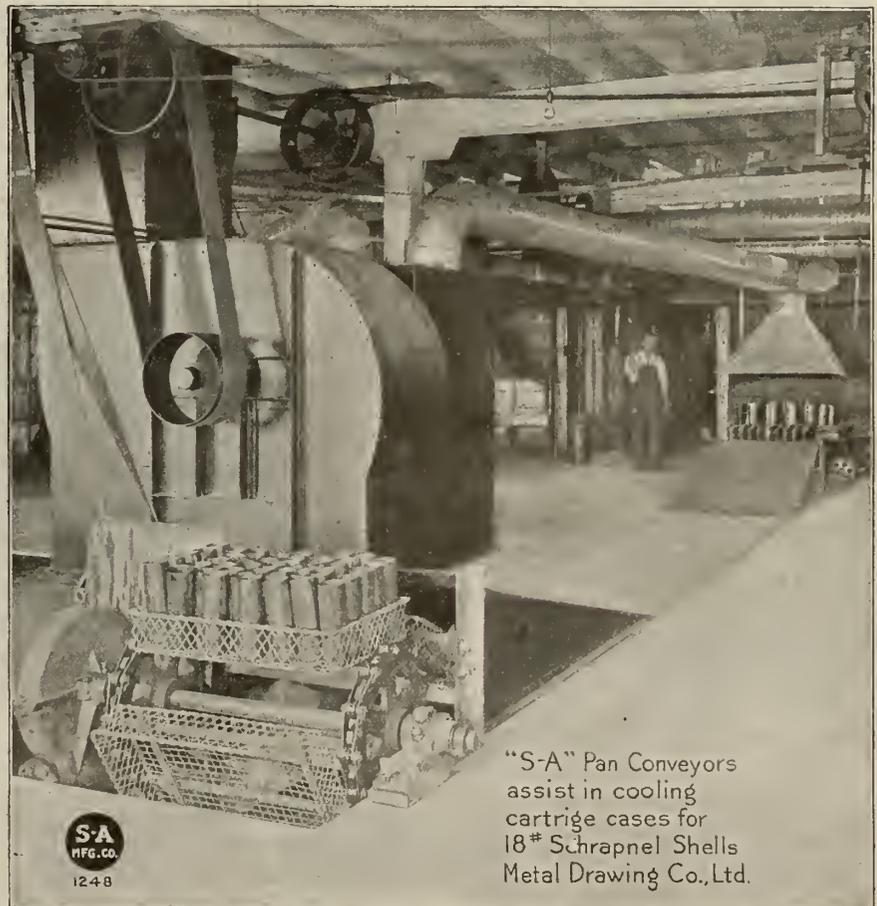
"S-A" Pan Conveyors assist in cooling cartridge cases for 18# Shrapnel Shells Metal Drawing Co., Ltd.
