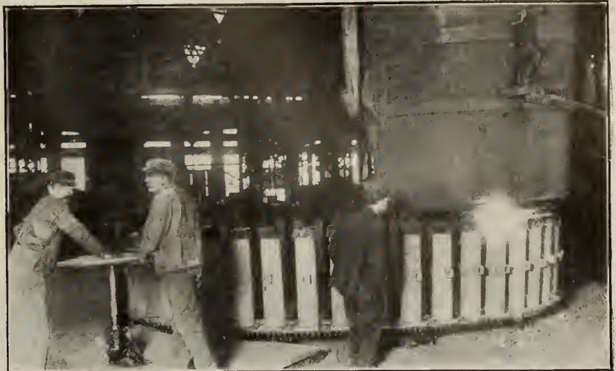
FIG. 5. POURING A BATTERY OF INGOT MOLDS.
