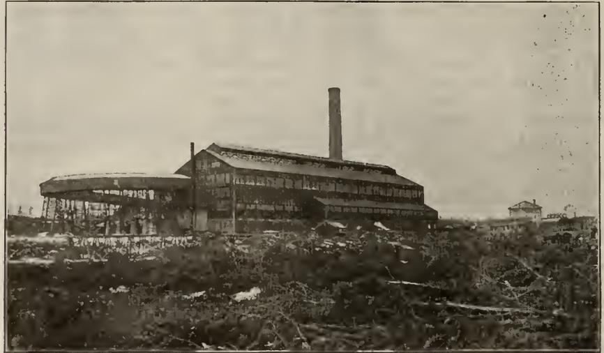
GENERAL VIEW OF THE COMPLETED PLANT AT CONISTON. NOTE THE CURVED LINE OF TRESTLES CARRYING THE TRACKS THAT RUN UNDER THE ORE BINS AND ON THE CHARGING FLOOR LEVEL.
