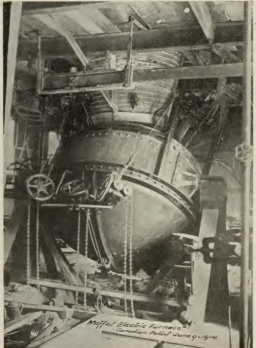
SHOWING ELECTRODE GOVERNING WHEELS AND TOPS OF OSCILLATING HYDRAULIC CYLINDERS WHOSE RAMS TILT THE FURNACE; MOFFAT-IRVING SMELTERS, LTD., TORONTO.
