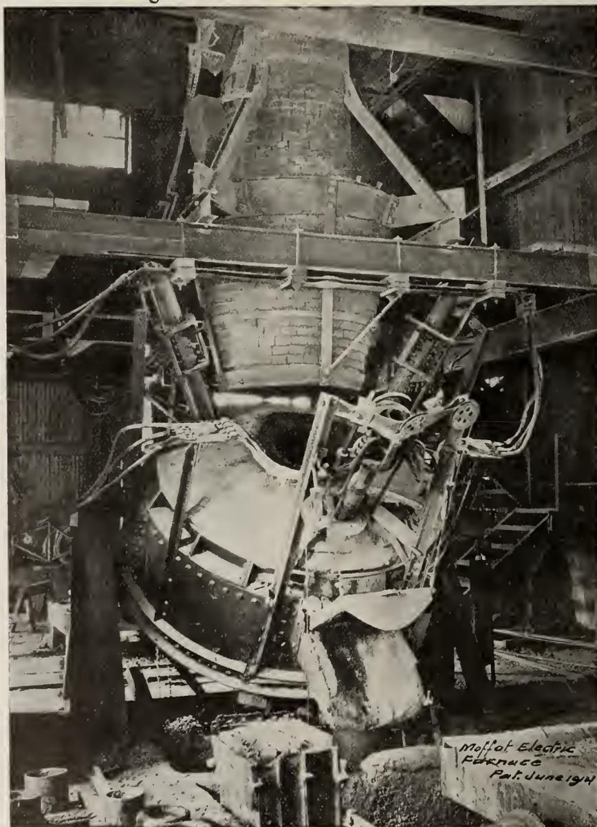
SHOWING POURING POSITION OF ELECTRIC FURNACE, AND VENT THROUGH WHICH ESCAPING GASES ENTER THE SUSPENDED STACK; MOFFAT-IRVING SMELTERS, LTD., TORONTO.
