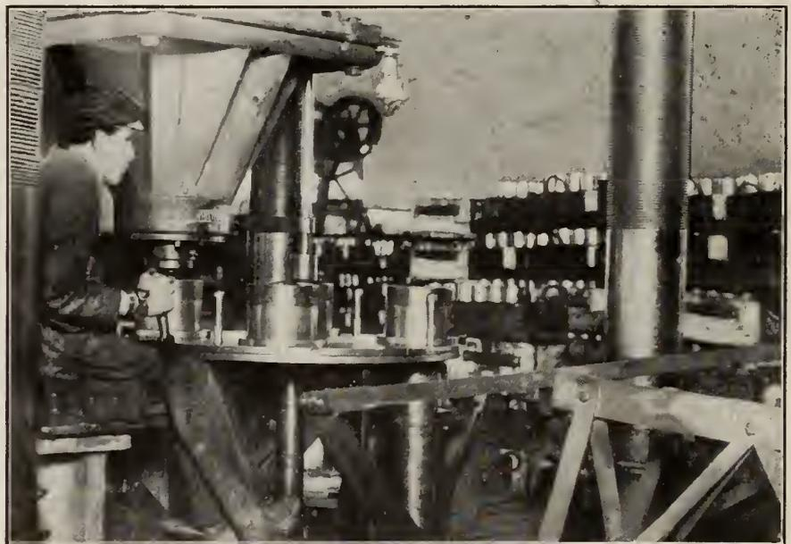
FIG. 8. INDENTING 18-PDR. SHRAPNEL SHELL CARTRIDGE CASES ON A 500-TON HYDRAULIC PRESS.
