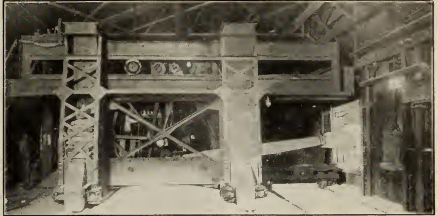
CHARGING MACHINE DEPOSITING MATERIAL IN FURNACE.
