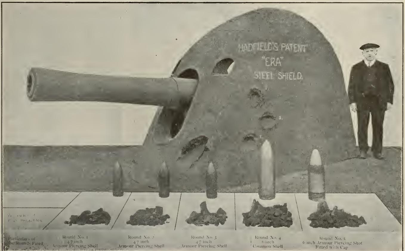
PROJECTILES MADE FROM NICKEL STEEL, MANUFACTURED BY HADFIELD'S STEEL FOUNDRY CO., SHEFFIELD, ENGLAND. MOND NICKEL USED FOR NICKEL STEEL.
