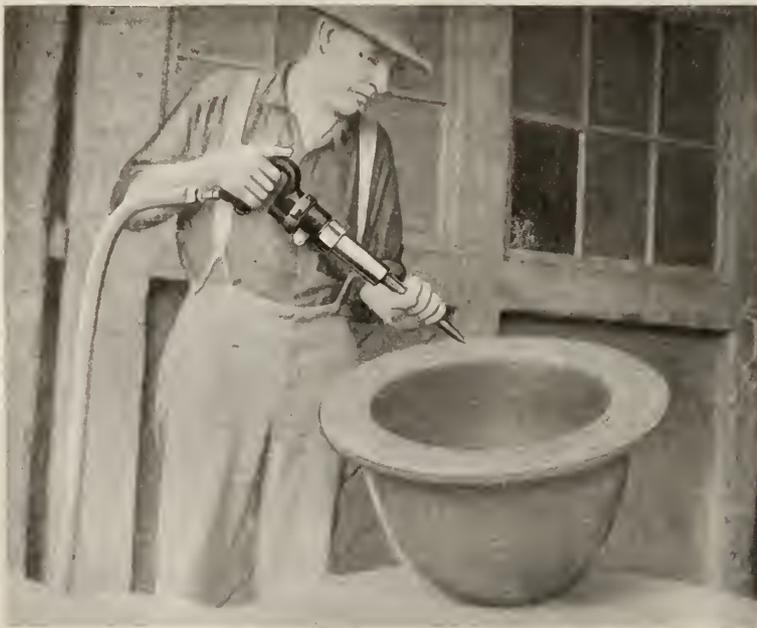
Type L Pistol Grip Pneumatic Hammer Chipping Casting
