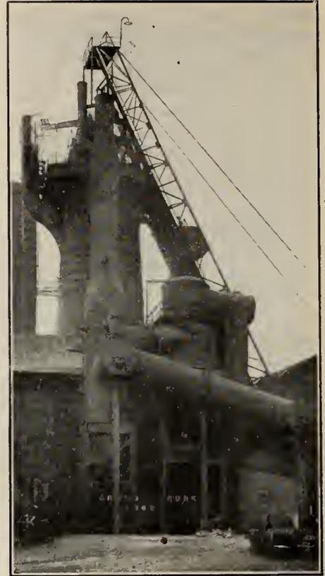
EXTERIOR VIEW OF BLAST FURNACE. SHOWING PIPES FOR CONVEYING WASTE GASES TO STOVES, DUST SEPARATOR IN FOREGROUND.
