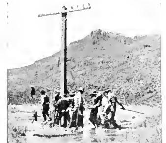
(6) SETTING A POLE IN A SALT SINK.
