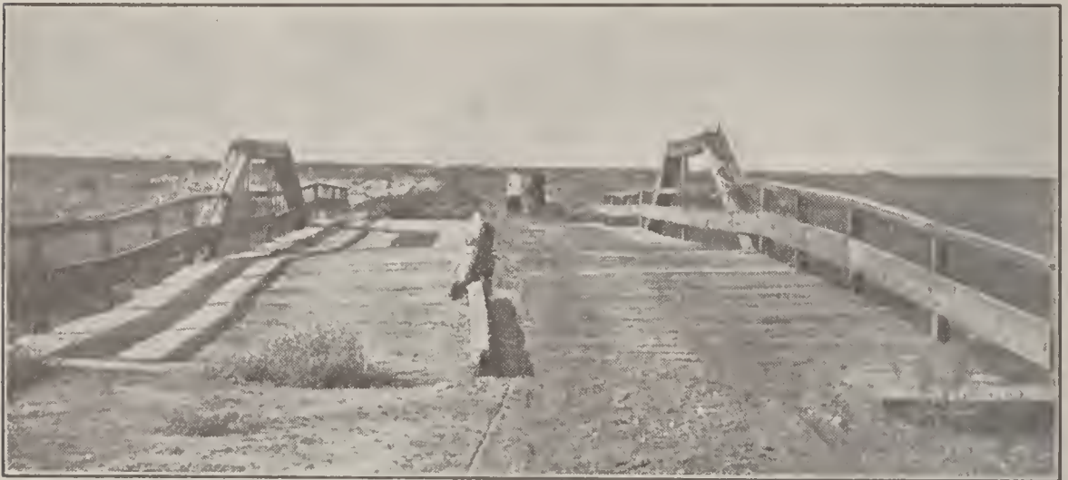
Dangerous Wooden Bridge
