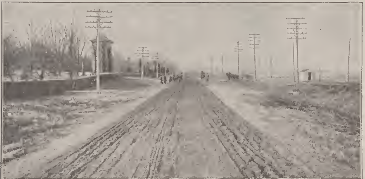
Road before Dragging
