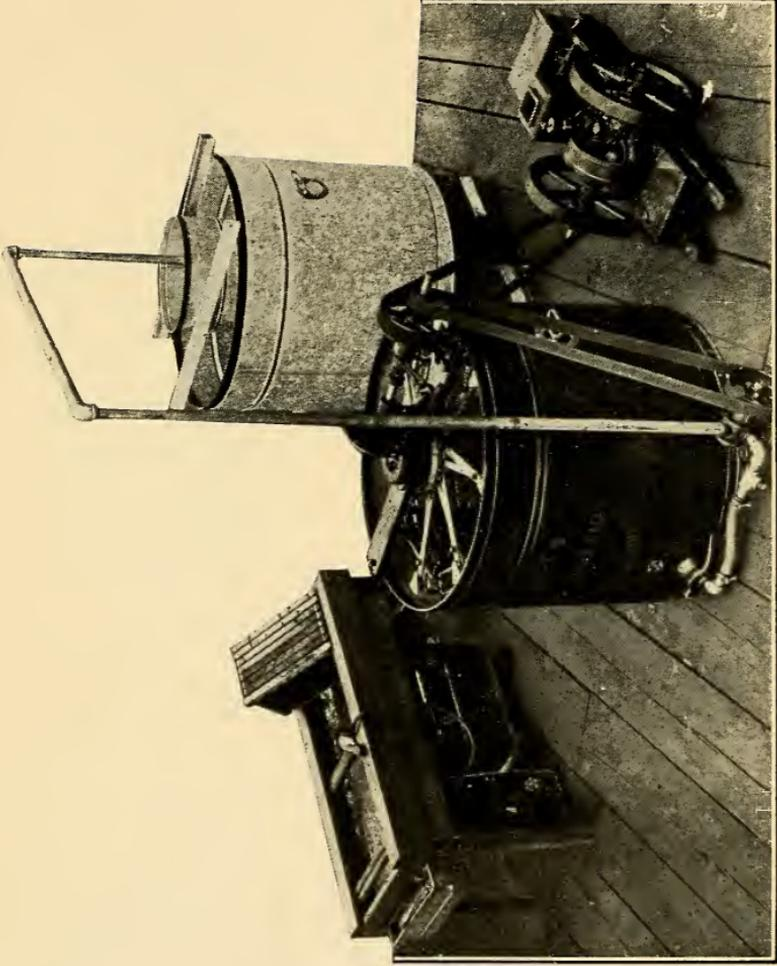
FIG. 122. — Power extracting outfit. Capping melter of large capacity (on left), 8-frame automatic reversible, friction-drive extractor, gasoline engine, honey-pump and strainer.
