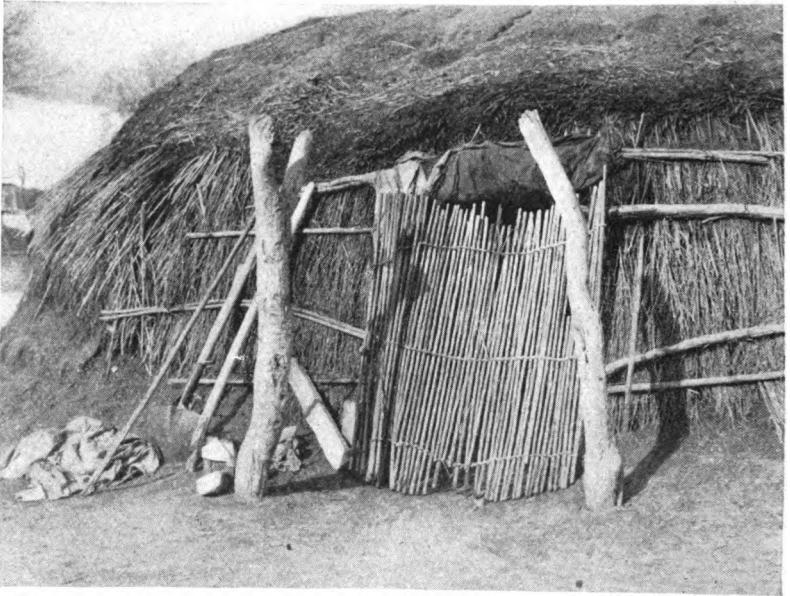
Fig. 3. Oldest Type of House showing a Door constructed with Rows of Wrapped Weaving.
