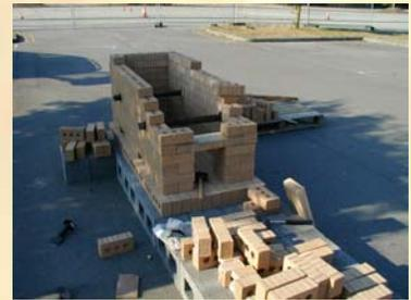
The advantage of the perforated floor is that it positively encourages combustion of the embers over the entire floor thereby giving much better pre heating and consequently even better fuel economy. The 2 inner lines of bricks supporting the floor are also perforated to encourage air cross flow. The outer lines are plain house bricks.
