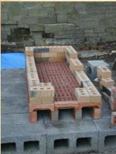
Here you can see the 3 channels which are the primary air entries in this design. The channels extend right through to the other end to provide enough for full combustion (see the notes on proportions at the end of this section). During firing one or more entries can be closed at either end to help vary the atmosphere inside.
