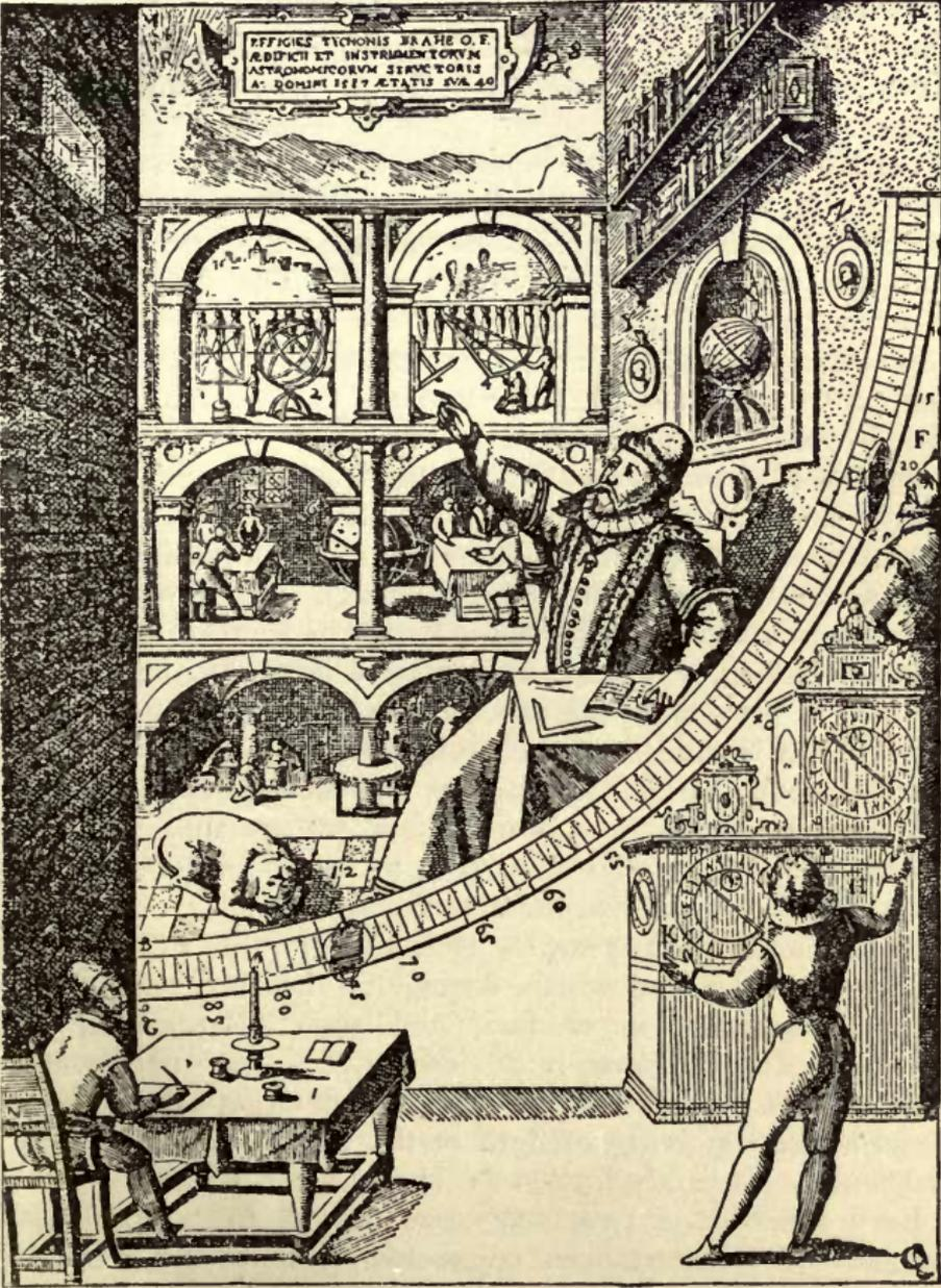
Fig. 277.—Tycho Brahe's Mural Quadrant for measuring Vertical Angles.
