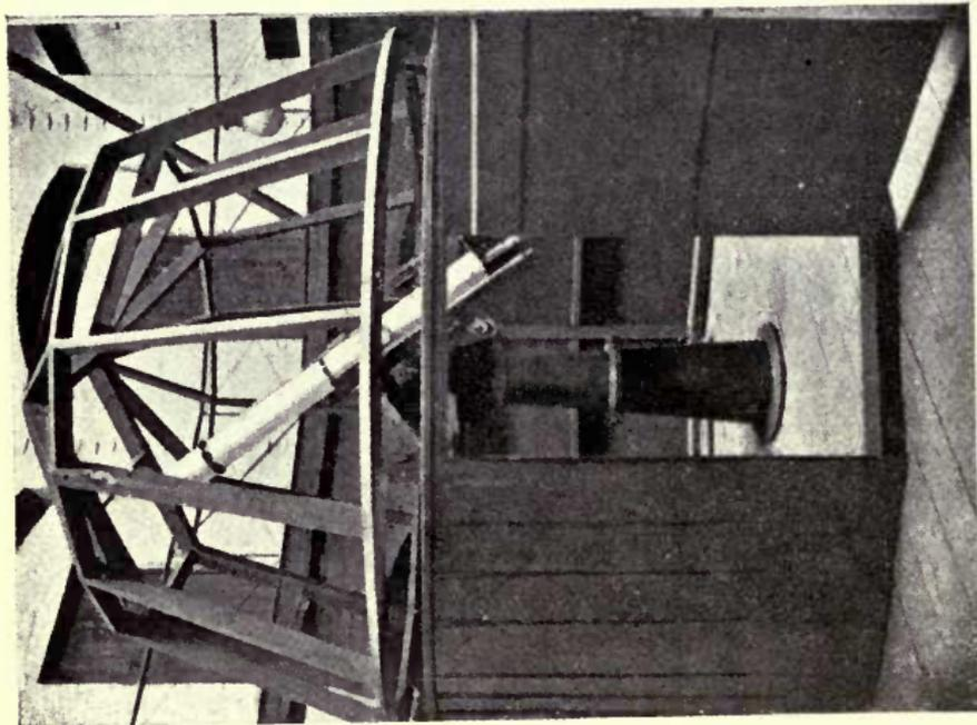
Simple Wooden Framework of Revolving Roof, suitable for covering with either papier mâché or canvas.
