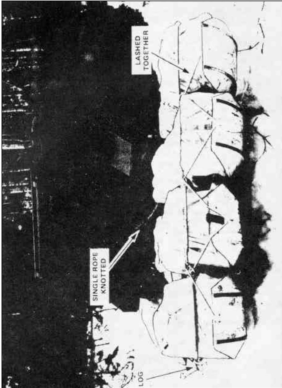
Figure 2-11 The Whippetree Method of Lashing Toboggans Together
