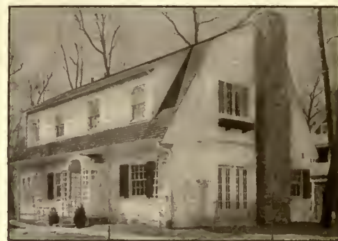
Walls finished with Cabot's Old Virginia White. Roof stained with Cabot's Creosote Stains. F. A. Cooper & Co., Architects, Chicago
