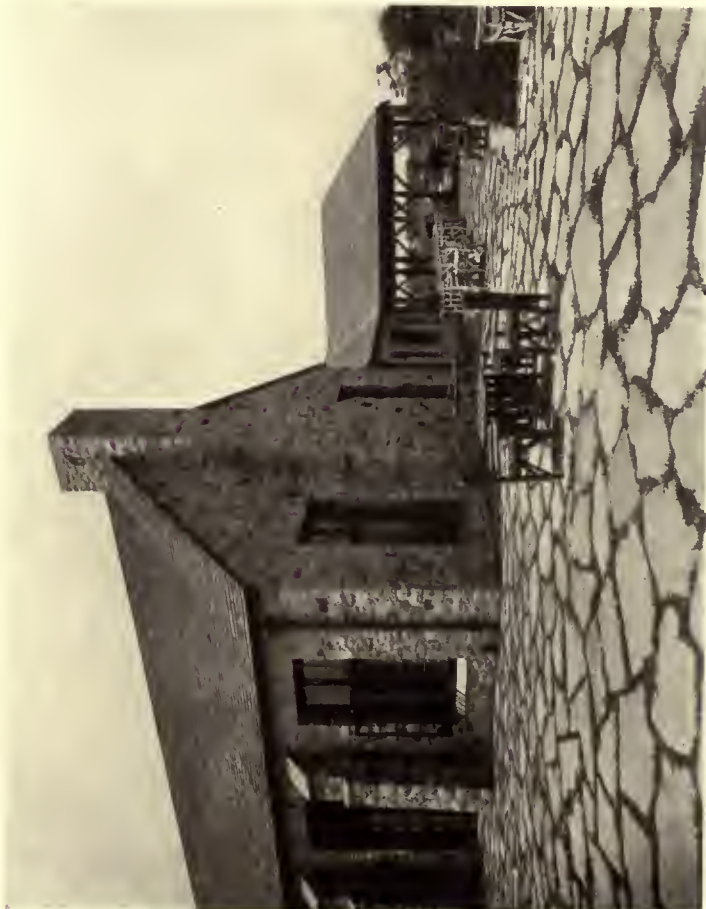
The end of the living-room and entrance porch. The buttresses counteract the thrust of the heavy trusses on the inside of the living-room.
