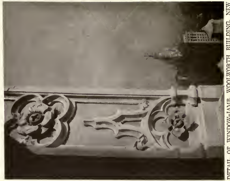
DETAIL OF WINDOW-JAMB, WOOLWORTH BUILDING, NEW YORK. Cass Gilbert, Architect. Polychrome terra-cotta.
