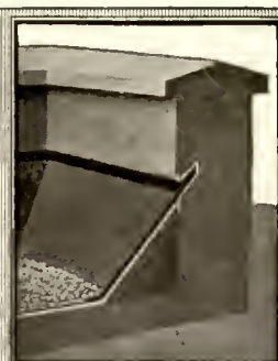
Corner of Roof Showing Concrete Wall with Flashing Form and Flashing Installed
