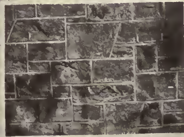
Fig. 6. Square uncoursed Rubble tooled joints
