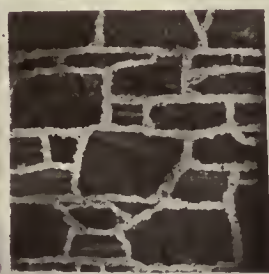
Fig. 2. Rough Rubble - large white, roughly pointed joints
