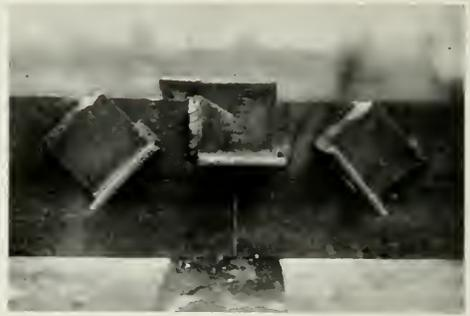
CLIPS FOR CROSS BRACING ON BOTTOM CHORD
