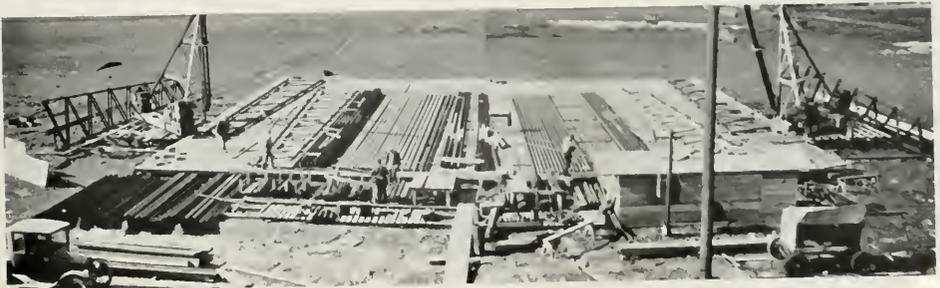
WELDING PLATFORM AND STOCK PILES, A STRUCTURAL ENGINEER ACTING AS FOREMAN. FOUR WELDERS AND TWO LABORERS FABRICATED FIVE TRUSSES PER DAY
