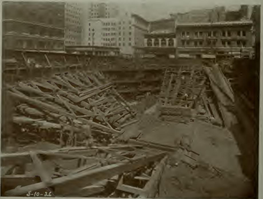
FIG II - STREET WALLS SHORED WITH HEAVY TIMBERS
