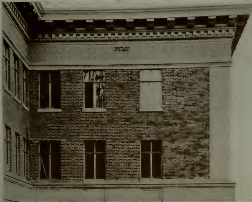
DETAIL OF CORNICE, MADE OF ARMCOR SHEET METAL, BELVEDERE APARTMENTS
