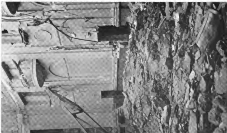
Showing truss T-12 against the 18th Street wall. Note terra cotta above ceiling line upon which truss rested.
