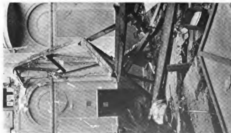
Truss T-12 up against the 18th St. wall. Note ventilating fan at left, which was carried down by collapse of the concrete roof.
