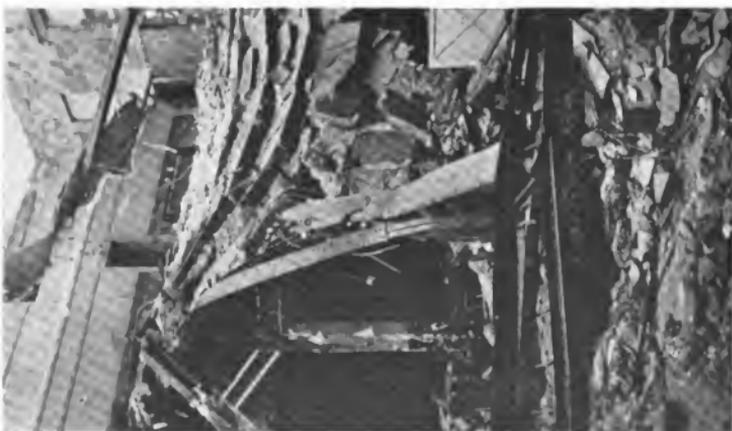
Intersection of Columbia Road wall and south wall. On the left, column C-2 and that part above the joint broken off. Here is an excellent presentation of what came down on the heads of the spectators. The concrete roof is only three inches thick.
