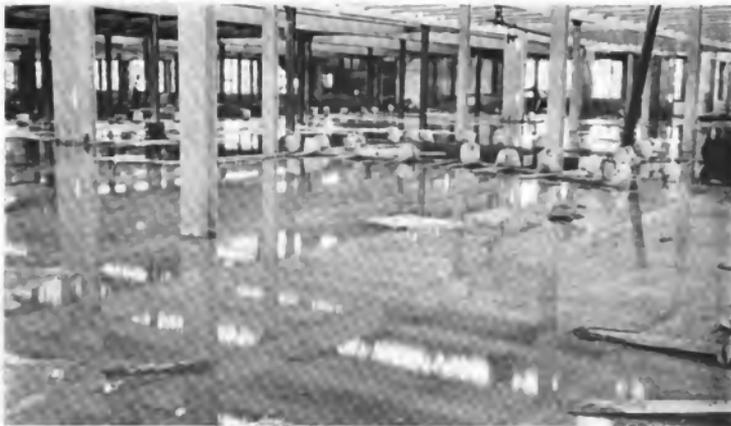
CONCRETE FACTORY FLOOR PROTECTED WHILE HARDENING BY "PONDING"
