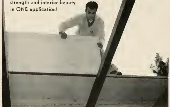
Created for popular exposed beam construction—sturdy roof deck panels made of 1/4" select Western Hemlock Plywood laminated to four layers of 1/2" asphalt-impregnated insulating boards. Panels span 48". Prefinished surface is V-grooved for decorative planked effect. Size: 23" x 96" x 2 1/4". Check Sweet's Architectural File for full details.
