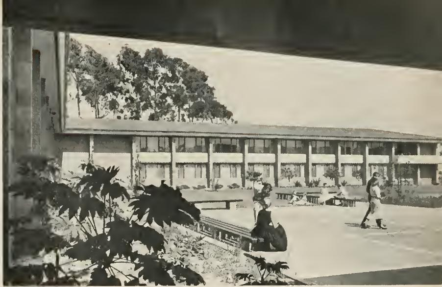
tectural firm of Stone, Mulloy, Marraccini, and Patterson found that by using a steel framework an extra floor could be added. The steel system allows the use of lighter walls and floors, saving from 35 to 50 pounds per square foot of floor area. Smith and Moorehead are the structural engineers. One floor providing approximately 65 additional beds will be completed by
