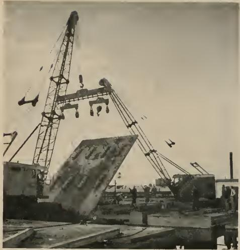
**ABOVE**—one of the thirty-four panels being raised into final construction position.
