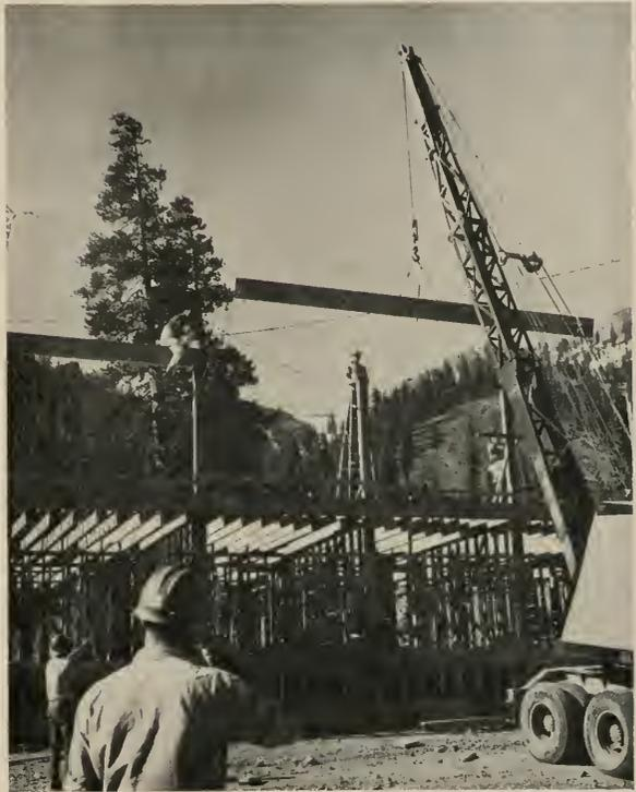
girders, and inclined cable tension members. Each half of the main frame acts independently in somewhat the manner of a guy derrick, with the roof girder functioning as the boom, the column as the mast, and the inclined cables as the guys.
