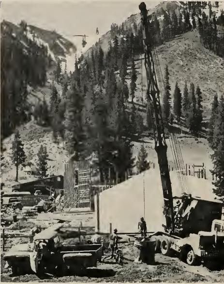
**PRESS BUILDING:** Takes form as workmen prepare to pour concrete wall.
