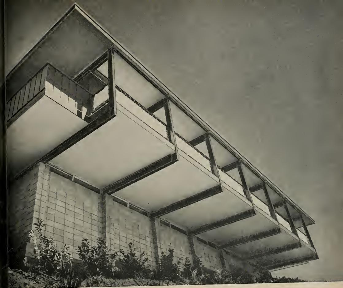
This "L" shaped plan is open and flexible... a blending of inter-related spaces and well-meshed indoor-outdoor living areas. On the uphill, or ground-level, is a large concrete patio with redwood dividers is sun-sheltered under a wide roof overhang, resting on the smoothly tapered tips of the seven major steel supports. The United States Steel shapes in this home are used by steel fabricators and are also available through steel jobbers in your area.
