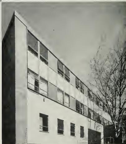
Illustrated: Ariston steel curtain walls with insulated panels.
