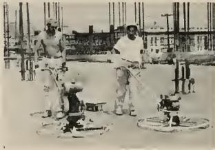
Both models measure only 16 1/2" from blades to engine top (32" former models); new completely enclosed transmission with self contained clutch; planetary gear design, 36 to 1 ratio, direct connection to engine by vertical, centralized, ball bearing mounted shaft; lubricated for life; uses 2 3/4 h.p. engine with 35" ring; rigid cast steel blade supporting arms on both models are surface ground and jig bored. Complete data from Superior Cement Tool Corp., 11616 Wright Road, Lyndwood, California.
