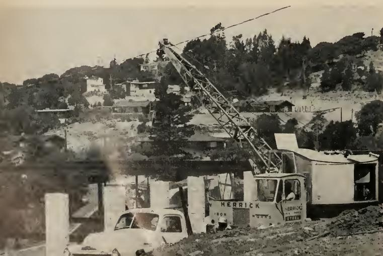
Erecting rigid steel frames; floor joists of steel ribs were landed on concrete piers and wall of 45 degree lot, ceiling joists bolted to seven concrete block pillars; 12 foot by 1-foot shear wall connected to two of the interior frames will provide lateral support.
