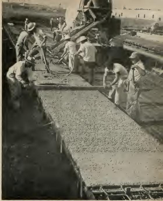
**ABOVE:** As the mixer truck rolls down the line, freshly poured lightweight concrete is vibrated and surface evened-off preparatory to being tamped down and smoothed by finishing crew.
