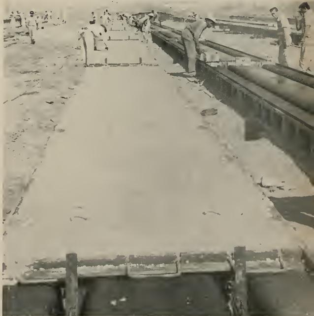
**AT RIGHT:** Finishing crew puts final touches on pre-tensioned, prestressed concrete panels while another 350 ft. casting bed (right) is prepared for pour. Each bed accommodates eight 40-ft. panels, maintaining a 56-ton stress during the 2½ day curing period.
