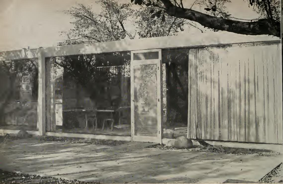
*The steel framing of this building has an 8-inch WF 48-pound member running through the center, supported on a 5 x 5 16-pound column. The front and rear members are 12-inch 10.6-lb. steel channels. These are supported on the 5 x 5 center column and masonry end walls. Intermediate roofing members are 6-inch channels and 8-inch wide flanges.*
