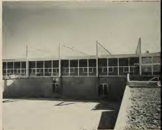
**STEEL FOR VERSATILITY!** Exposed steel trusses solved a problem in the construction of the Green River School's gymnasium . . . and saved about \$30,000 in building costs! Since soil conditions required the building to be founded on pilings, the gym could be recessed half its height into the ground. This unique design allowed for a continuous roof plane. For *your* next project, consider the advantages of steel—United States Steel.
