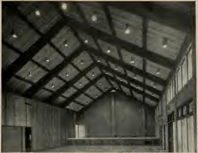
**BELOW:** Shows common entrance for two buildings and 96 foot long roof beams in place — darker plastic panels are colored to contrast with majority in opaque.
