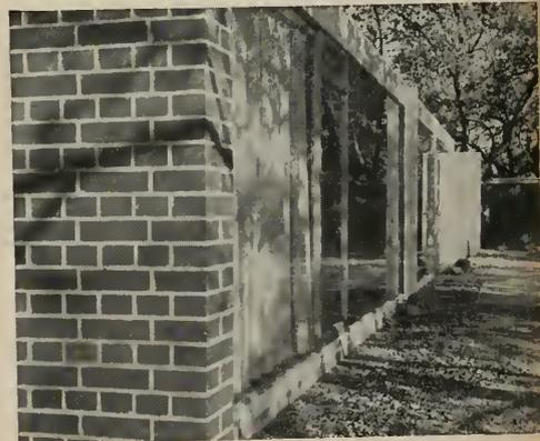
Steel is complementary to any building material. Here the steel frame is set off at either end with English Bond brick bearing walls. The architects favor white painted frames so that shadows will give the structures a "sculptured look."
