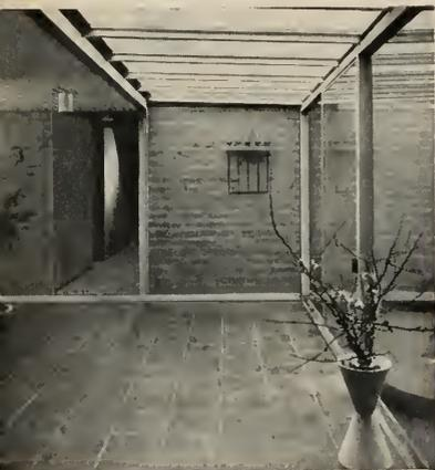
*This Atherton, California, home combines the native qualities of both steel and adobe brick—the strength and versatility of steel and the insulating ability of adobe. The owner has a home that is attractive, permanent, fire and termite resistive, and requires the barest minimum of upkeep. Construction cost, in 1955, was \$11.34 per square foot of living area. The home is arranged in a bi-nuclear design with living and sleeping quarters separated by a glass entry.*
