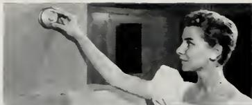
Welcome touch in 1st National's new Portland home is "zone control." Personnel simply set handy wall dials for the blend of air they wish. Hot and cold air streams meet in hi-pressure "mixing boxes"... blend and flow into offices at just the right degree for pleasant air conditioning.
