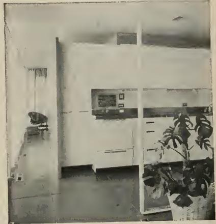
Steel framing leaves interiors open to such possibilities as this plumbing core, a compact gathering of kitchen, laundry, bath and mechanicals. This also serves as an island separating living and bedroom areas. The ceiling is a simple plaster panel suspended from the steel frame.
