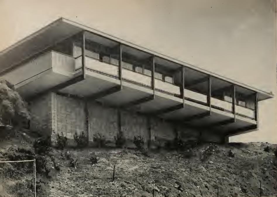
Cantilever extending 11 feet over supporting foundation and wall is made possible by using steel sections. Structure utilizes skeleton of steel ribs which support roof and floor without load bearing walls.
