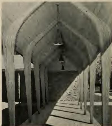
of the decking. Diffused, soft daylight envelops the chancel area from this novel form of lighting and from openings in the chancel roof which are capped on the exterior side by plastic bubbles. The upsweeping beams are unbroken with any lighting fixtures or other ornaments so that the worshipper has a sensation of looking upward and away into undefined distance.
