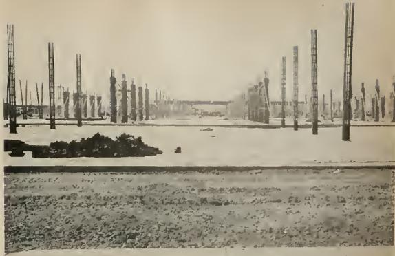
backfilled and compacted, and pouring of the floor slabs began. The slabs are 8 inches thick and, for the most part, are of unreinforced concrete. They were poured in 25 ft. lanes and inserts were left in the slabs for temporary wall braces. In constructing the floors, which are now entirely completed, over 40,000 cubic yards of Class AA concrete was used which met a minimum compressive strength of 3,750 psi at 28 days.
