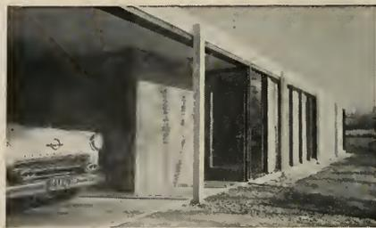
*A distinguishing feature of these Cannon, Smith & Gustavson homes is steel columns riding outside the structure so that loads are carried in shear. The exposed frame presents a clean consistent rhythm that becomes the basic element of the architecture. By introducing some moment into the columns, the architects were able to use lighter steel members.*
