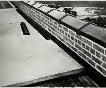
Extending 4 in. up the wall and 4 in. over the deck, they are available in lengths of 40 in. or 47 in., packaged 32 pieces to the carton. Easy to handle and cut, they are protected from attack by termites, dry rot or fungus growth.
