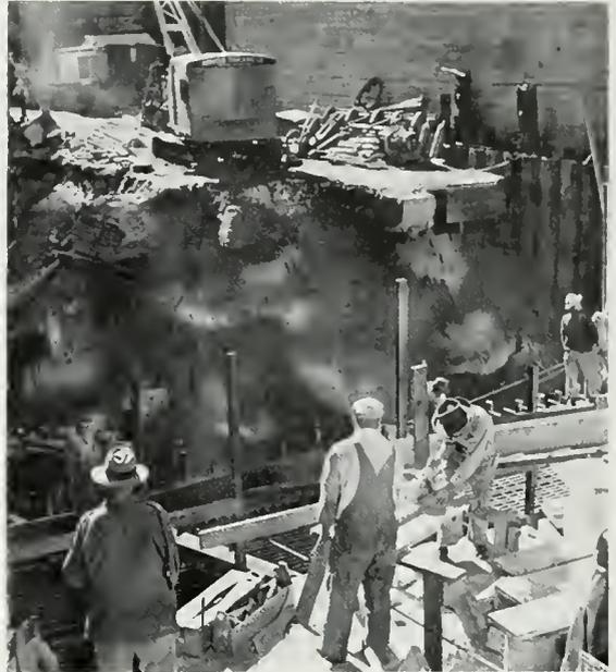
Moke-Ready-Steel mat reinforcing in foreground . . . Foundations of old five story building may be seen in center back around steel sheet piling to left and right.
