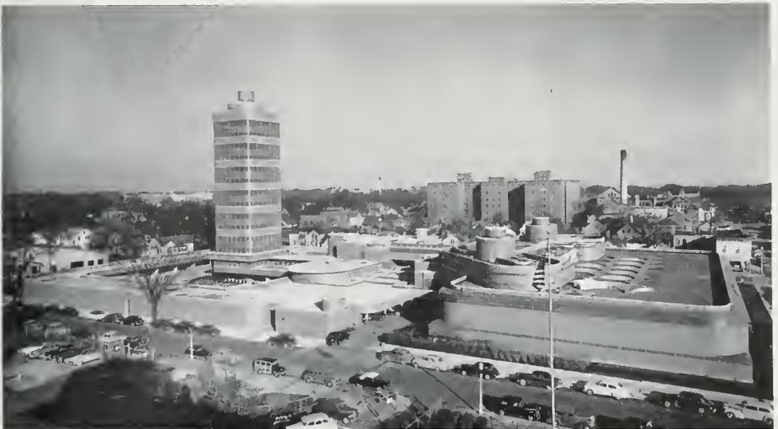
on their particular tasks, and each floor is cantilevered from the central core which is a cluster of circular, reinforced concrete shafts, and rises 156 feet above the ground and is anchored to a concrete foundation which penetrates fifty-four feet into the earth. The main or square floors are cantilevered 21½ feet to each corner, while the circular floors are cantilevered 12½ feet.
