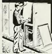
**CLIPPER PANELS** are fitted to tolerances of 1/64"; must be easily removable and replaceable—typifying "custom" care in construction, pride of craftsmanship.
