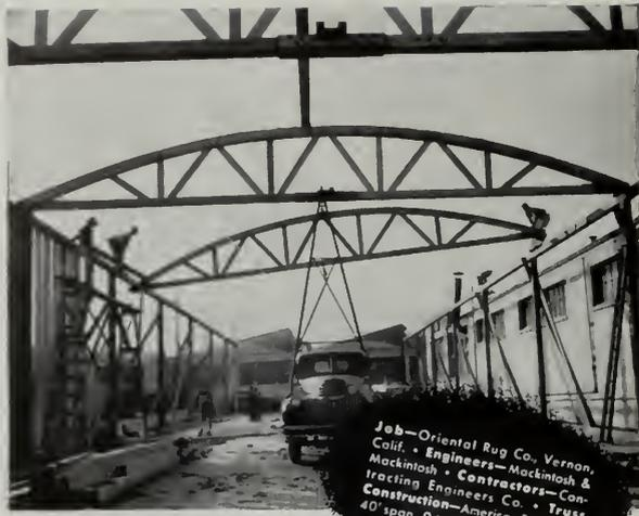
Job—Oriental Rug Co., Vernon, Calif. • Engineers—Mackintosh & Mackintosh • Contractors—Contracting Engineers Co. • Truss Construction—American Bowstring, 40' span, 9 trusses, 17' apart.
