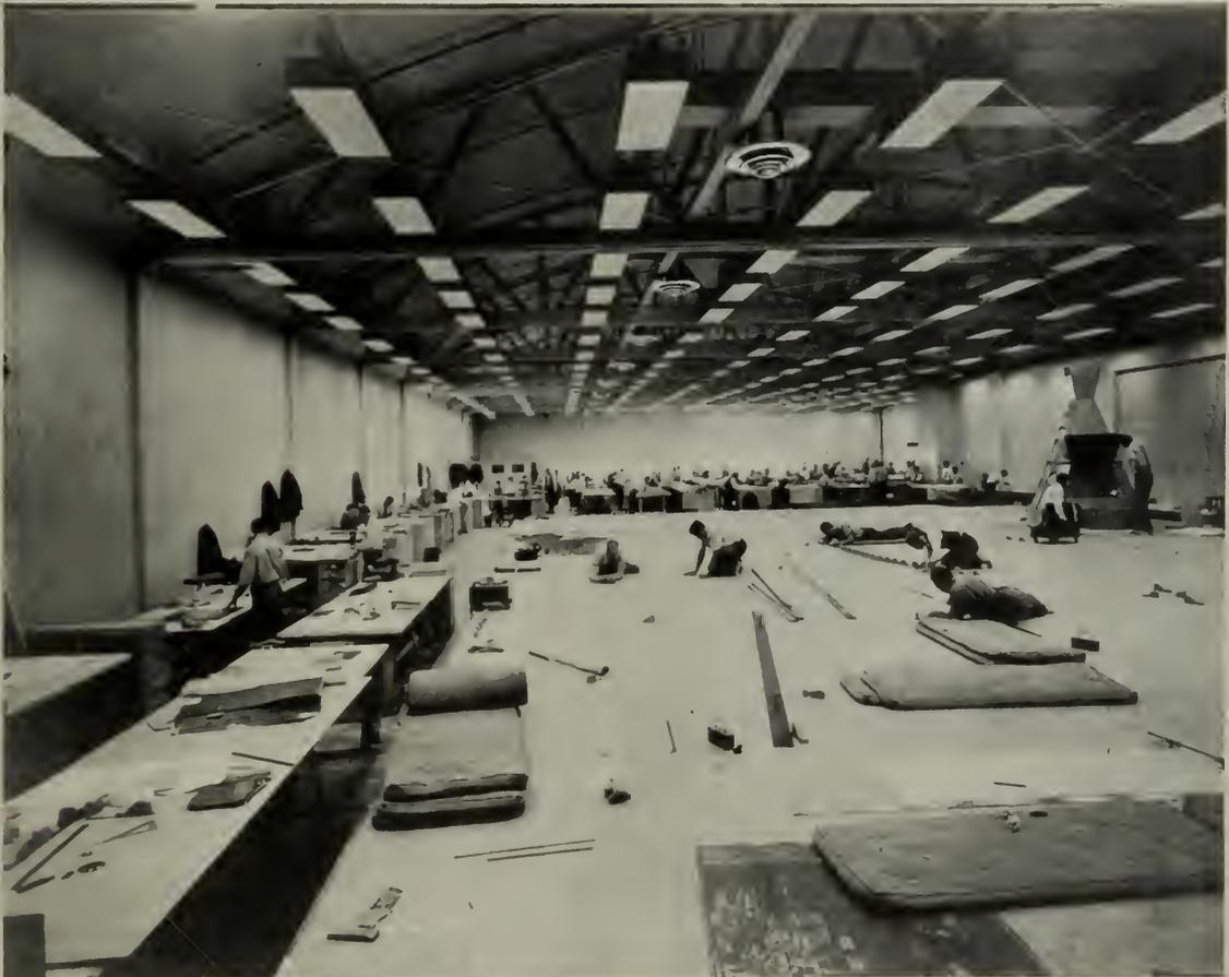
**Air is distributed uniformly and without drafts over the vast floor area of this loft of the Vega Aircraft plant, at Burbank, California. By scientific air-diffusion, Anemostats (on the under-side of the trusses) insure equalization of both temperature and humidity.**
