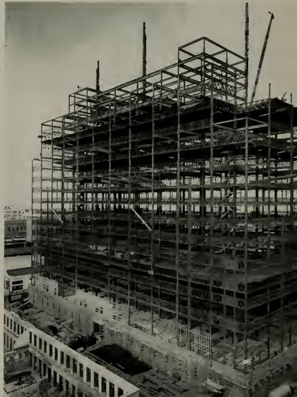
Photo shows steel frame completed. Note girder construction at each floor, a feature of the earthquake design.
