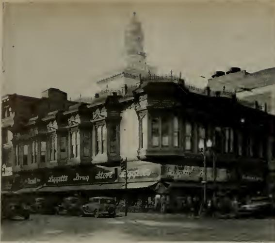
Modernization of the Delger Building called for the removal of bay windows, unadorned roof line and new exterior without making alterations of the structural elements.
