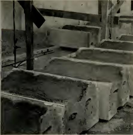
Picture at left illustrates treatment of coping before being set. Several days before installation, each piece was turned hollow side up and filled solid with a very wet, lean mix of grout composed of:
