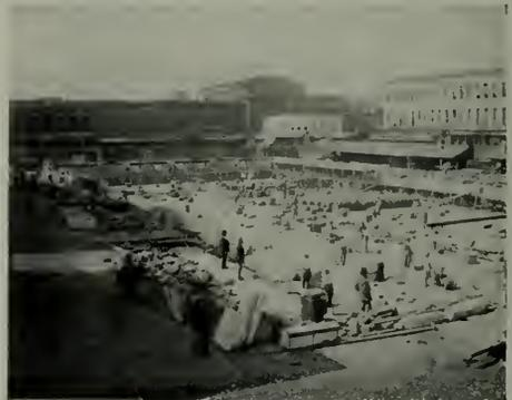
**Photo shows start of construction of old Appraisers Building (1874). Note hand concrete mixers, wheelbarrows and foremen wearing stove-pipe hats to distinguish their official station.**
