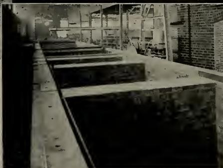
Showing how to construct a tank of Krafftile brick and Nukem jointing compound so as to resist high concentrations of almost any acid and withstand hard usage year after year.
