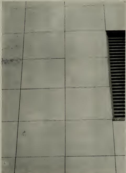
The mortar used in the quarter-inch horizontal and vertical joints (**but not elsewhere**) for setting and pointing the Ceramic Veneer was mixed as follows:
