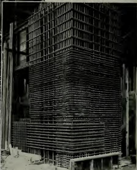
**RIGHT:** Reinforcement at corner. Vertical reinforcing rods ( $1\frac{1}{4}$  inches) are continuous to fourth floor. Each bar is welded to permit continuity.
