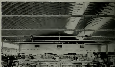
Below: Surv-All Market, 4411-21 West Slauson (Windsor Hills), Los Angeles. Roof supported by five Summerbell Trusses of 120 ft. span . . . Stiles O. Clements, Architect . . . Edwin F. Rudolph, Structural Engineer . . . Robert E. Millsap, Inc., General Contractors.
