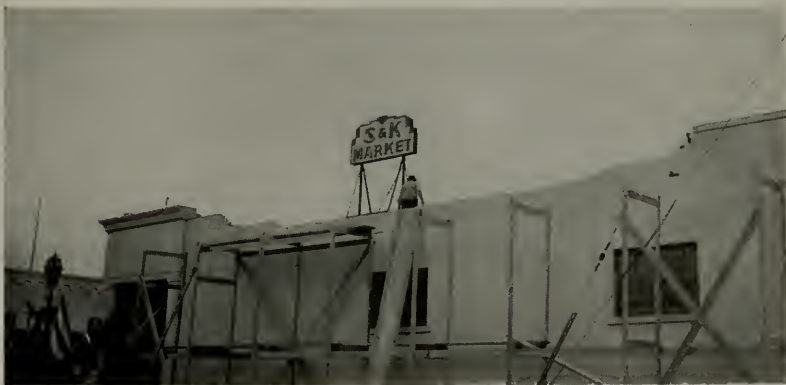
Looking west at S & K Market, State and Ortega Sts., Santa Barbara, California. Top of brick wall on southeast side of building fell.
