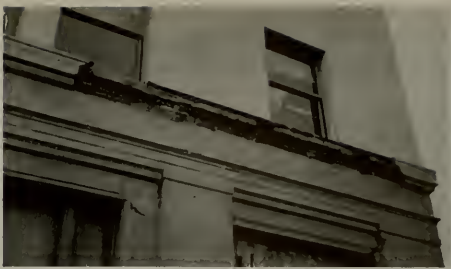
Looking west at Benjamin Franklin Life Building, Santa Barbara, California. Fallen facing from east side of north corner.
