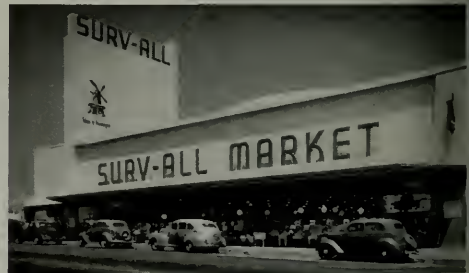
Below: Surv-All Market, 4411-21 West Slauson (Windsor Hills), Los Angeles. Roof supported by five Summerbell Trusses of 120 ft. span . . . Stiles O. Clements, Architect . . . Edwin F. Rudolph, Structural Engineer . . . Robert E. Millsap, Inc., General Contractors.
