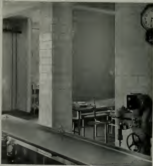
Ceramic Glazed Wall Units (Unsize) are widely used in industrial plants and commercial structures where beauty as well as utility is important. Laid with a nominal \frac{1}{4} -in. joint. Triple-glazed surfaces available in a variety of colors—bright, mat, mottled or clay-coated.
