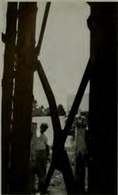
Water Tank, S.P. R.R., Santa Barbara, California. Showing bent diagonal in lower panel of steel tower. About a dozen diagonals were similarly bent.
