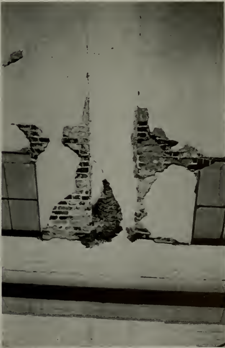
Looking northeast at Bekins Van & Storage Warehouse, Santa Barbara, California. Showing broken brickwork and possible cracked column.
