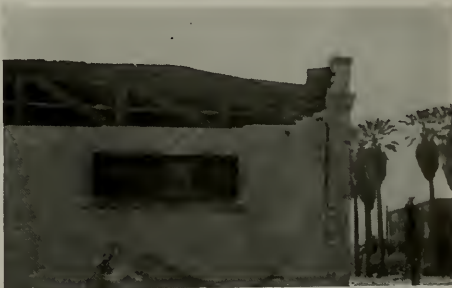
Looking northwest at 618 Linden Ave., Carpinteria, California. Northeast wall tilted out two inches and separated from the southeast wall.
