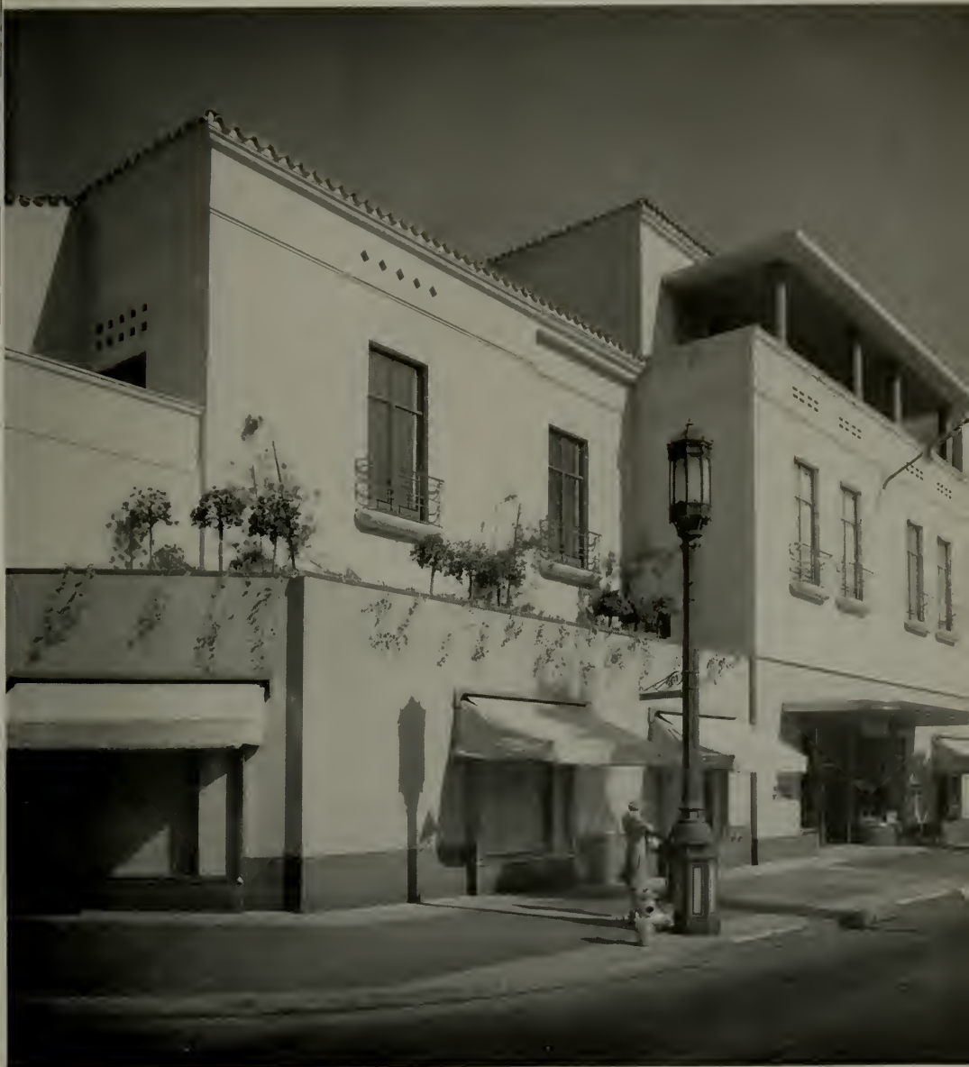
ABOVE—BULLOCK'S WESTWOOD STORE, LOS ANGELES, CALIFORNIA. JOHN AND DONALD B. PARKINSON, ARCHITECTS. THE FINISH IS ADHESION TYPE CERAMIC VENEER, DEEP CORAL, WITH BASE OF DEEP PINK GRANITE.
