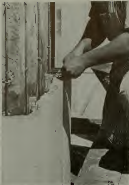
SETTING THE ANCHORED TYPE OF CERAMIC VENEER. PICTURES ABOVE AND BELOW SHOW THE UNIT BEING TIED TO THE RODS INSTALLED IN THE CONCRETE.
