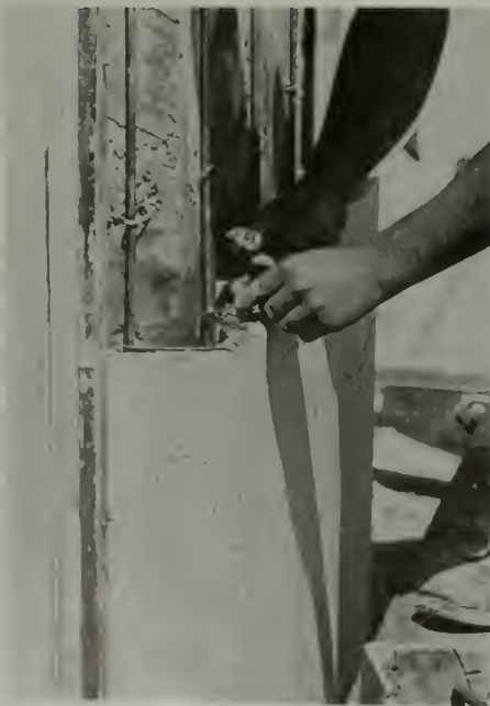
SETTING THE ANCHORED TYPE OF CERAMIC VENEER. PICTURES ABOVE AND BELOW SHOW THE UNIT BEING TIED TO THE RODS INSTALLED IN THE CONCRETE.
