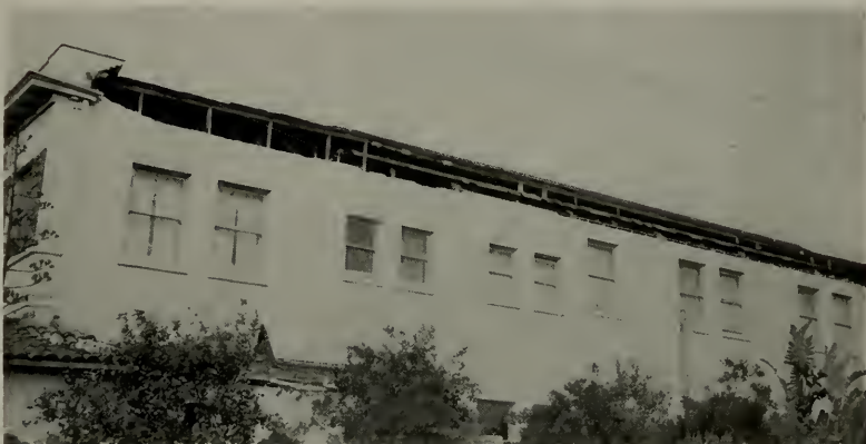
Looking south at Masonic Temple, Carpinteria. Top of northeast brick wall fell.
