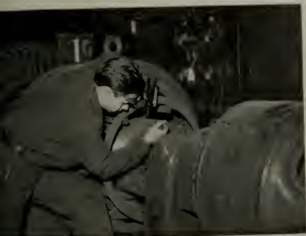
At the Carnegie-Illinois Steel Corporation's mill in Gary, Indiana, an apprentice gets practical experience under-cutting a generator commutator.
