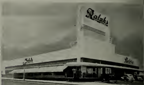
Above and below: Ralphs Market No. 30, West 3d, at Sherbourne, Los Angeles, built like practically all the Ralphs chain, with a Lamella Roof, 100 x 200 feet . . . Stiles O. Clements, Architect . . . Clarence J. Stacy, Structural Engineer . . . S. N. Benjamin, General Contractor.
