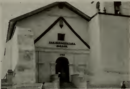
Looking north. Mission at Ventura, California. Brick building with concrete stucco veneer. New cracks in veneer but many cracks are old ones.
