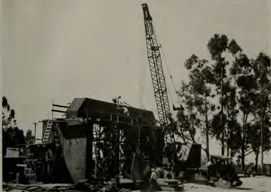
MORE THAN 4900 TONS OF STEEL, ALL ARC WELDED, USED IN CONSTRUCTION OF THIS MONSTROUS STRUCTURE AT UNIVERSITY OF CALIFORNIA, BERKELEY
