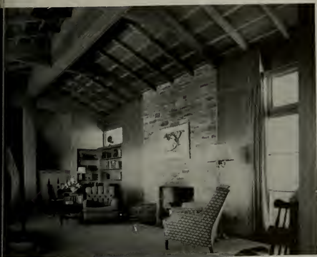
LIVING ROOM is paneled in Philippine mahogany with redwood and pine ceiling. Note gusset roof construction in place of customary trusses.
