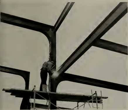
Welding steel frame of apprentice building
