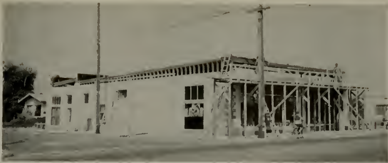
Looking east at Drug Store building, Carpinteria, California. 1-story concrete block building. Front and side walls fell into street.
