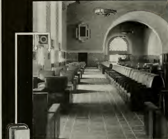
The architects for the Union Passenger Terminal, Los Angeles, have protected the Johnson room thermostats, in the main waiting room, by designing special protective housings, so that there will be no interference with their important functions.
