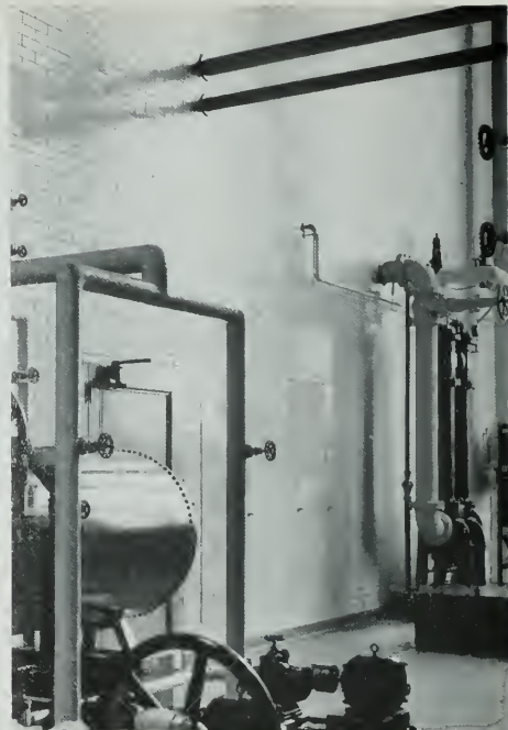
TWO VIEWS OF BOILER ROOM, ASSEMBLY PLANT OF FORD MOTOR COMPANY, SEATTLE, WASHINGTON, SHOWING KRAFTILE ENAMEL BRICK INSTALLATION
