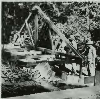
Standard 32-foot span timber roof truss for warehouse at Forest Service Experimental Range Station, Strawberry, Calif. 2\frac{1}{2} " TECO split ring connectors at all joints.
