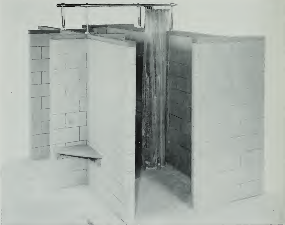
Shower and dressing compartment partitions for Girls' High School Gymnasium, Vallejo, California, as constructed at Kraftile Company plant for tests of structure and seismic resistance. Three-cornered wooden seat in one of the dressing compartments is in Wall B, as tested. At right, is Wall A, as designated in sketch. Hardware for doors, at each end of unit, and plumbing, including shower head, were omitted in test set-up.
