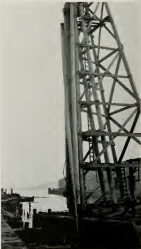
Photograph shows removal of piles at Pier 19, San Francisco waterfront, October 26, 1937, to make room for new pier. Note excellent condition of piles after service of 23 years. The piles were originally treated with West Coast Wood Preserving Company's creosote, represented in San Francisco by J. H. Baxter Company.
