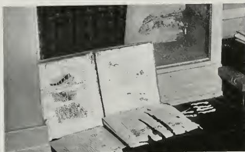
Fig. 3—The hazard in building an unprotected structure near a termite colony is very real. Within four months after his home was completed this damage was done.
