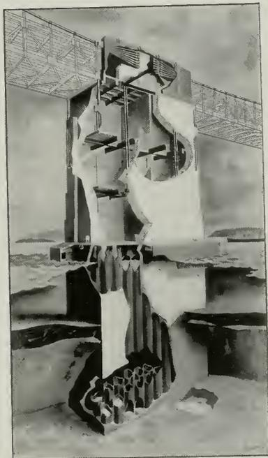
the injury to ships. The fender is fitted with timber to withstand the impact of small boats.
