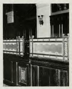
Bank counter screens of tapestry (obscure) plate glass, sandblasted with one deep cut.
