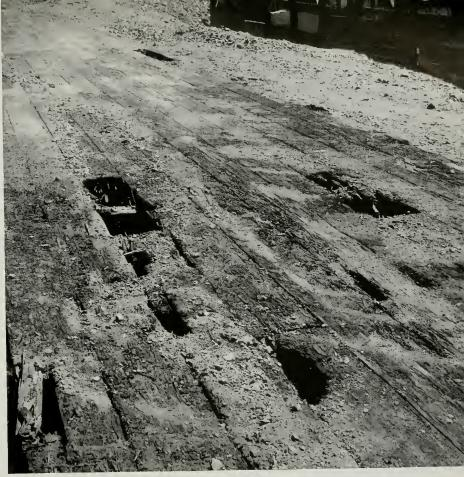
FIG. 2—VIEW SHOWING CONDITION OF REDWOOD COVER PLANKS, ISLAIS CREEK SEWER, AFTER FILL HAD BEEN REMOVED
