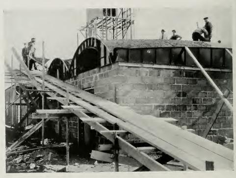
EXTERIOR VIEW OF REAR OR LAKE SIDE. NOTE STEEL GABLE FORMS. DOUBLE CURVE IS PLAINLY VISIBLE
