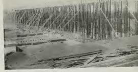
WALL FRAME ERECTED READY TO RECEIVE FLOOR JOISTS
