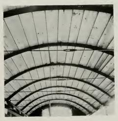
UNDERSIDE OF FORMS, SHOWING CURVED STEEL RIBS RESTING ON CURVED BEAMS—SHEATHING BOARDS—AND PLYWOOD SHEETS.
