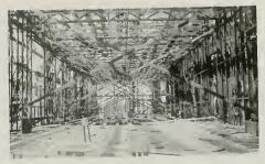
EARTHQUAKE BRACING IN ALL NON-BEARING TRANSVERSE PARTITIONS
