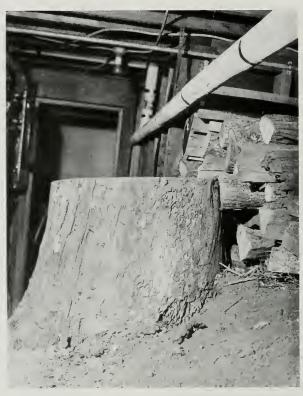
Fig. 21—Tree stump left under an apartment building. The stump is infested with subterranean termites. The firewood piled in contact with the ground and stump may also provide an avenue of attack.
