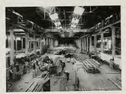
WALL PANELS BEING FABRICATED IN SHOP
