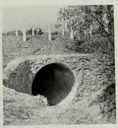
FULL-ROUND, 105-INCH DIAMETER DRAINAGE Way made of heavy corrugated plates bolted together in the field. The rubble headwall of native stone presents a pleasing appearance.
