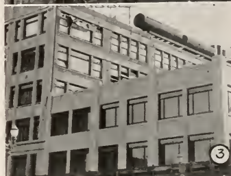
The three views above show a large four-story building in which a 3-story wing has been reconstructed with reinforced concrete exterior walls and plaster finish, applied to blend in color and appearance with the exterior facing of the main building. (1) Walls being cast in the forms. (2) Removal of form. (3) Completed exterior.
