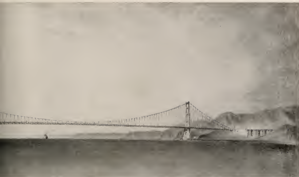
TH A SINGLE CLEAR SPAN OF 4200 FEET, LONGEST SPAN IN THE WORLD
