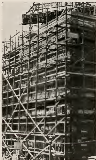
A large skeleton frame building prepared for application of reinforced gunite facing to the masonry, showing diagonal bracing welded to the steel frame.
