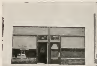
Almost any desired effect may be produced in placing concrete building fronts, a great variety of mold and form selections being available. The upper view shows a surface produced by form liners, while the lower picture shows effect obtained by the surfacing of the wood forms.
