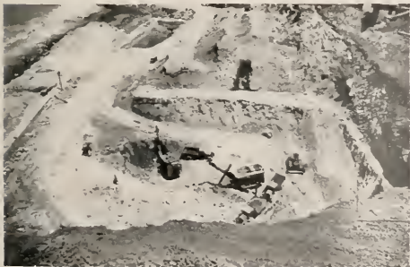
EXCAVATING FOR CABLE ANCHORAGE SAN FRANCISCO SIDE
