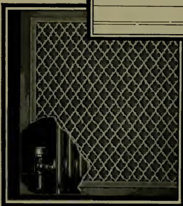
At left: A cabinet hides the "standing radiator" with Johnson valve on steam supply.
