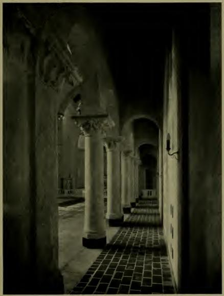
Columns, caps, etc., poured monolithic in place
