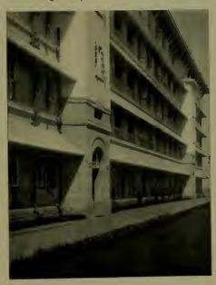
A CLOSE-UP OF THE "CHUJJAS", OR COR-NICE, WHICH HELP TO MAKE LIFE MORE COMFORTABLE IN BOMBAY. THESE ARE CAST IN CONCRETE, WITH THE REST OF THE STRUCTURE
