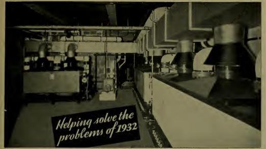
The two automatic gas-fired steam boilers, at right, furnish efficient service to approximately 8,000 square feet of cast iroo radiatioo. The third automatic gas-fired holier, at left, is connected to two 2,000-galloo tanks, equipped with steam coils for hot water supply.
