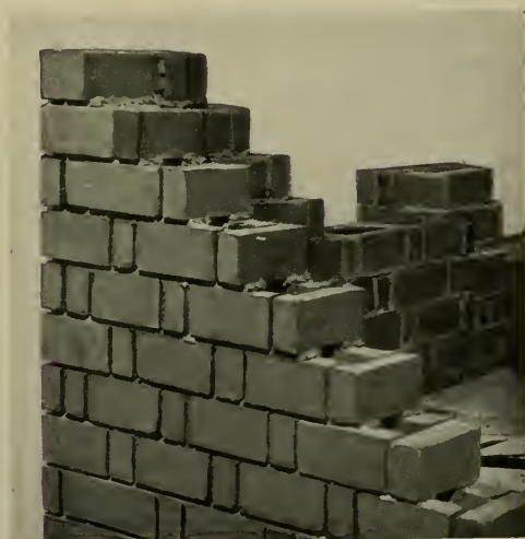
TYPE OF BOULDER CITY HOUSE CONSTRUCTION EIGHT INCH WALLS WITH HOLLOW SPACE
