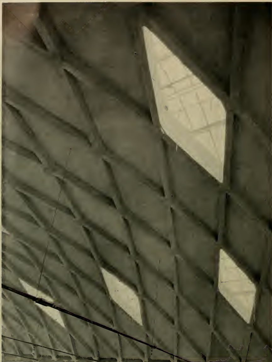
CLOSE UP OF ROOF CONSTRUCTION, COCO COLA WAREHOUSE STEEL MEMBERS FIREPROOFED WITH TWO INCHES OF CONCRETE
