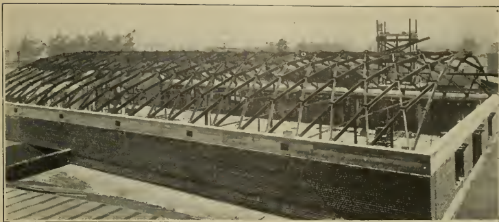
STEEL LAMELLA ROOF, COCO COLA PLANT, LOS ANGELES. THIS ROOF HAS A 70-FOOT SPAN
