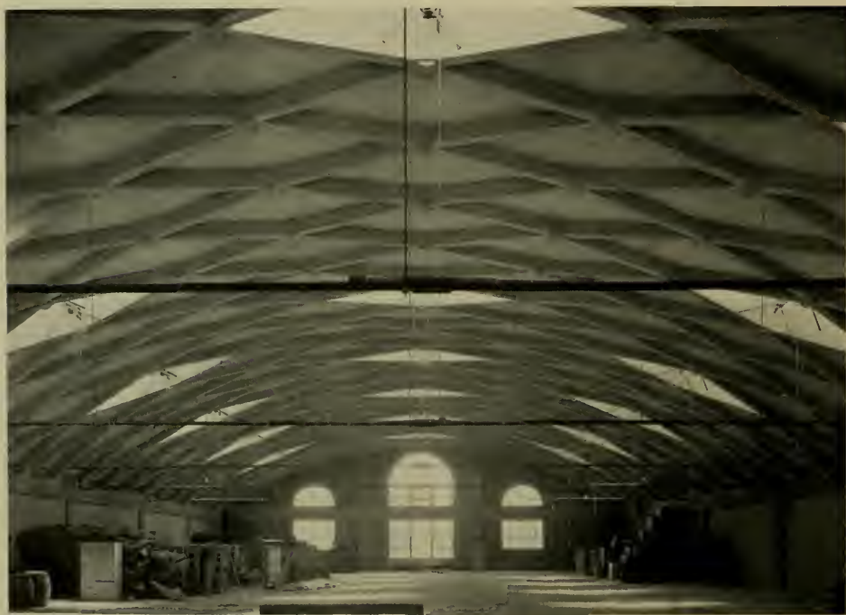
GENERAL VIEW OF INTERIOR, COCO COLA PLANT, LOS ANGELES, SHOWING ROOF CONSTRUCTION IN COMPLETED STATE
