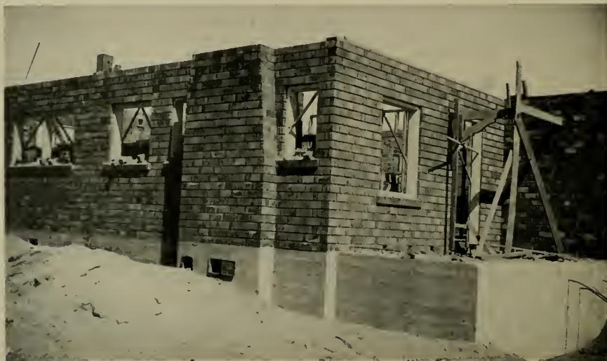
BOULDER CITY, NEVADA Typical residence showing stripped joints in brickwork.
