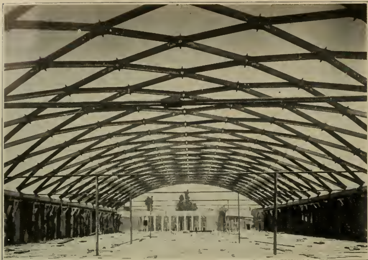
INTERIOR VIEW OF ROOF CONSTRUCTION, SHOWING STEEL TRUSSES BEFORE ENCASED IN CONCRETE
