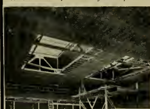
Ribbed STEELTEX Lath for plaster is used for school ceilings, either nailed to wood joists or wire-tied to steel joists or suspended ceilings.
