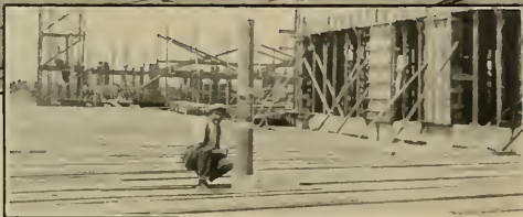
Above: Sisalkraft being used for curing and protecting concrete in the Rigler School, Portland, Ore. Architect, George Jones. Contractor, Ross B. Hammond. Cement Finisher, V. C. McCormick.
