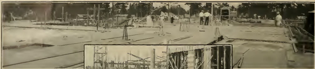
Above: Sisalkraft being used for curing and protecting concrete in the Rigler School, Portland, Ore. Architect, George Jones. Contractor, Ross B. Hammond. Cement Finisher, V. C. McCormick.
