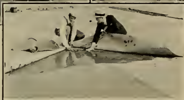
The floors in all the buildings of the University of California at Los Angeles, shown above, were cured and protected with Sisalkraft. The close-up at the right shows the excellent condition of the floor in the Coca Cola plant at Los Angeles after curing under Sisalkraft.
