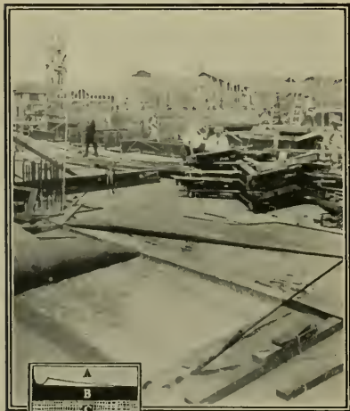
Sisalkraft is composed of crossed layers of sisal fibres imbedded in asphaltum and covered by layers of heavy kraft paper. The construction is exclusive. Made in rolls 3, 4, 5, 6 and 7 feet wide.
