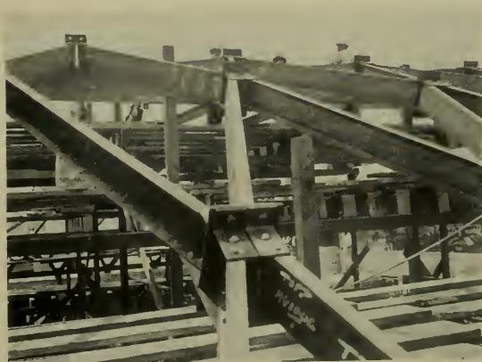
BRACKETS RIVETED TO ENDS OF STEEL CHANNEL LAMELLAS AND BOLTED TOGETHER THROUGH STEEL PLATES
