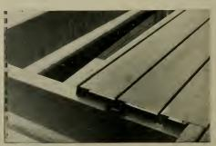
WELDING COMPLETED, ONE END OF UNIT FASTENED TO PURLIN
