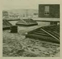
ROOF AREA, SHOWING WIDE MESH BURLAP EMBEDDED IN HEAVY LAYER OF STANDARD PIONEER EMULSIFIED ASPHALT
