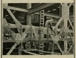
Welded bracing for horizontal stresses-new Southern California Edison Building, Los Angeles
