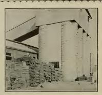
Battery of eight storage bins for crushed slate. Port Orford Cedar was chosen for this job because of its durability, because it shrinks but little.
