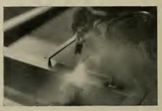
ARC WELDING TO PURLINS, WORKING FROM TOP OF ROOF
