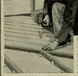
STEP SIX -WOOD FLOOR. After sleepers are securely in place, wood floors are laid. Sleepers and floors are laid without waiting for fill to dry.
