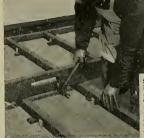
STEP FOUR-LEVnailing, necessary leveling with straight edge is quickly accom-plished. Jaints come within clips and bath ends are nailed.
