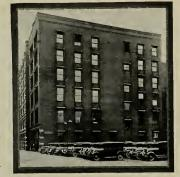
Although Intended primarily for fire protection, the doors and shutters on the first floor are lowered every night to prevent unlawful entrance, and those on the wall ere used, in the summer, instead of ewologs.
