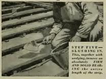
THE Bull Dog Method and process of anchoring wood floors over concrete prevents buckling, squeaking and doming. Once properly wedged and slushed, the sleepers hold the floors rigidly, permanently.
