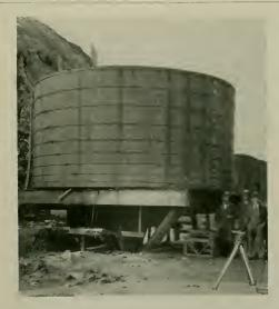
EQUIPMENT USED BY BARRETT AND HILP IN MAKING SOIL. TESTS FOR PROPOSED GOLDEN GATE BRIDGE FROM SAN FRANCISCO то MARIN COUNTY
