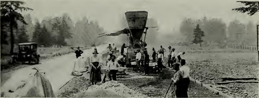
WIDENING CONCRETE HIGHWAY TO CAMP LEWIS, PIERCE COUNTY, WASHINGTON—MISS MORGAN IN FOREGROUND—COUNTY ENGINEER WHITE BLOCKING TRAFFIC ON PAVED HIGHWAY.
