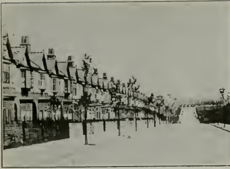
Typical overpaved street and modern narrow roadway of the new type for minor residence streets. Great saving in paving costs can be made when the residence zones are definitely established and major and minor streets determined upon.
