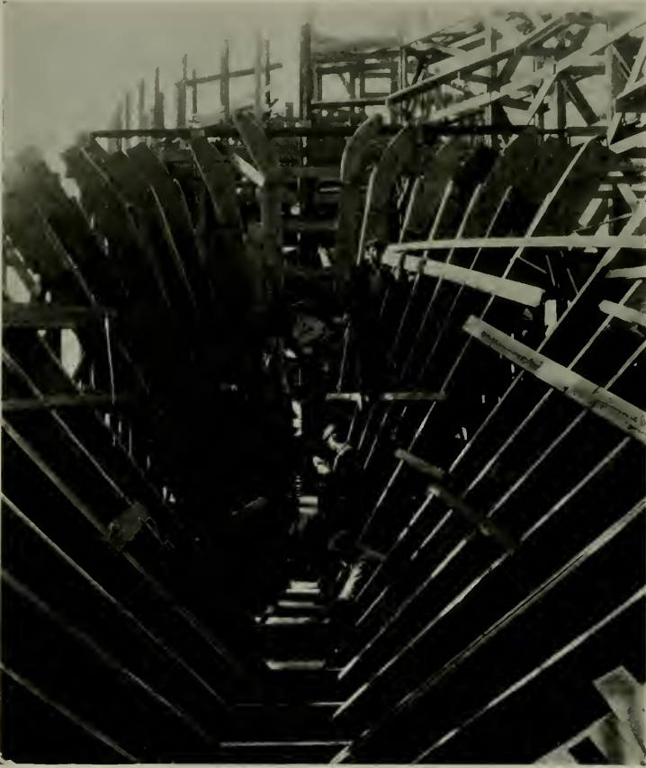
LOOKING AFT IN 7500-TON CONCRETE OIL TANKER, SHOWING STERN FRAME IN PLACE
