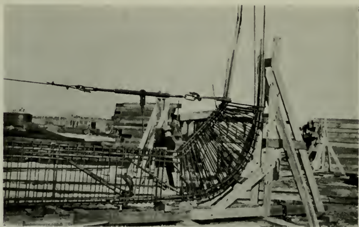
FIG. 4—Bottom frame steel of the Atlantis, built up as a unit on the ground and by means of a cable and ratchet pulled together at top to facilitate placing frame inside the shell steel previously erected.
