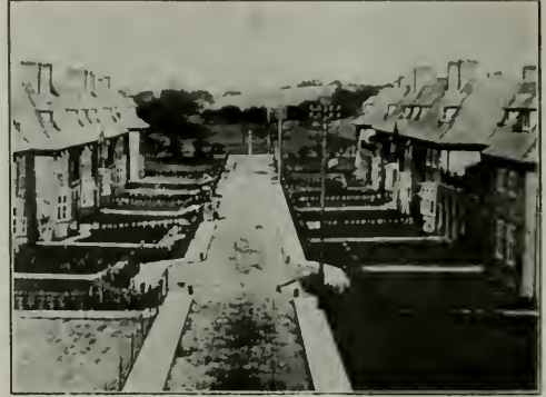
Typical overpaved street and modern narrow roadway of the new type for minor residence streets. Great saving in paving costs can be made when the residence zones are definitely established and major and minor streets determined upon.
