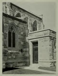
VIEW SHOWING EFFECT OF CONCRETE TRIM STONE IN FIELD OF NATURAL SANDSTONE
