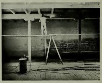
BUILDING FOR ENTERPRISE ELECTRIC COMPANY, SHOWING APPLICATION OF PABCOAT, THE STONE VENEER, TO INTERIOR WALLS
