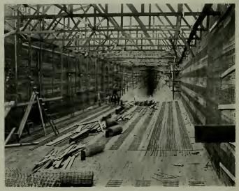
THE FAITH UNDER CONSTRUCTION, SHOWING METHOD OF STEEL REINFORCEMENT
