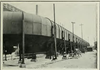
Balloon Flue of The St. Joseph Lead Company, Herculaneam, Mo. Total installation more than one-fourth of a mile long and eight feet in diameter. ARMCO (American Ingol) from used exclusively.
