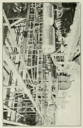
Interier of one of the largest musting factories in the country, showing the London overhead energy-not system in operation. All finings and horings from each machine are carried to a central storage, thus saving every exerp, an economy which will in a short time pay for entire installation. (alifornia laylatadic and bagineering simply Co., San Francisco, agents.
