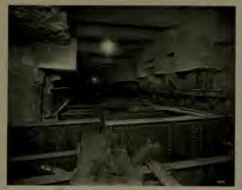
LATTICE GIRDERS INSTALLED ON SUBWAY ROOF BEAMS TO DISTRIBUTE FOUNDATION LOADS
