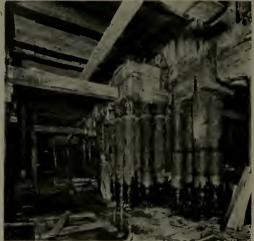
PERMANENT UNDERPINNING PILES BETWEEN SUBWAY TRACKS. TEMPORARY PILE CLUSTERS MARKED 25 TO BE REMOVED
