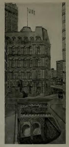
SYSTEM OF GIRDERS ON SECTIONAL PILES SUPPORTING POST OFFICE AND FIRST SUBWAY DURING CONSTRUCTION OF SECOND SUBWAY IN QUICKSAND UNDERNEATH POST OFFICE BUILDING, NEW YORK CITY
