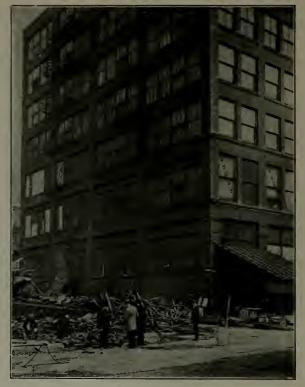
A SUCCESSFUL FIRE STOP Showing satisfactory fire retardent service of metal window frames and wire glass. Warehouse opposite side twenty-foot alley was totally destroyed. Windows at rear were broken when side wall of burning building fell.
