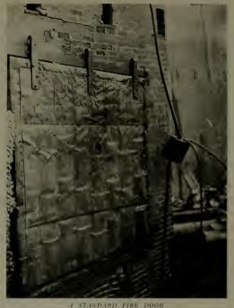
In a large paper trarelionse, where everything in one section teas destroyed by fire, a line of standard timelad fire doors effectively protected all stories of the adjoining section. The accompanying pho-tograph shows one of these doors.
