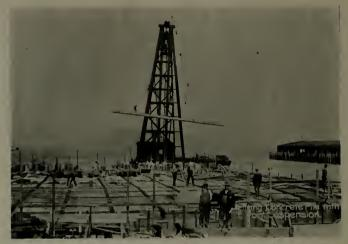
LIFTING CONCRETE FILE WITH FIVE-POINT SUSPENSION, FIER 3, SAN FRANCISCO WATER FRONT
