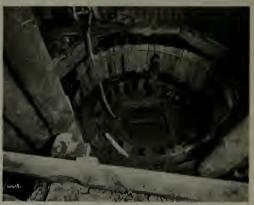
SUMP PIT ENCAVATED AND SHEET PILED WITH CONCRETE WALL FORM PARTLY ASSEMBLED
