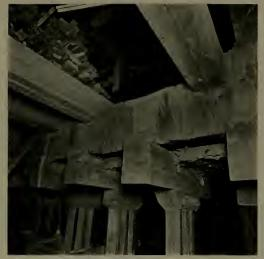
CONCRETED GIRDERS SUPPORTING OLD FOUNDATION. CON-CRETED COLUMNS UNDER THEM BEARING ON SECTIONAL PILES
