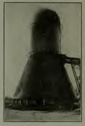
Refuse Rurner of Rine Annealed Armon Iron, built by the Walsh Construction Co. of Vancouver, R. U., for Runting & Merritt Launher Company,
