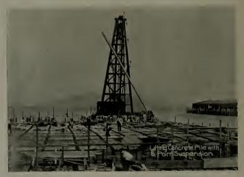
LIFTING CONCRETE PILE WITH FIVE-POINT SUSPENSION, PIER 3, SAN FRANCISCO WATER FRONT J. D. Hummah, Contractor
