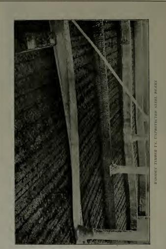
The fire in this mill did not affect the stability of the wooden timber, olthough the ten-inch steel beams sogged and were twisted to a degree which required rebuilding. The wooden beam was used in the frame because not enough steel had been ordered to complete the work promptly. In rebuilding, wooden beams were used throughout.
