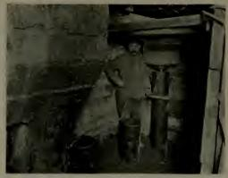
TESTING SECTIONAL PILE WITH HYDRAULIC JACK /
