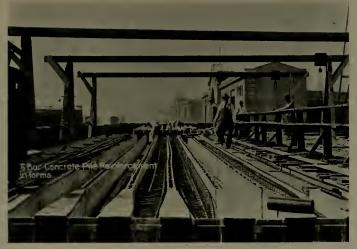
CONCRETE PILE REINFORCEMENT IN FORMS, PIER 31 SAN FRANCISCO WATER FRONT
