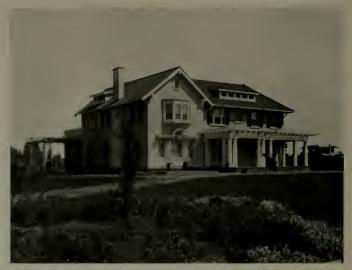
HOUSE FOR MR. A. G. WISHON, FRESNO. EXTERIOR OF ASBESTOS STUCCO Coates & Traver, Architects
