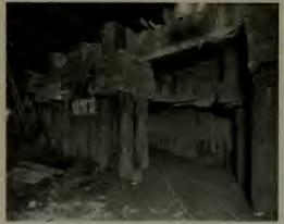
UNDERVISING PILES SUPPORTING CONCRETED GIRDERS UTTU SUBILAY ROOF REAMS ON TOP
