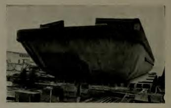
REINFORCED CONCRETE BARGE
