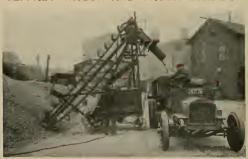
Type A-16 Loader, motor driven, loading a truck in three to four minutes. The self-propelling device enables one man to handle the loader. He can move it into the pile or from pile to pile under its own power.
