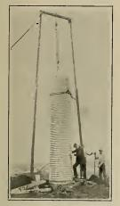
Showing a simple but efficient derrick for handling curbing.
