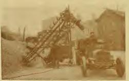
Type A-16 Loader, motor driven, loading a truck in three to four minutes. The self-propelling device enables one man to handle the loader. He can move it into the pile or from pile to pile under ite own power.
