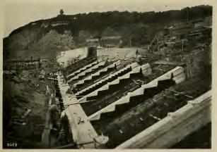
SECTION B OF ESPLANADE. H-BEAM GIRDERS AND REINFORCEMENT FOR BLEACHER SLABS IN PLACE
