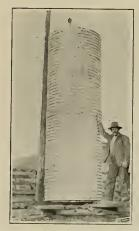
"Armeo" Iron Galvanized, Corrugated Well Curbing of 42" diameter being installed on ranch of Geo, C. Russell near Enterprise, Oregon,
