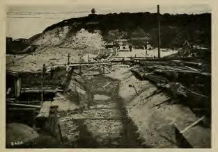
BUILDING SECTION B PREPARATORY TO PLACING H-BEAM GIRDERS. SHEET PILING IN PLACE
