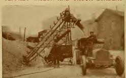
Type A-16 Loader, motor driven, loading a truck in three to four minutes. The self-propelling device enables one man to handle the loader. He can move it into the pile or from pile to pile under its own power.
