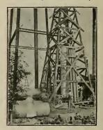
Corrugated Well Curbing being placed in municipal well at Clovis, N. M. The installation of 29 feet of 30" diameter was accomplished in tweke hours. Material was No. 14 gauge galvaniced "Armoo" Iron.
