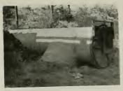
Fig. 4—48 inch Automatic Drainage Gate, attached to 300 fect of corrugated pipe, installed on Reclamation District No. 1000, about twenty miles north of Sacramento, California.
