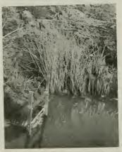
Fig. 6—Automatic Gate closed against high water, 36-inch Automatic Drainage Gate installed on Russ Island, five miles west of l'allep, Calorinia. This picture was taken about ten minutes after the turn of the tide and shows the gate closed. This gate was installed by means of a dredger at approximately one-half the estimated cost of a wooden gate of equal capacity.
