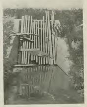
Fig. 7—Wooden grating for catching debris. Automatic Drainage Gate, Ralph Bull ranch, near Arcata, California, on Humboldt Bay.
