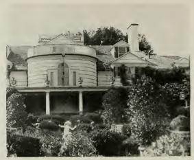
Fig. 1. Doy view of the residence of J. L. Breese, showing the arrangement of the projector units on the roof of the porch for lighting this garden, and also in the foreground the two box lights for lighting the fountain
