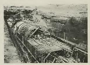
SECTION CONSTRUCTED IN OPEN CUT AT WEST END, TWIN PEAKS TUNNEL, SAN FRANCISCO.
