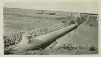
Fig. 9—Showing 24-inch riser pipe 2 feet high, with balted top, which is used to clean culvert after flood season.
