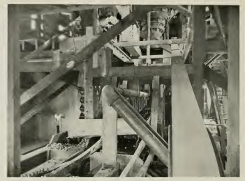
INTERIOR OF PLANT, SHOWING CRUSHER, SHAKING SCREEV AND WATER SUPPLY PIPE
