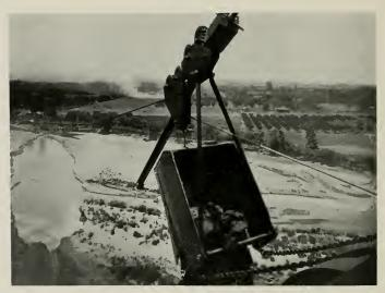
BUCKET CONVEYING RAW MATERIAL FROM GRAVEL PIT TO PLANT
