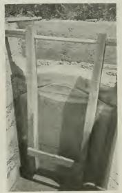
Fig. 1—Automatic Drainage Gate, Ralph Bull ranch, near Arcata, California, an Humbaldt Bay. Concrete conduit and wooden cover. Arca of conduit approximately 16 square feet. Approximate thickness of concrete 6 inches. The wood gate is not sufficiently sensitive to water level changes.
