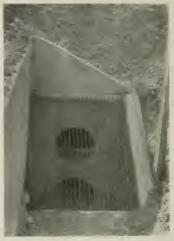
Fig. 8—Intake end standard drain for water pocket. The lower pipe has Automatic Drainage Gate on opposite end, and runs through levee into candi. The upper pipe is an inverted stylion used to represent the standard of the properties of the gate. Water thus entering the District is permitted to drain naturally to the river leves, where it is caught in sumps and pumped into the river.
