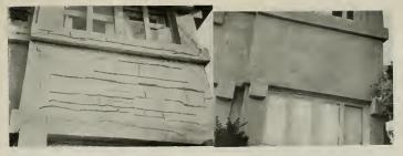
Fig. 5 Section of coment-plastered residence. Note defects due to absorption of water.
