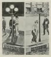
bedded in the vertical sides of the curbs. These consist of waterproof cast-iron boxes, 40 inches long and 8 inches deen, perforated with the street names and illuminated by means of tubular electric lamps which are connected with the city lighting system. Two of these signs are installed at each of the four corners at the intersection.
