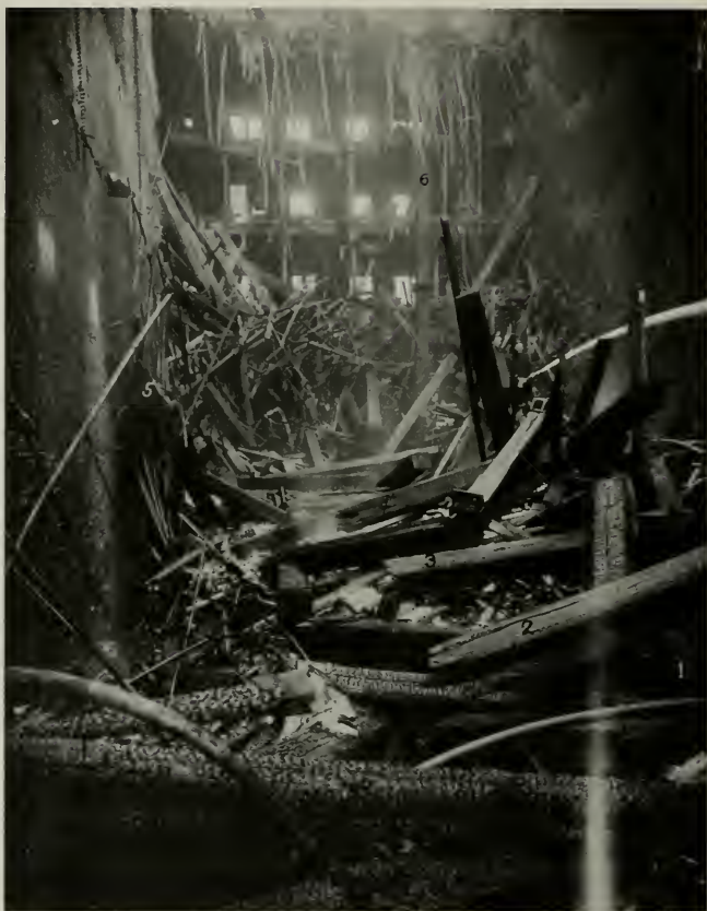
Dry Rot in Timbers. —Shortly after the fire was under control the floors began to fall in irregular sections, and in two or three hours the whole floor system of the large building had fallen in a tangled mass to the basement. The reason of this collapse is indicated by the condition shown in timbers numbered 1 to 6.
