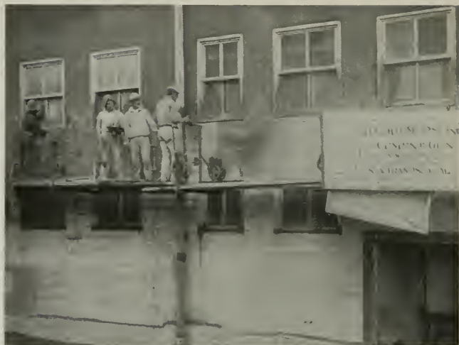
REAR WALL OF HALE DEPARTMENT STORE, SAN FRANCISCO, being waterproofed with the aid of the Cement Gun. Part of the west wall of this building was similarly treated several years ago and it was the only dry spot during the recent heavy rains.
