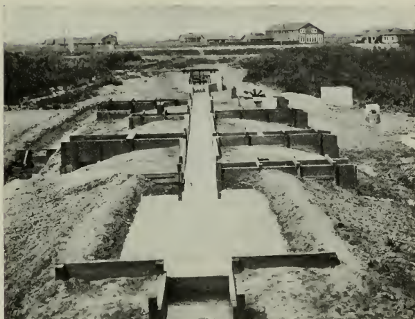
WATER MEASURING DEVICES, UNIVERSITY STATE FARM DAVIS (Used in experiments to determine the duty of water)
